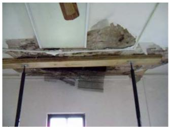
2<sup>nd</sup> floor office, damaged plaster ceiling
