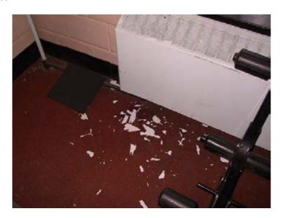
Room 1, first floor, south wall and front window. Deteriorated paint was sampled for lead.
