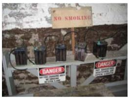
Photo 14: An old battery charging area that is located in the electrical room.
