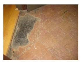
Photo 7: Damaged 9 inch x 9 inch brown floor tile with black and white flecks located in Room 9 (Cammo Room).
