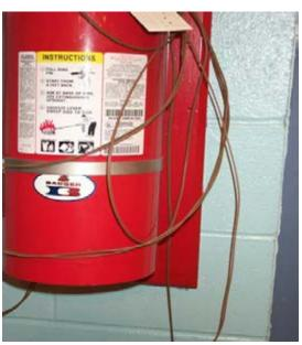
Fire extinguisher wrapped with wires
