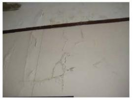
Photo 5: Evidence of water damage on the wall of Room 21 (First Photo 6: Evidence of water damage Room 8 (Supply Office). Sergeant's Office).
