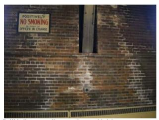
Drill hall, west wall, water-damaged bricks
