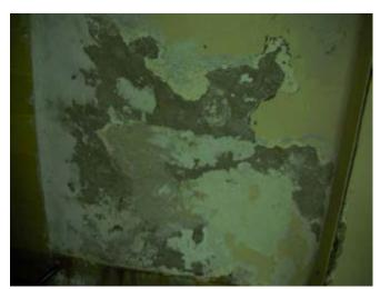
Basement restroom, damaged plaster
