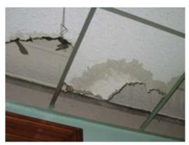
Photo 7: Water stained suspended ceiling tile in the first floor bathroom
