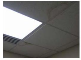
Photo 6: Water stained ceiling tile located in office 160.
