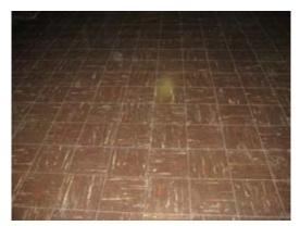
Photo 3: Brown 9 in x 9 inch floor tile with white and red flecks, located in the first floor corridor outside of the main Drill Hall.
