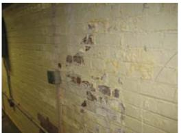
Photo 9: Evidence of water incursion in the Old Firing Range that now functions as a Ventilation Room.
