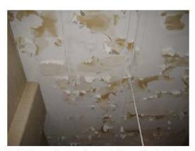
Photo 7: Evidence of water damage to the ceiling in Hallway 3-7a.
