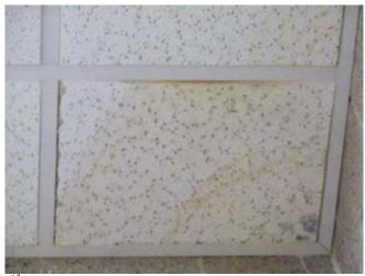
2<sup>nd</sup> floor stairwell, stained/moldy dropped-ceiling tile
