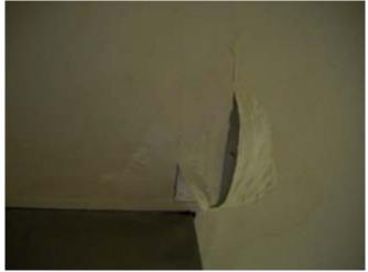
Room 22, dishwashing room, water-damaged drywall ceiling
