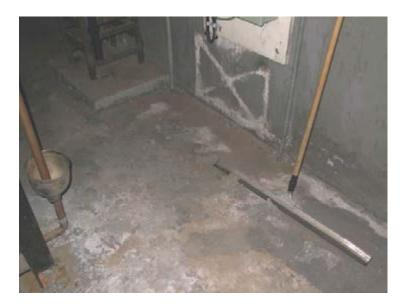
Floor of Boiler Room. Floor surface flaking due to water damage and age.
