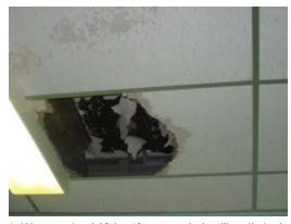
Photo 6: Water stained 2ft by 4ft suspended ceiling tile in the first floor bathroom.
