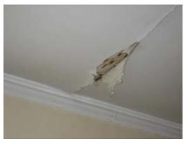
Photo 8: A water damaged ceiling located in Room 201.
