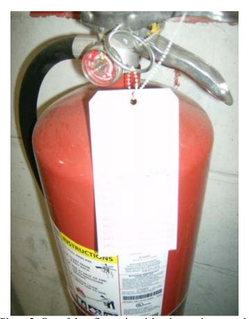
Photo 2: Out of date fire extinguisher inspection record.
