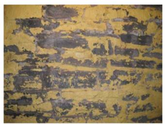
Basement, room 3, water-damaged wall and peeling paints
