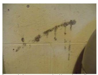
Basement locker room, suspected mold growth on wall
