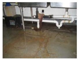
Photo 8: Water accumulation on the floor of the kitchen is reportedly from a back-up in the sump pump.
