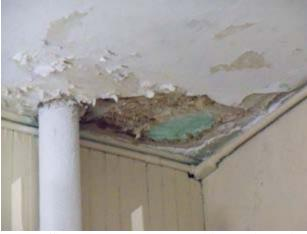
Supply office 122, damaged plaster ceiling/peeling white paint
