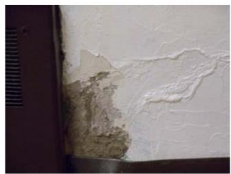
Room 107, peeling white paint and water-damaged plaster wall
