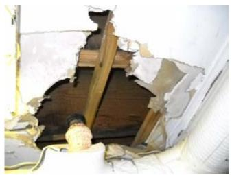
Room B7, damaged drywall ceiling
