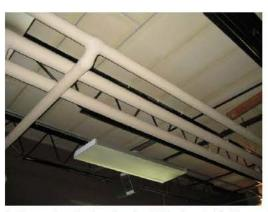
Photo 8: Suspect asbestos pipe insulation located in Room 17 (Club Room).
