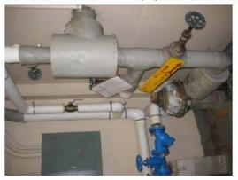
Photo 9: Suspect asbestos pipe insulation located in the Boiler Room.
