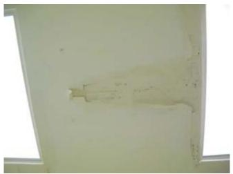
Room 58, restroom, water-damaged ceiling
