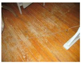
Photo 17: Communication cable across a walkway presents a trip hazard in the Commanders off.
