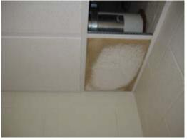
Photo 5: Water stained ceiling tile located in the administration office.
