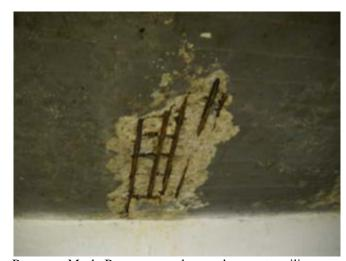
Basement Mech. Room, water-damaged concrete ceiling
