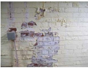
Mechanical room 232, peeling yellow paint / water-damaged brick wall
