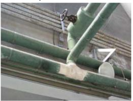
Photo 3: Suspect asbestos-containing pipe insulation located in Photo 4: Water stained ceiling tile located in the mess hall. the Atrium area.
