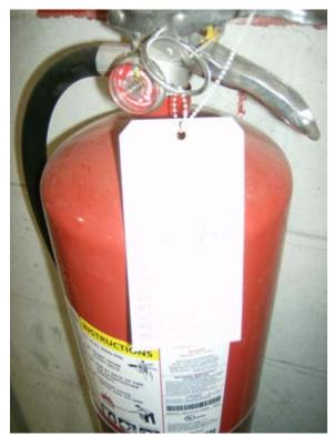
Photo 1: Out of date fire extinguisher inspection record.
