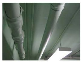
Photo 12: Green suspect asbestos pipe fittings located in the Basement Classroom.
