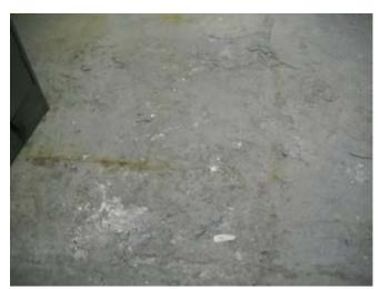
Room B5, water-damaged concrete floor
