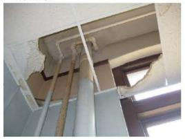
Photo 10: Evidence of water damaged ceiling tiles in Room 2-2 (Office).
