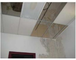
Photo 8: Evidence of water damage to the ceiling and walls in Room 3-10f (Office).
