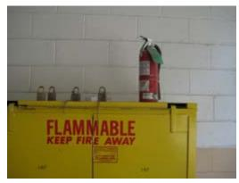
Photo 12: A fire extinguisher is not properly mounted to the wall in the Atrium area.
