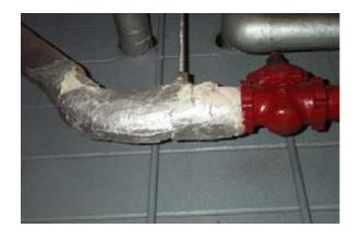
Asbestos containing insulation
