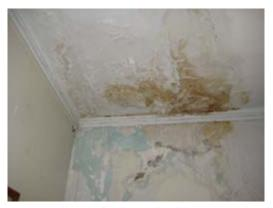
Photo 7: A water damaged ceiling and wall located in Office 219.
