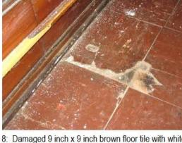
Photo 8: Damaged 9 inch x 9 inch brown floor tile with white and black flecks in Room 21 First Sergeant's Office.
