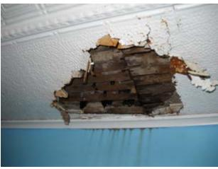
Room 305, water-damaged metal ceiling
