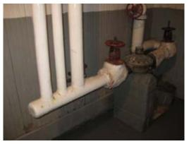
Photo 5: Suspected asbestos-containing pipe insulation on approximately 6 inch pipe in the basement change room.
