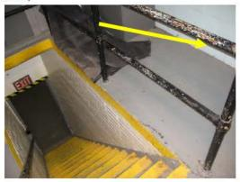
Photo 10: A hand railing is loose and unstable, presenting a fall hazard in the second floor Locker Room.
