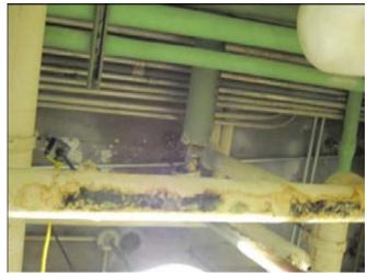
Room 75, Boiler room, fungal growth on FG pipe insulation
