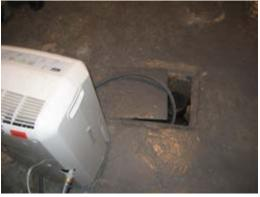
Photo 16: A partially removed drain cover presents a trip hazard in the basement kitchen area.
