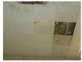
Photo 6: Water damaged ceiling tile located in the Firing Range.
