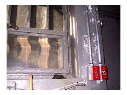
Boiler Room. Paint peeling due to age and high humidity.
