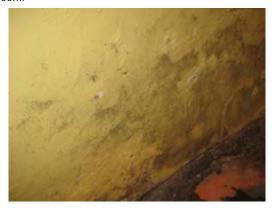
Photo 9: Suspect mold is located on a plaster wall in the basement storage area.
