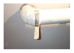
Locker Room (former IFR) – deteriorating pipe insulation
