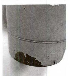
Photo 18: Classroom fire extinguisher showing signs of rust damage.
