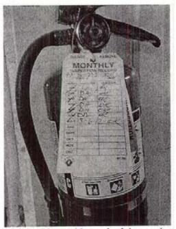
Photo 24: Fire extinguisher with expired inspection tag located in Basement.
