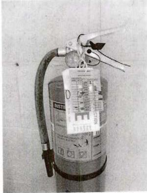
Photo 2: Fire extinguisher past due for monthly inspection and annual servicing.
