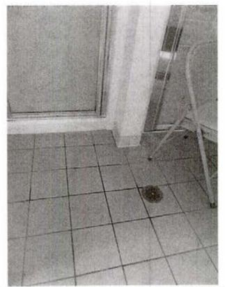
Photo 3: Floor drain in Men's Restroom releasing gas odor.
