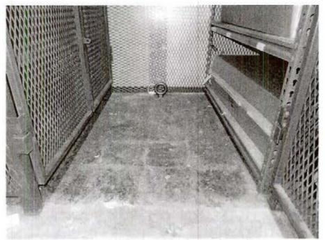
Photo 19: Mastic residue in supply vault.
