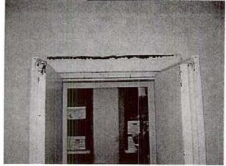
Photograph 13 Peeling paint located on storage room vault door
