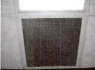
Photograph 7 Indoor Air Quality – Typical soiled return air grille
