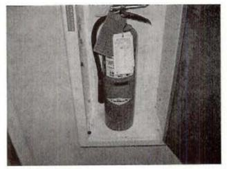
Photograph 9 Safety – Fire extinguisher without current monthly inspections
