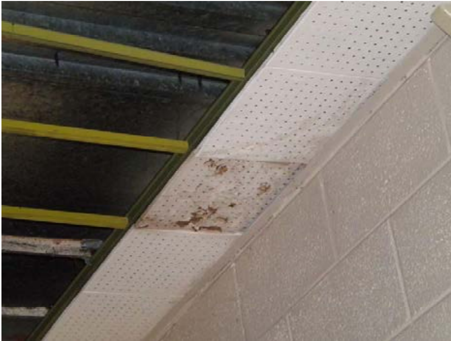
Damaged ceiling tile room 200
