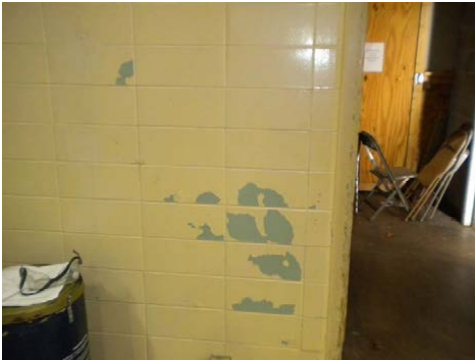
Peeling paint in drill floor area
