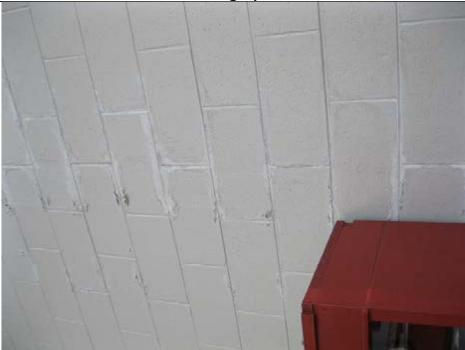
Flaking paint in drill hall
