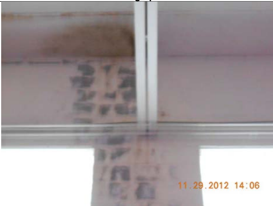
Peeling paint/water intrusion/gymnasium
