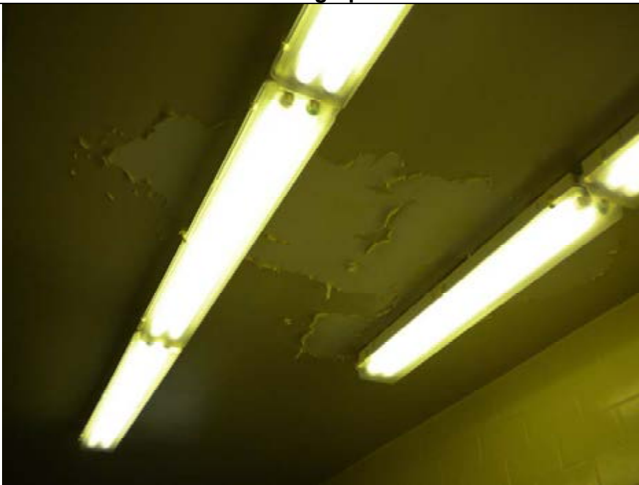
Peeling paint in scully area
