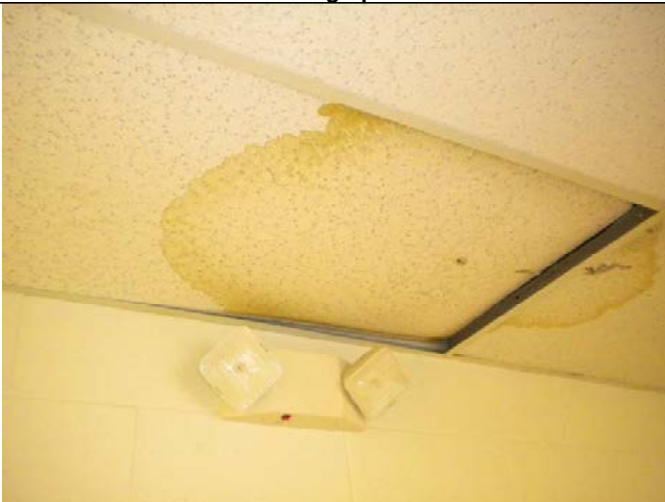
Water damaged tile in conference room
