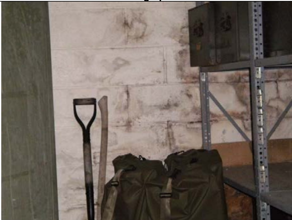
Moisture intrusion SE wall basement storage
