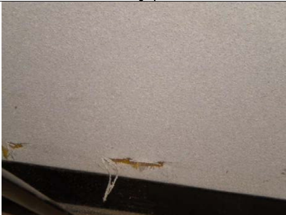
Suspect ACM in former of range
