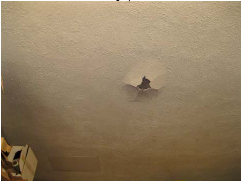
Damaged ceiling plaster
