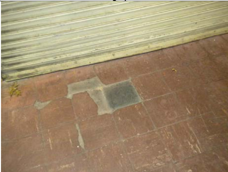
Damaged 9X9 tile in drill hall
