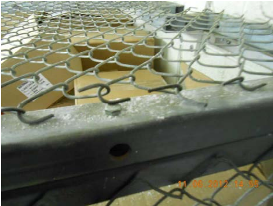
Possible ACM debris-supply room
