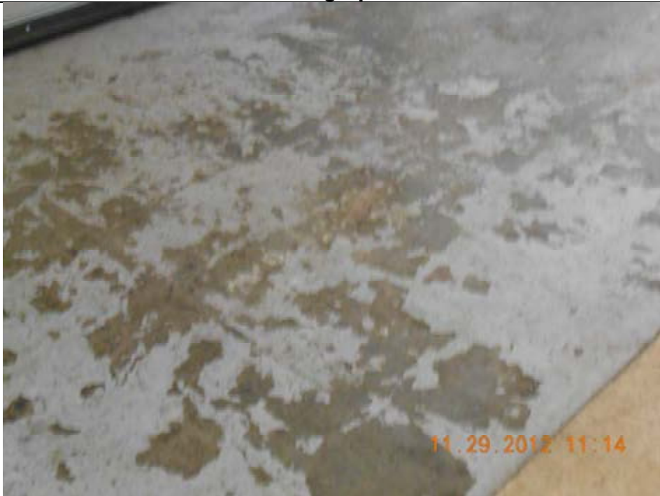
Damaged paint drill hall floor
