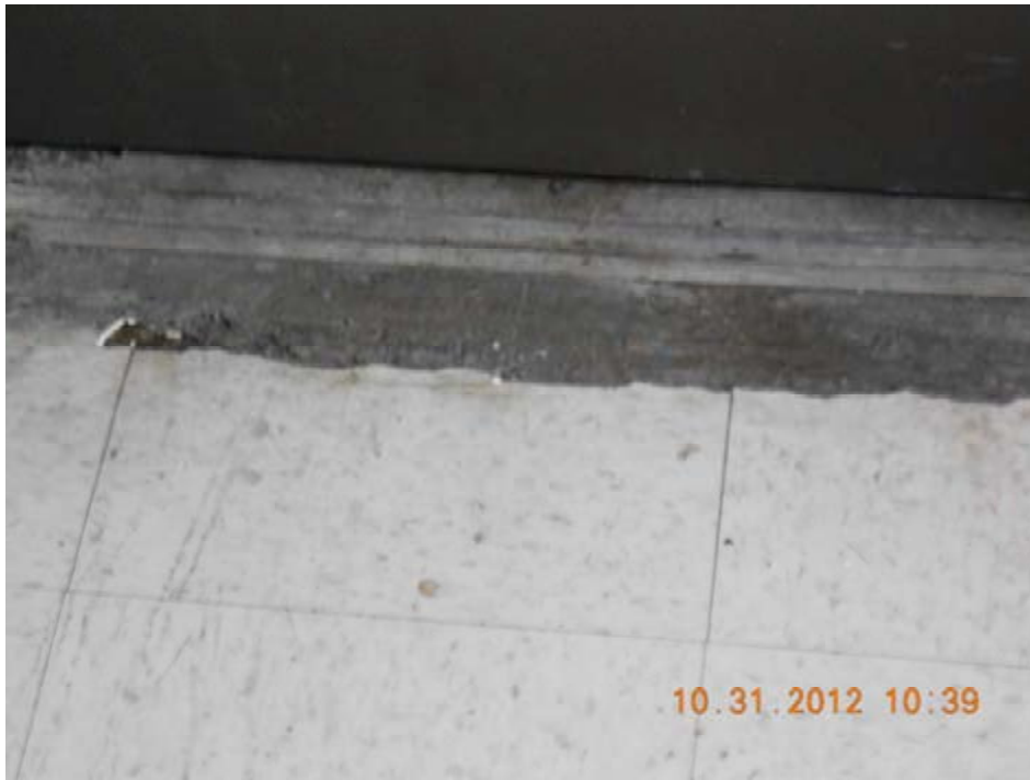
Damaged floor tile
