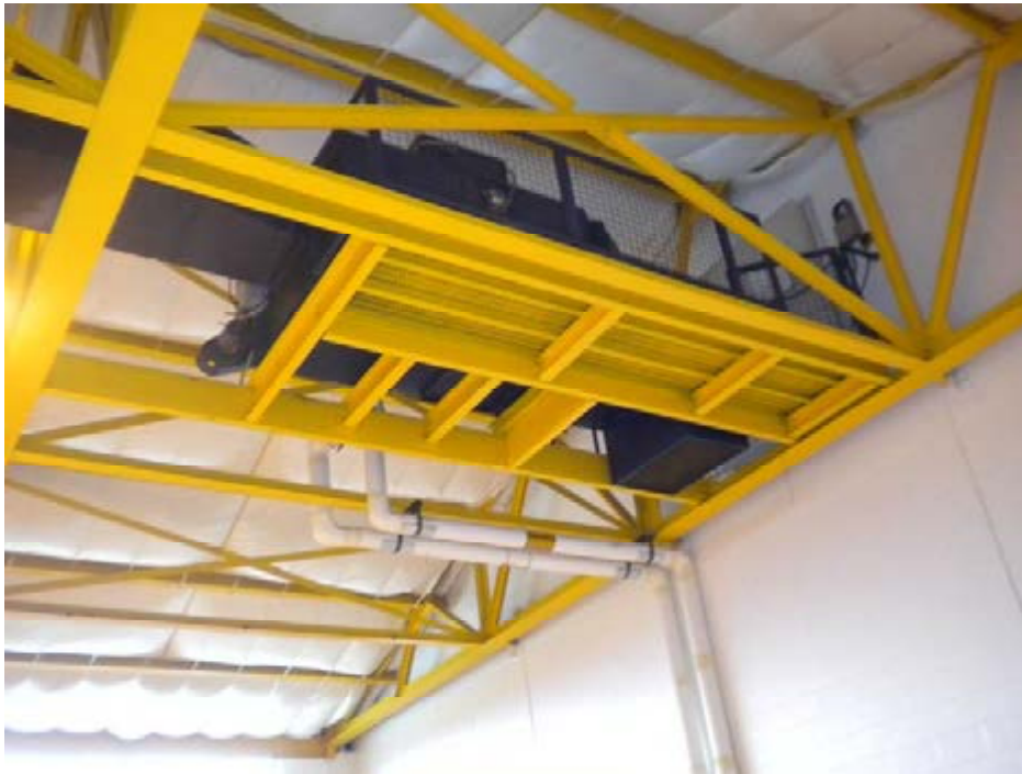
Drill floor air handler
