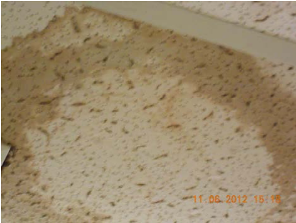
Foyer area water damaged ceiling tile
