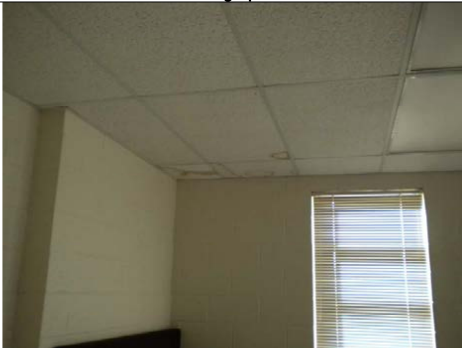
Water damaged ceiling tile classroom 7
