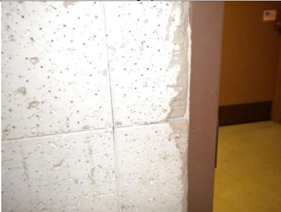
ACM basement acoustic tile on wall of range (AWT-003)
