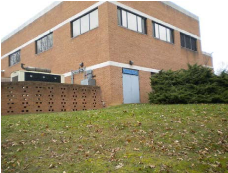
Generator is in close proximity to air intakes
