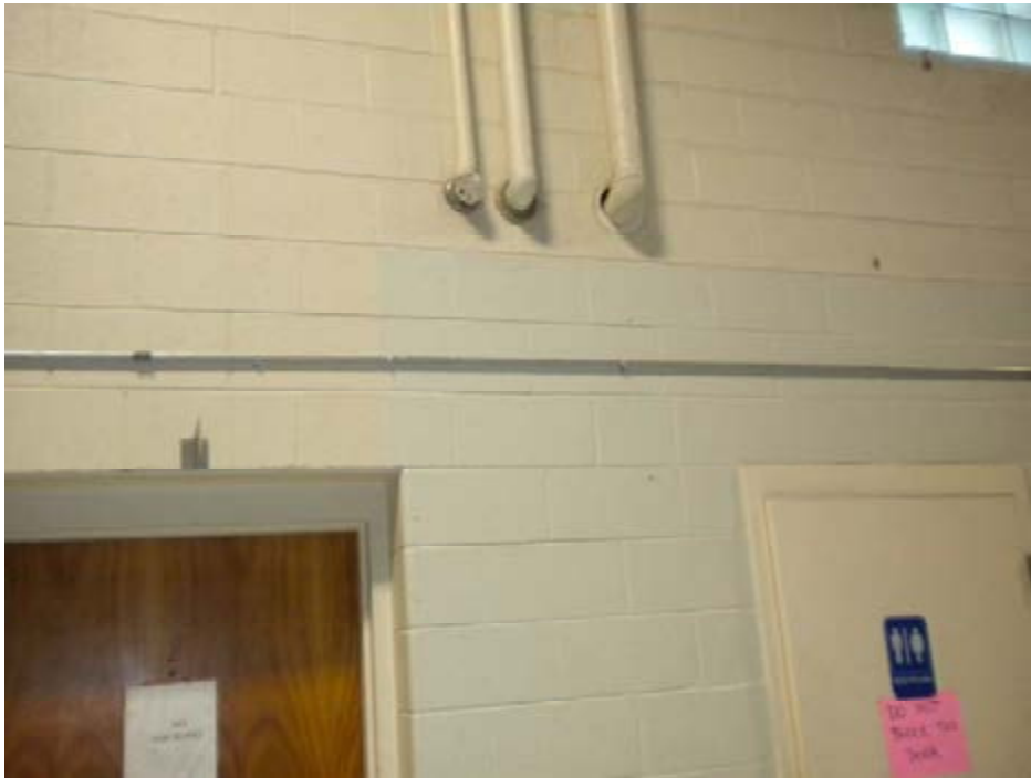
Damaged elbow in drill hall (PIE-002)
