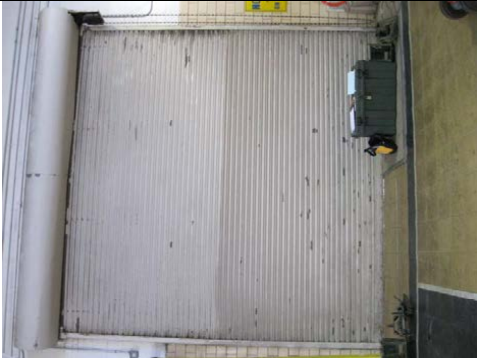
Drill hall roll up door/damaged paint
