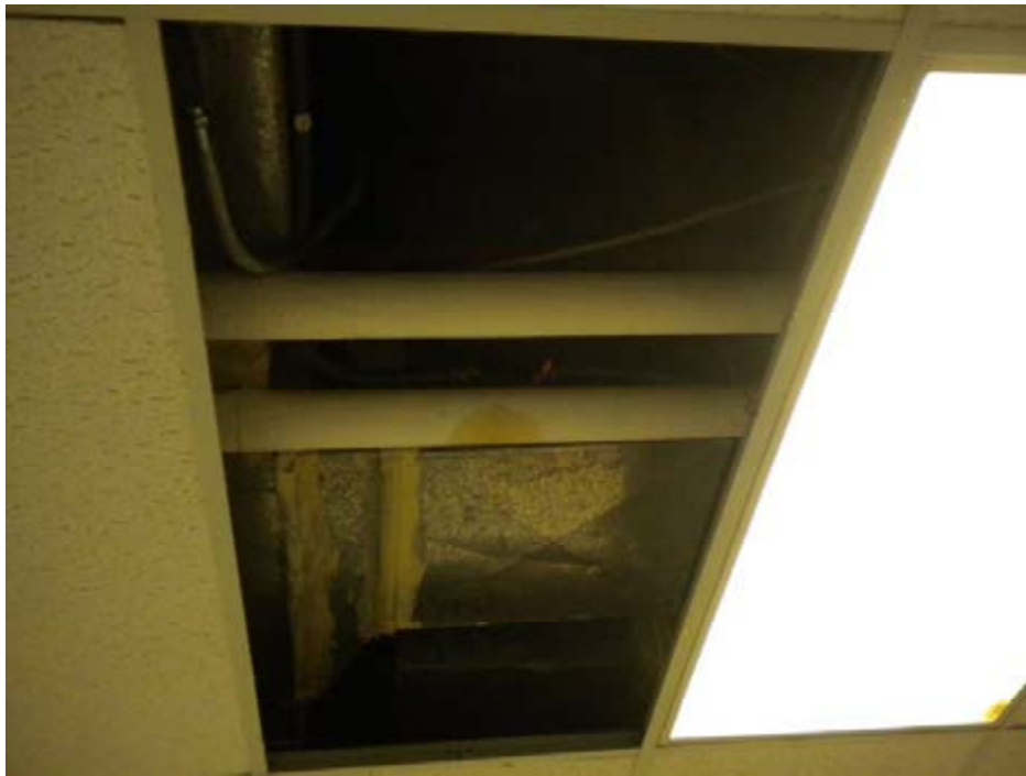
Area of former roof leak room AC-3
