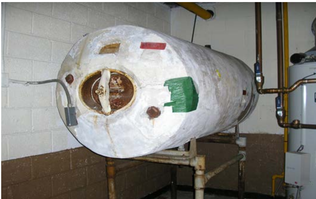
View of Suspect Tank Insulation on Tank in Boiler Room
