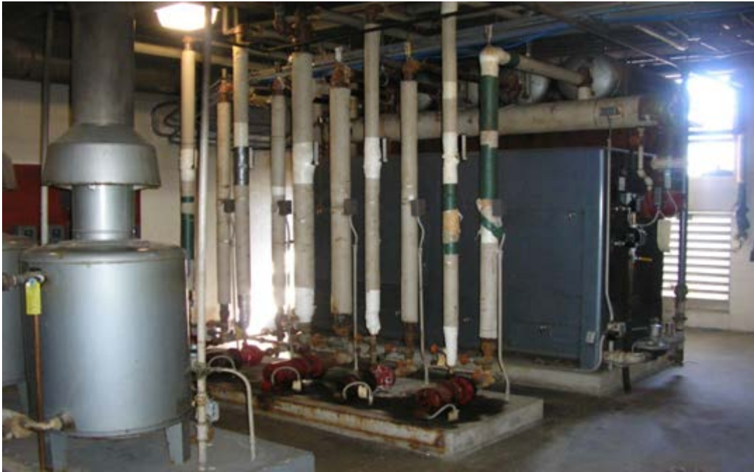
Suspect Pipe Insulation in Mechanical Area/Boiler Room
