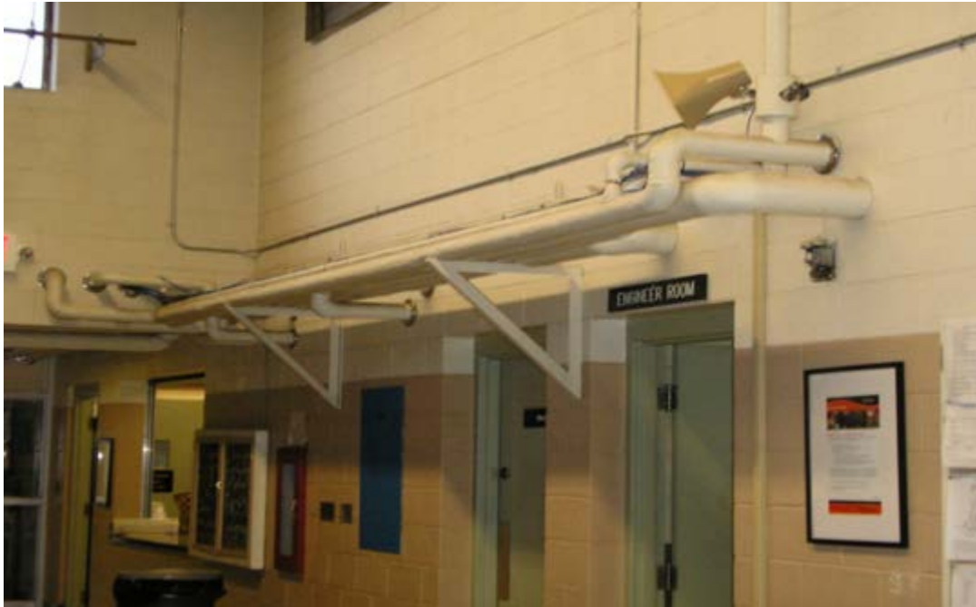
View of Suspect Pipe Insulation in Assembly Hall
