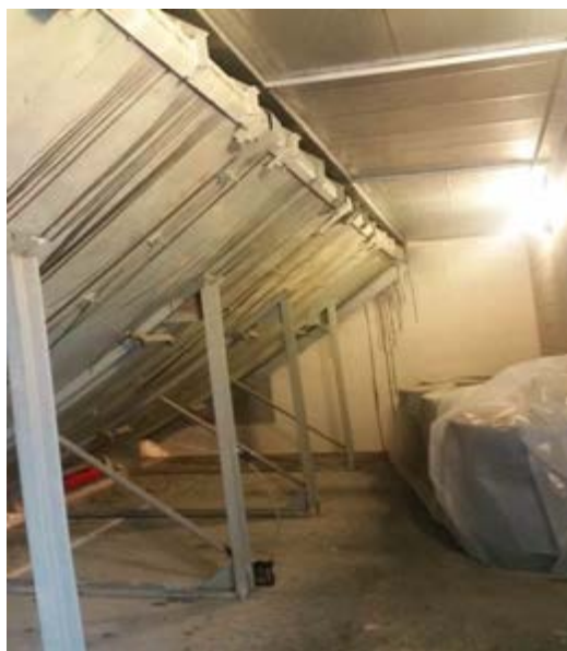
Photo D4. Area behind bullet trap: 1) bullets from bullet trays overflowing on the floor and 2) storing 55 gallon drums
