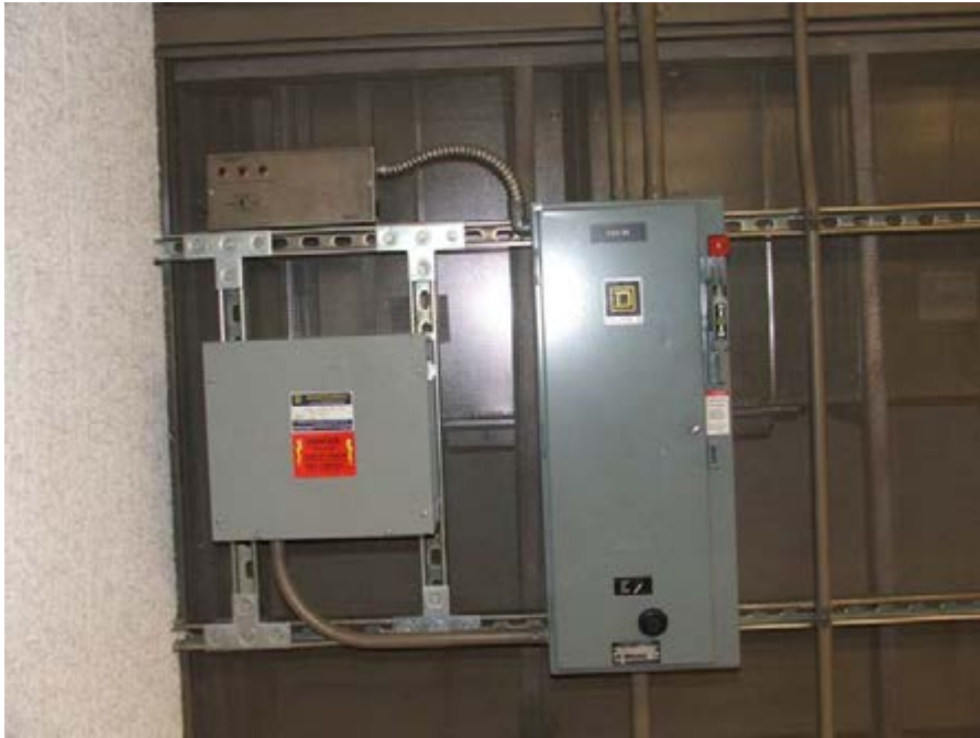
Photograph #3 – Exhaust & Supply Ventilation Control Box Mounted on Supply Plenum
