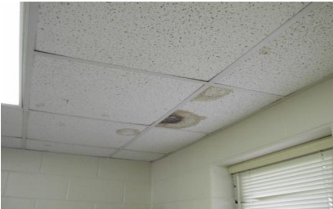
Water damage and suspect mold growth – Front Training Office
