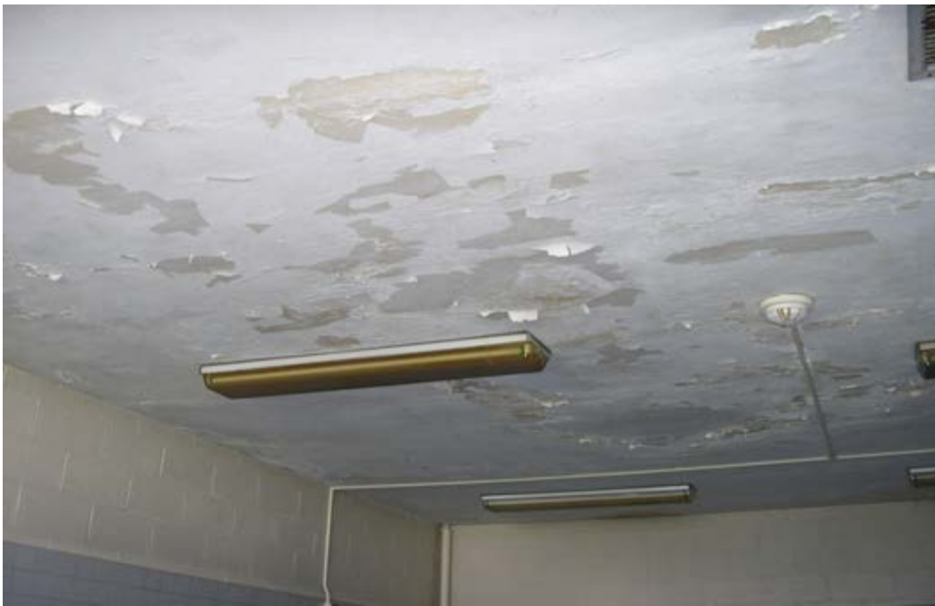
View of Damaged Paint on Female Locker Room Ceiling
