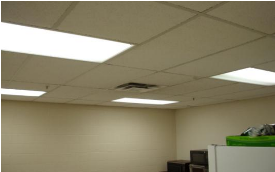
Typical Ceiling Tile and HVAC Supply
