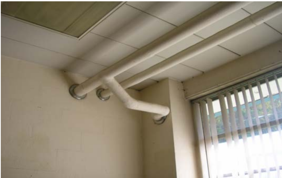
View of Suspect ACM Pipe Insulation
