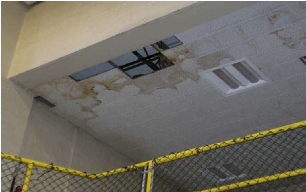
Water Damaged Ceiling Tile in Assembly Hall
