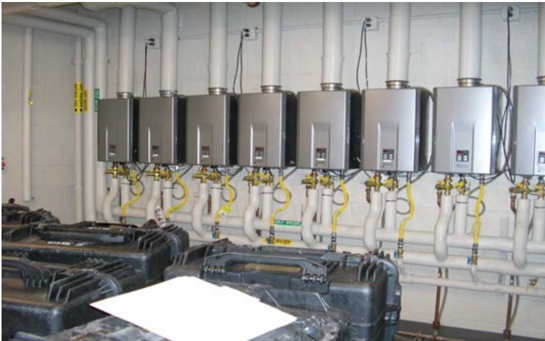
Mechanical Room – Domestic Hot Water On-Demand System
