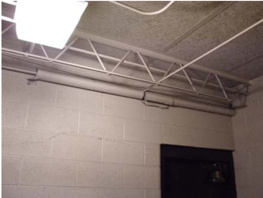
Damaged ACM TSI near Restroom
