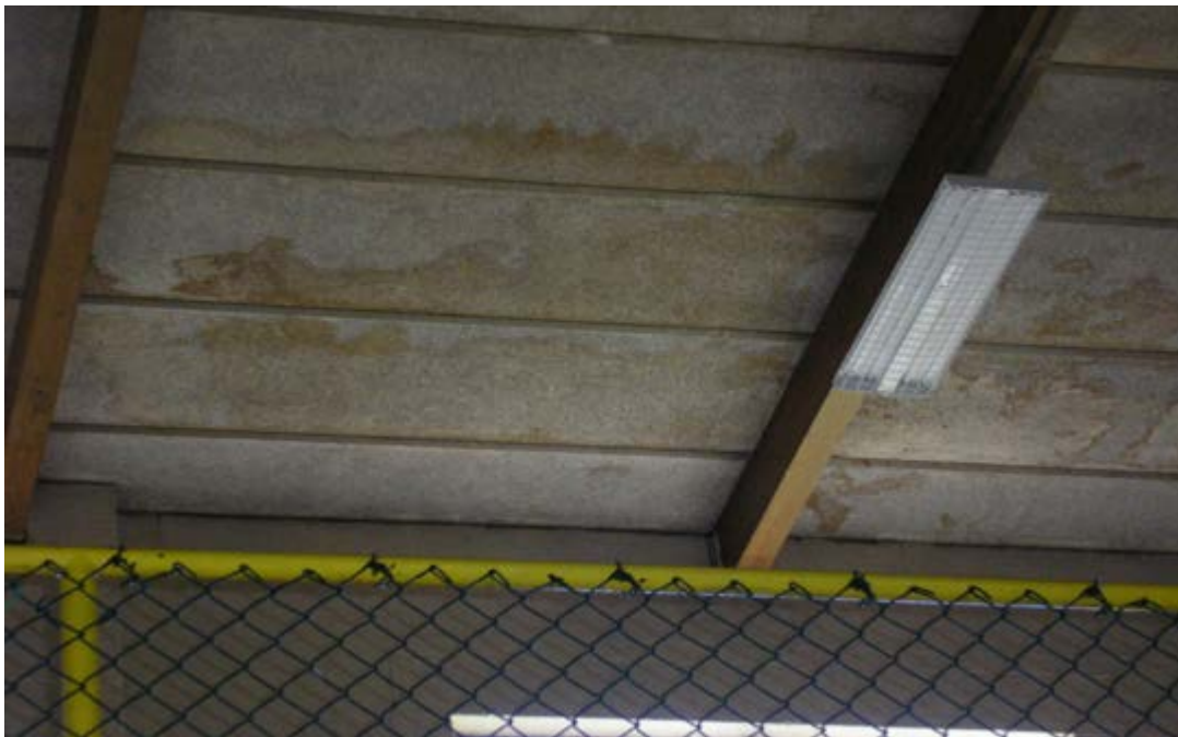
View of Water Infiltration Through Ceiling Deck
