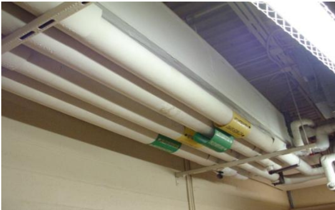
Typical Fiberglass Pipe Insulation
