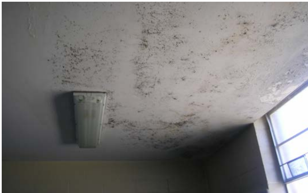
View of Women's Restroom Ceiling Damage and Visible Mold
