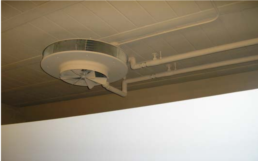
View of Suspect Pipe Insulation in Former Fire Range
