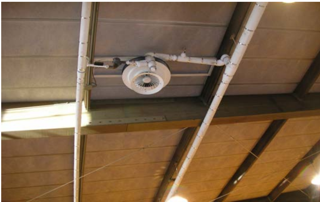
View of Suspect ACM Pipe Insulation in Assembly Hall
