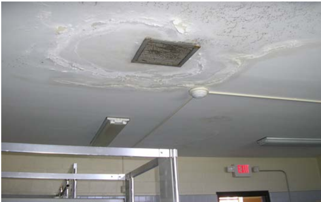
View of Water Damaged Ceiling
