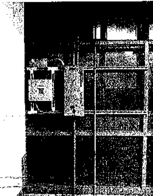
Figure C-4. Control Box blocking Airflow to Lane 5 on the range (insulating panels removed).
