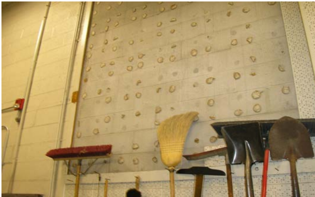
View of Glue Pucks to Missing 1'x1' Wall Tile
