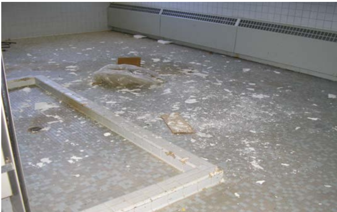
View Ceiling Debris on Female Locker Room Floor
