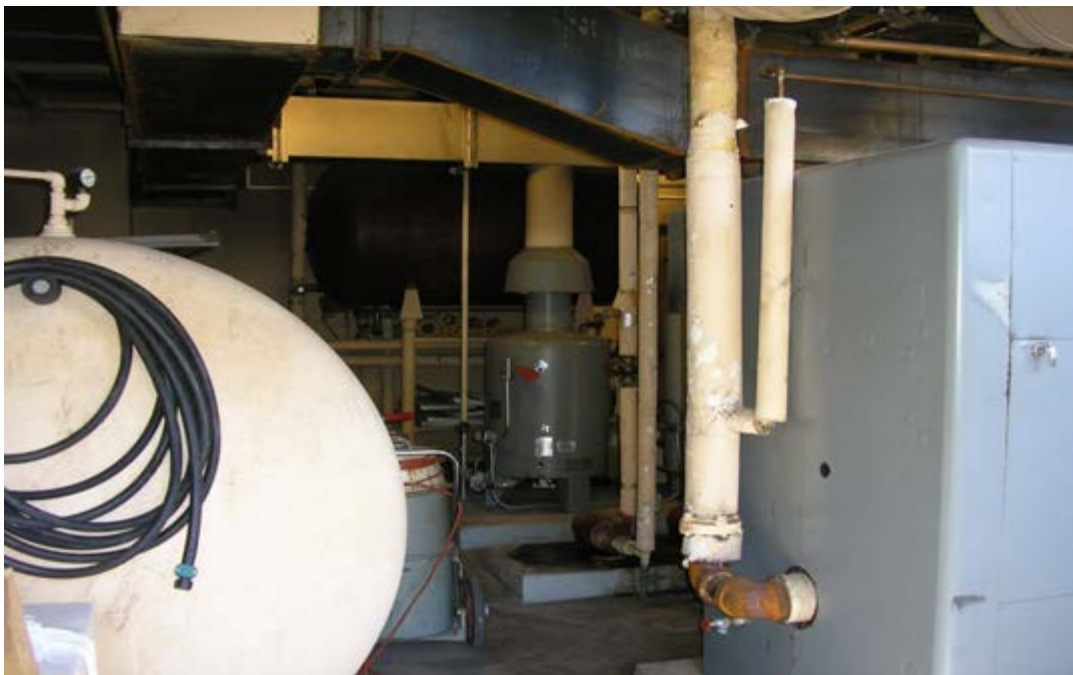
View of Suspect Pipe Insulation in Mechanical Room
