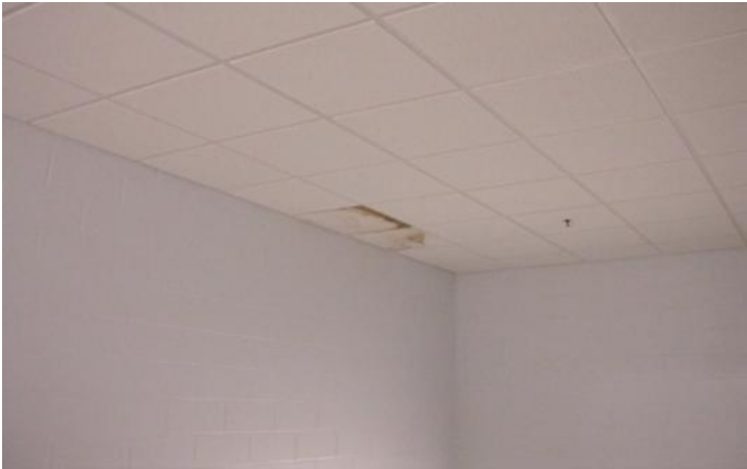
Water damaged ceiling tile in Stairwell
