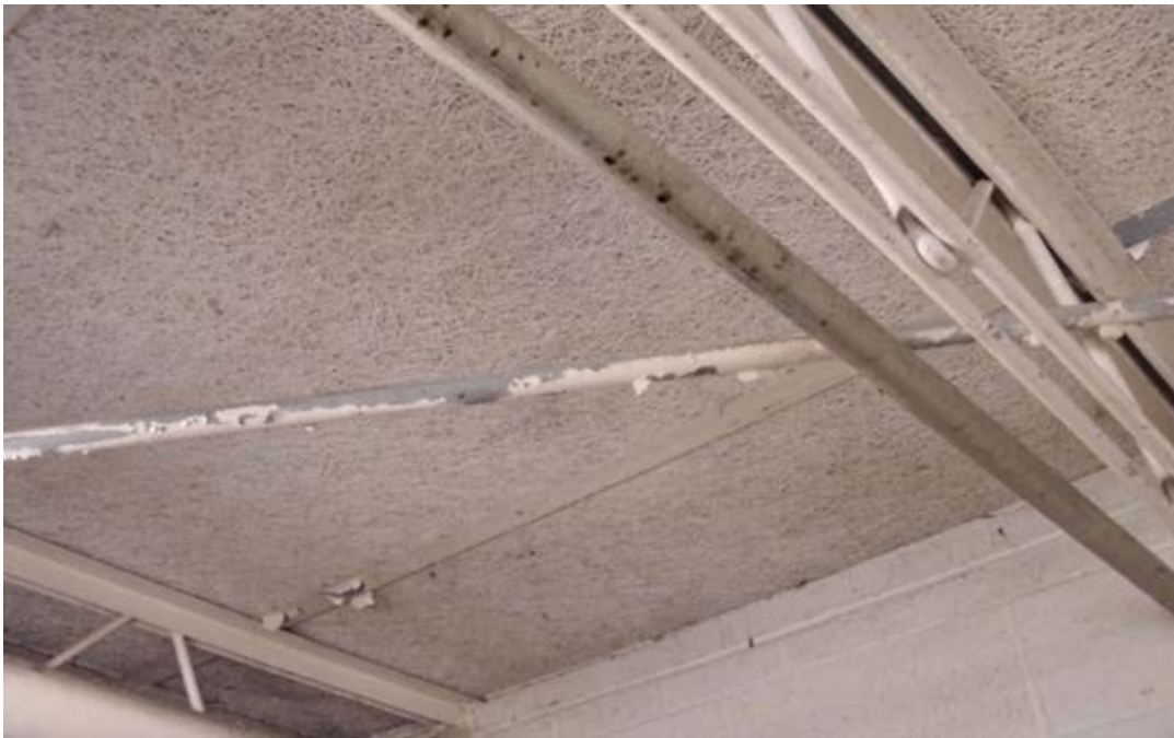
Peeling Paint on Rest Room Conduit
