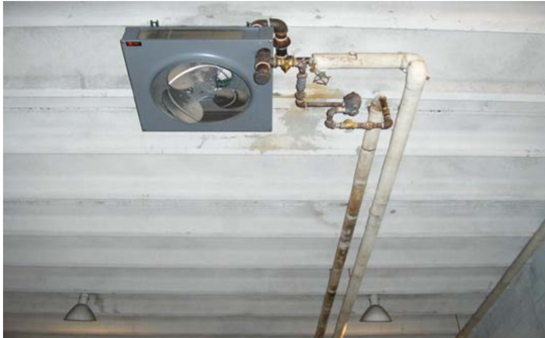
View of Suspect Pipe Insulation in Fire Range
