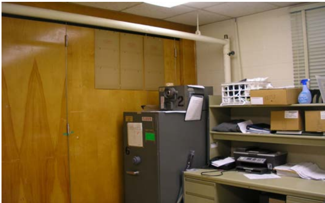
View of Suspect Pipe Insulation in Office
