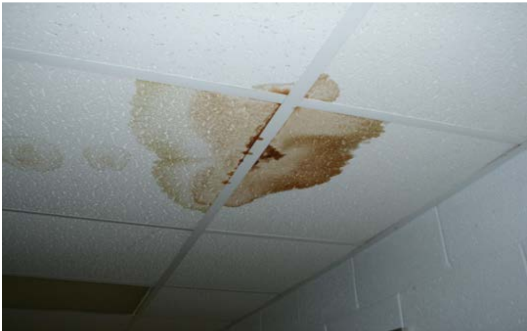
Water Damaged Ceiling Tile in corridor
