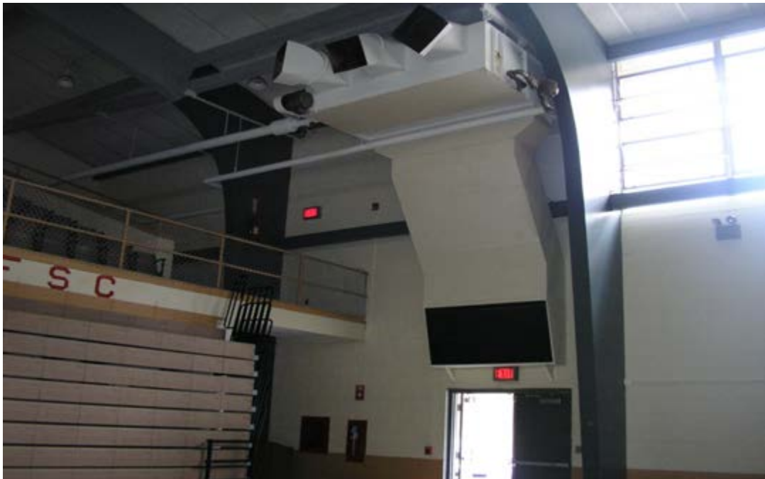
View of Radiant Heat Unit In Assembly Hall
