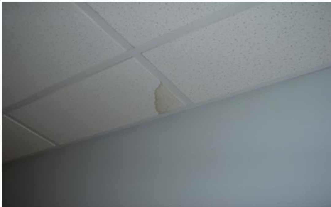
Water damaged ceiling tile in corridor
