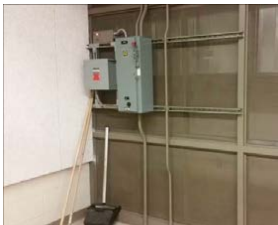
Photo D1. Control box on plenum wall blocking airflow.
