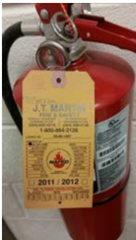
Photo D9. Fire extinguisher with expired annual inspection tag.
