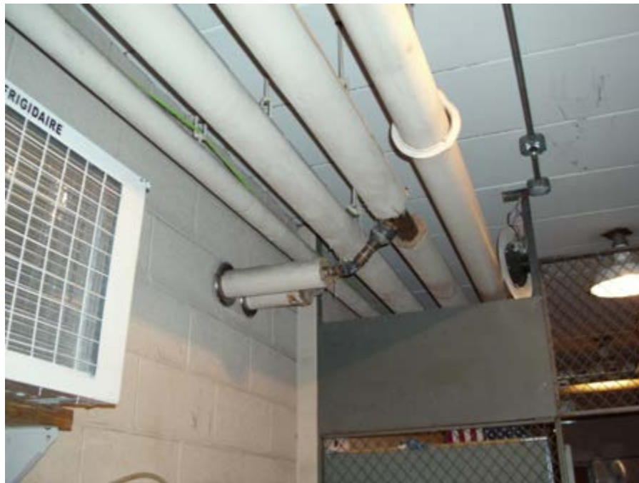
Typical Fiberglass Pipe Insulation
