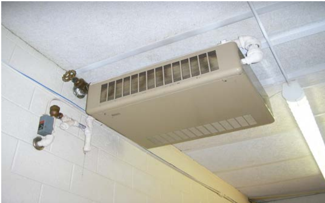
View of Radiant Heat Unit in Corridor
