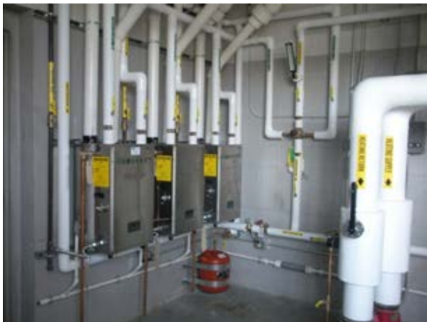
Photo 7: New tankless hot water heaters.
