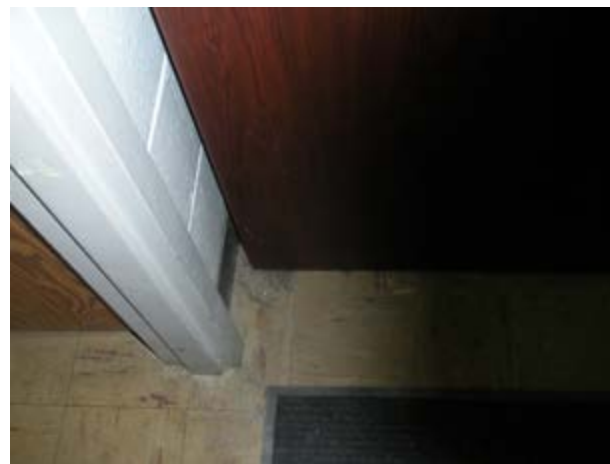
Photo 16: View of broken asbestos-containing floor tile typical of damage in the office areas.
