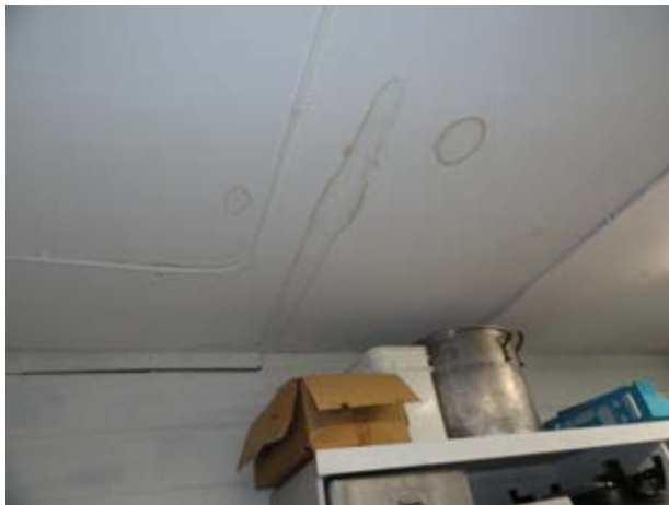
Water Damage on Ceiling
