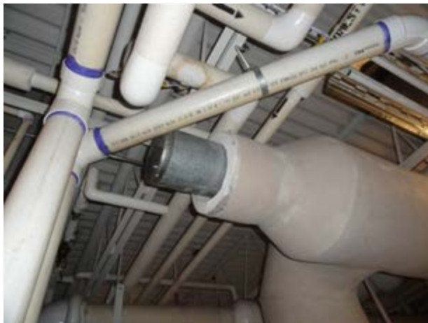
Boiler Room – damaged insulation
