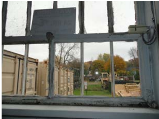
Deteriorating glaze and paint on windows
