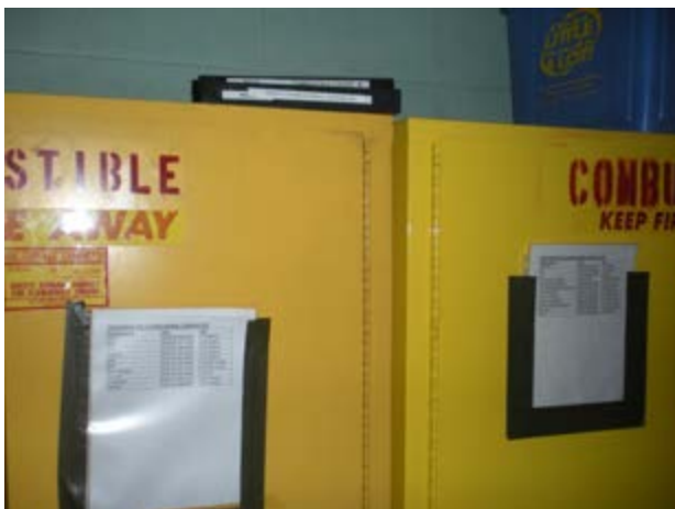
Photo 11: Flammable materials storage cabinets with MSDS book.
