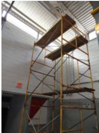
Scaffolding to fix a leak
