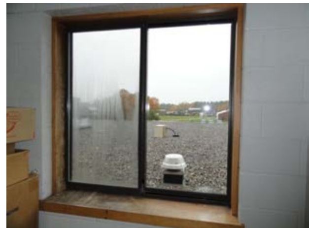
Window with water intrusion
