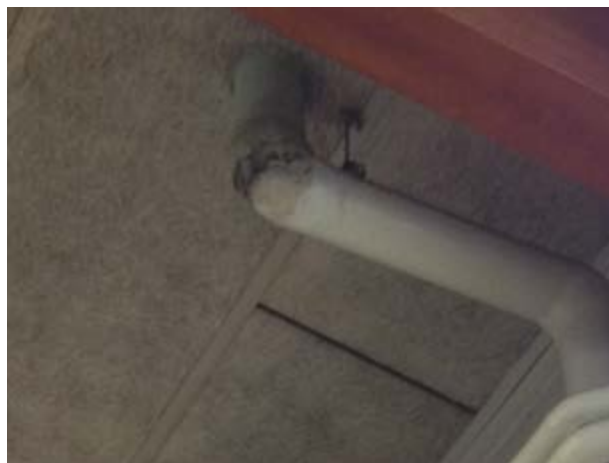
Photo 20: Damaged Roof Drain Fitting at Roof Deck of Drill Hall
