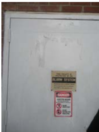
Photo 15: View of damaged paint on metal exterior door. The paint was tested and is not lead-based.
