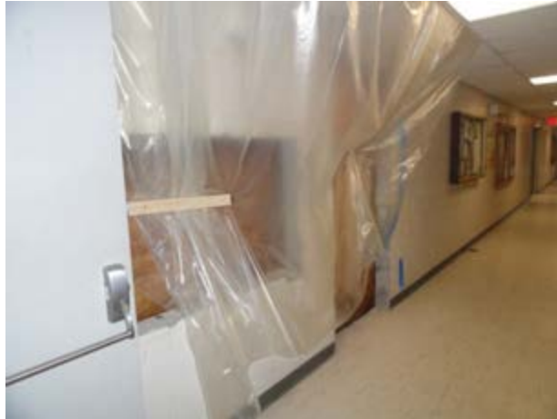
Containment near area being renovated
