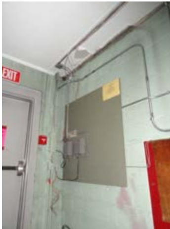
Same peeling paint and broken plaster as 2011 Survey
