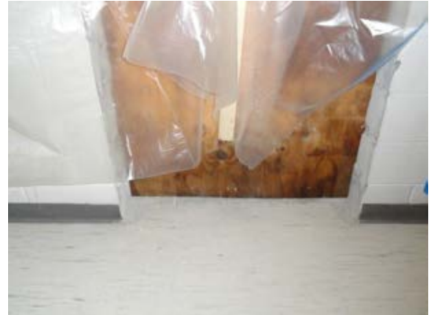
Containment does not go to floor to prevent dust from entering hallway
