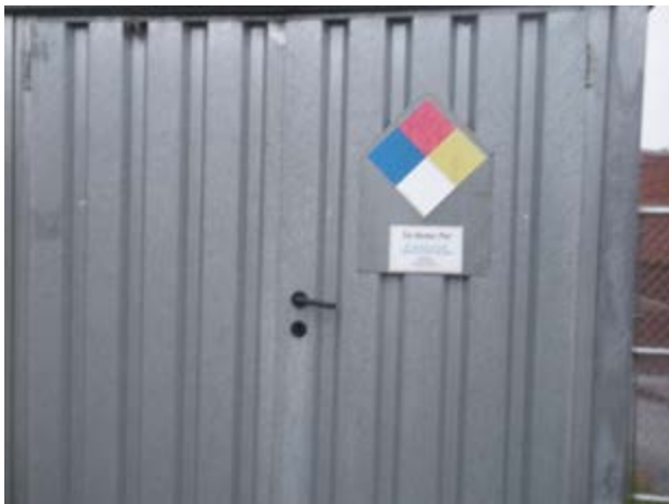
Photo 7: Storage locker located in fenced outdoor storage area. Note: the NFPA signage is missing applicable hazard classifications.
