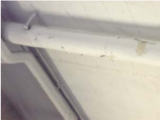
Photo 21: Peeling Paint on Roof Drain in Drill Hall
