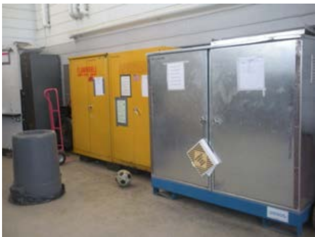
Photo 7: POL and flammable cabinets in Drill Hall. Note doors to POL storage cabinet do not function properly.
