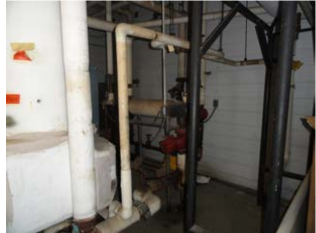
Boiler Room Pipe Insulation
