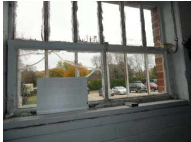
Deteriorating glaze and paint on windows
