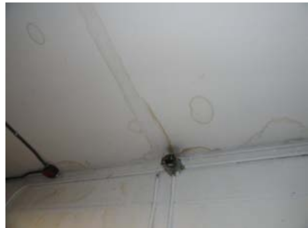
Water Damage on Ceiling
