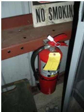
Photo 3: Fire extinguisher tags did not indicate recent inspection.
