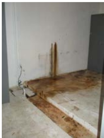
Photo 17: Water damage from active water leak in lower level former range area.
