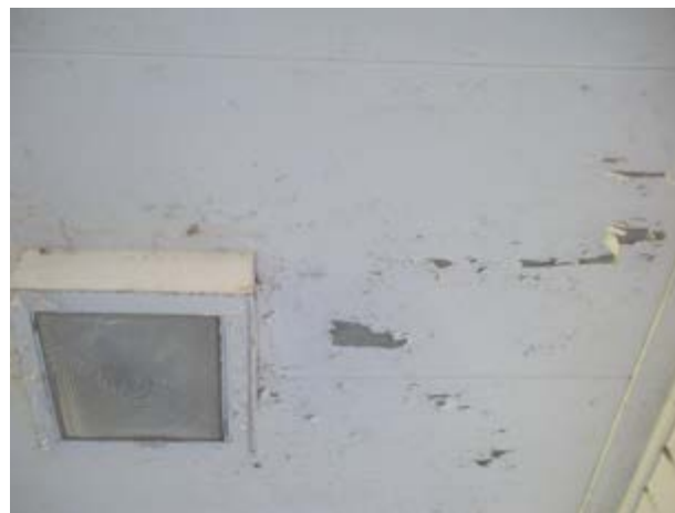
Photo 14: View of peeling, flaking and chipping lead-based paint on porch ceiling.
