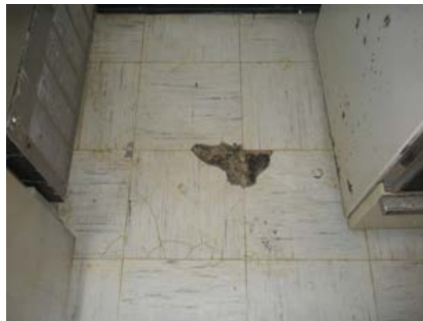
Photo 6: Damaged floor tile with exposed mastic in kitchen.
