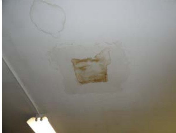
Water Damage on Ceiling
