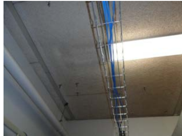
Insufficient lighting in telecom closet
