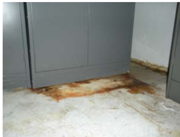
Photo 18: Water damage from active water leak in lower level former range area.
