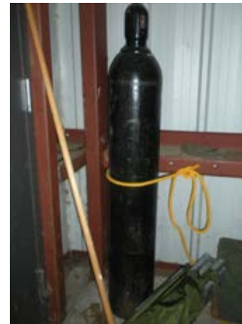
Photo 2: Improperly secured compressed gas cylinder.
