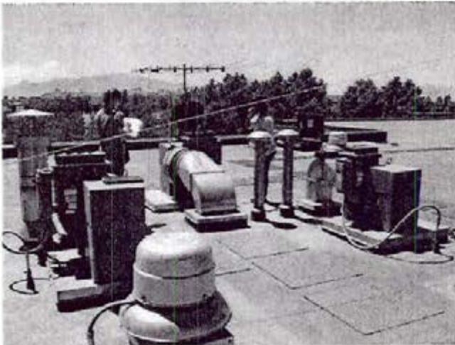
Photograph 3 Kitchen exhaust ducts, exterior
