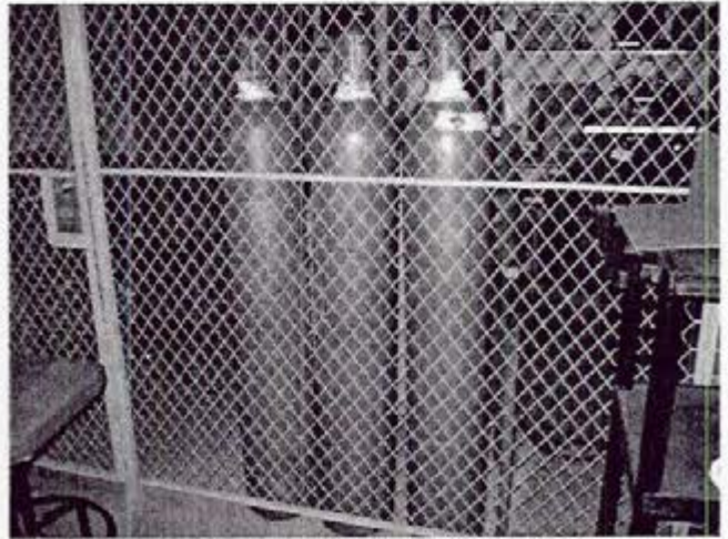
Photograph 10 Safety: Unsecured compressed gas cylinders
