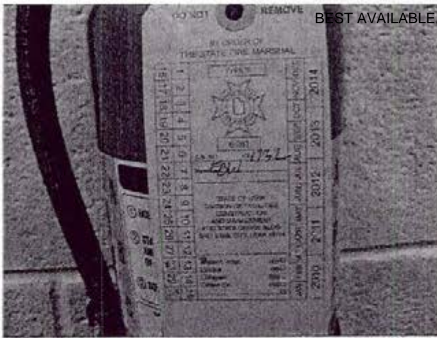
Photograph 7 Safety: Expired fire extinguishers
