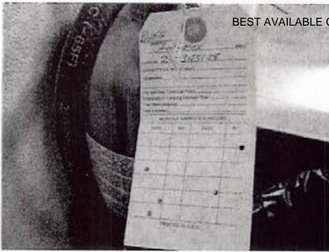
Photograph 7 Fire Extinguisher without Monthly Inspection
