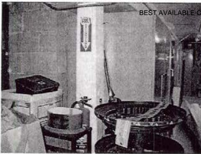
Photograph 7 Blocked fire extinguisher in the basement of 32 Potter
