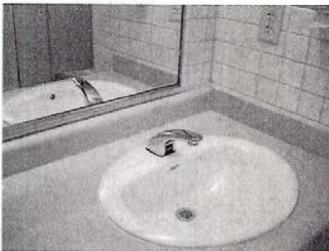
Photograph 9 Non-GFCI protected outlet within 6 feet of water source in Building at 31 Potter
