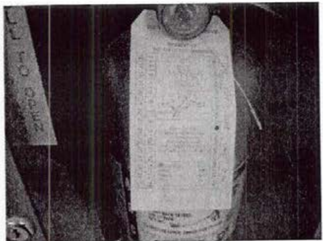
Photograph 4 Logan Armory, Fire extinguisher not current on annual inspection in kitchen
