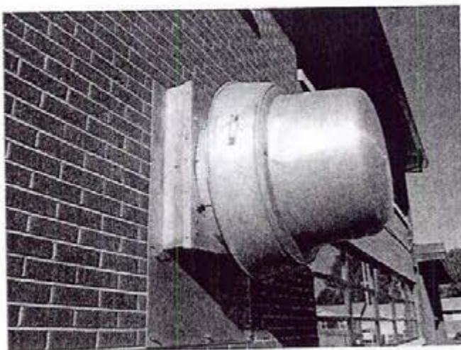
Photograph 5 Kitchen exhaust duct, Exterior
