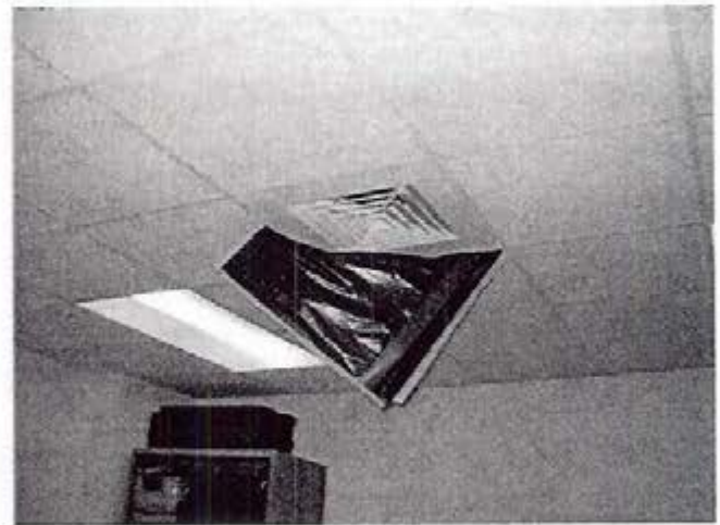
Photograph 12 Vents covered due to cold air blowing in during winter
