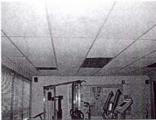
Photograph 9 Water-damaged Ceiling Tile
