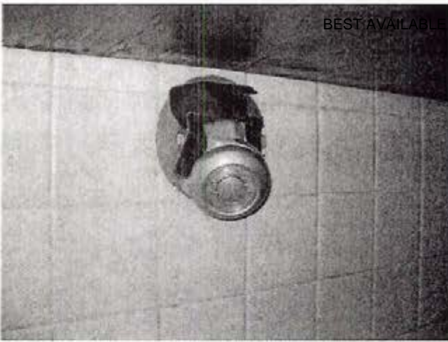
Photograph 13 Exposed wiring in breakroom
