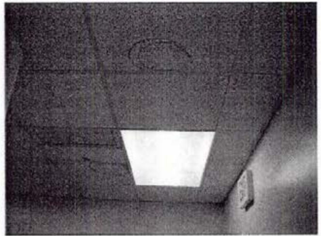
Photograph 10 Water-stained ceiling tiles located in central area of building
