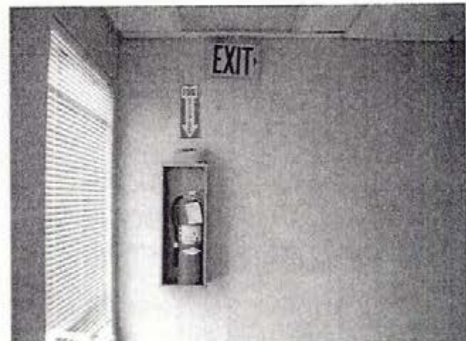
Photograph 6 Fire extinguishers without monthly or annual inspections and Egress signs not working
