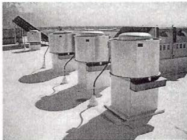
Photograph 6 The three roof-mounted vents for kitchen
