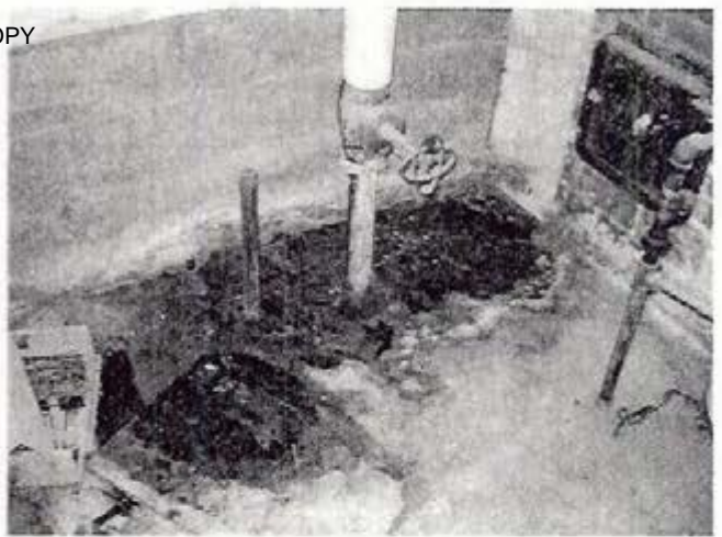
Photograph 8 Water leak and fungal growth in mechanical room
