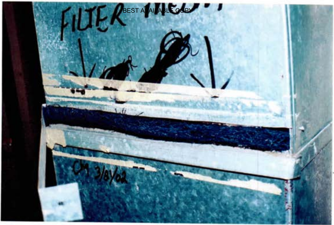
A/C-HEATING UNIT, FILTER
