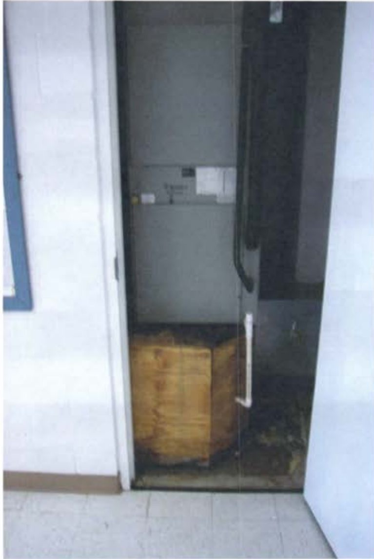
Photo #17: Water damaged wood return air plenum in the mechanical closet.
