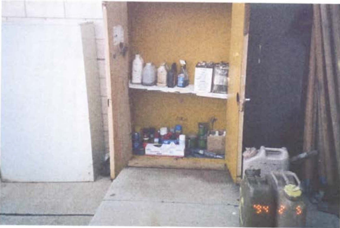
View of Hazardous Materials stored in a Flammable storage cabinet
