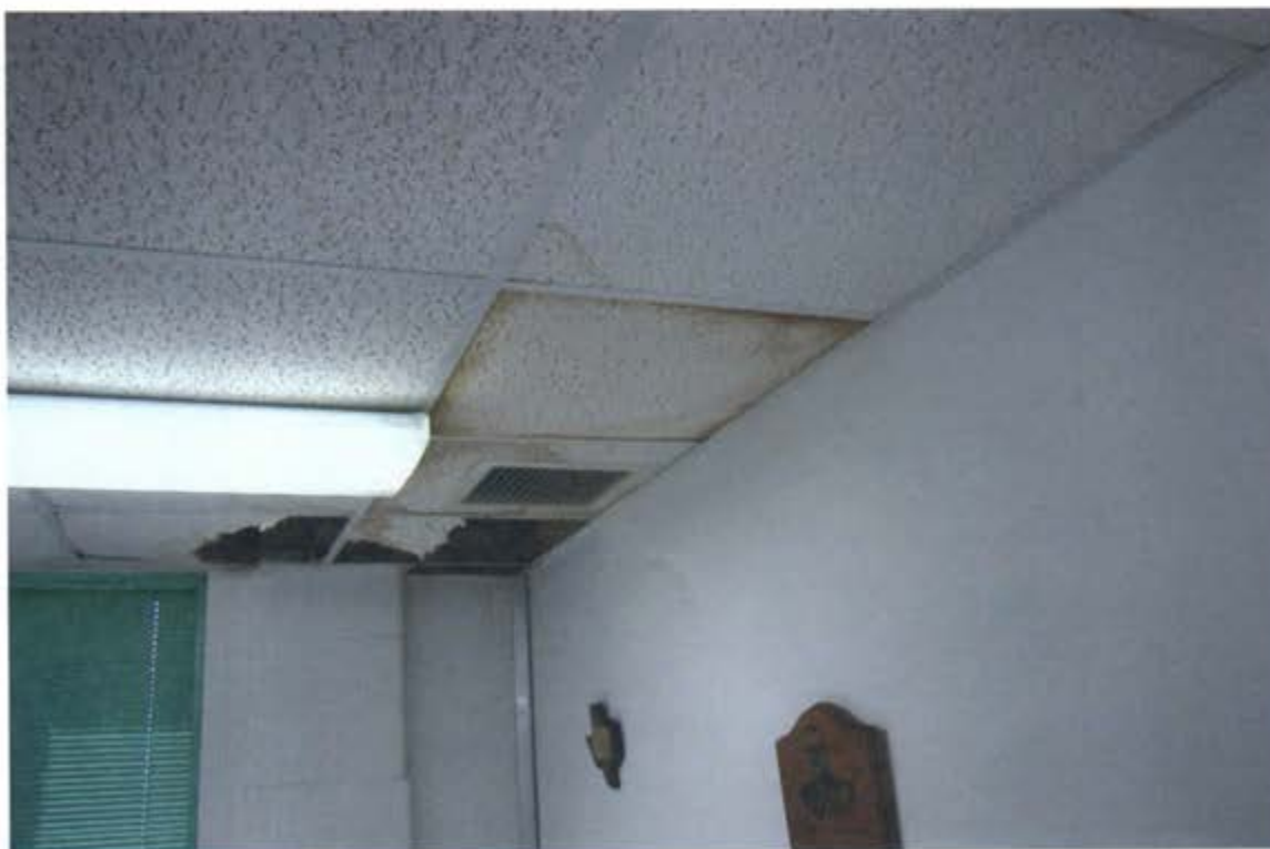
Photo #14: Water damaged ceiling tiles in the administrative area.
