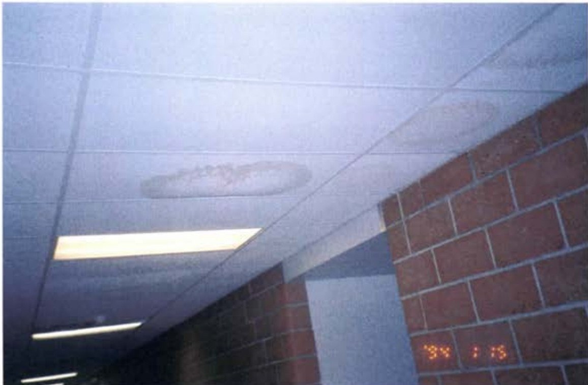
View of water leak in the classroom hallway ceiling
