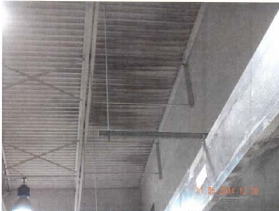
Potential Mold – Drill Floor Ceiling
