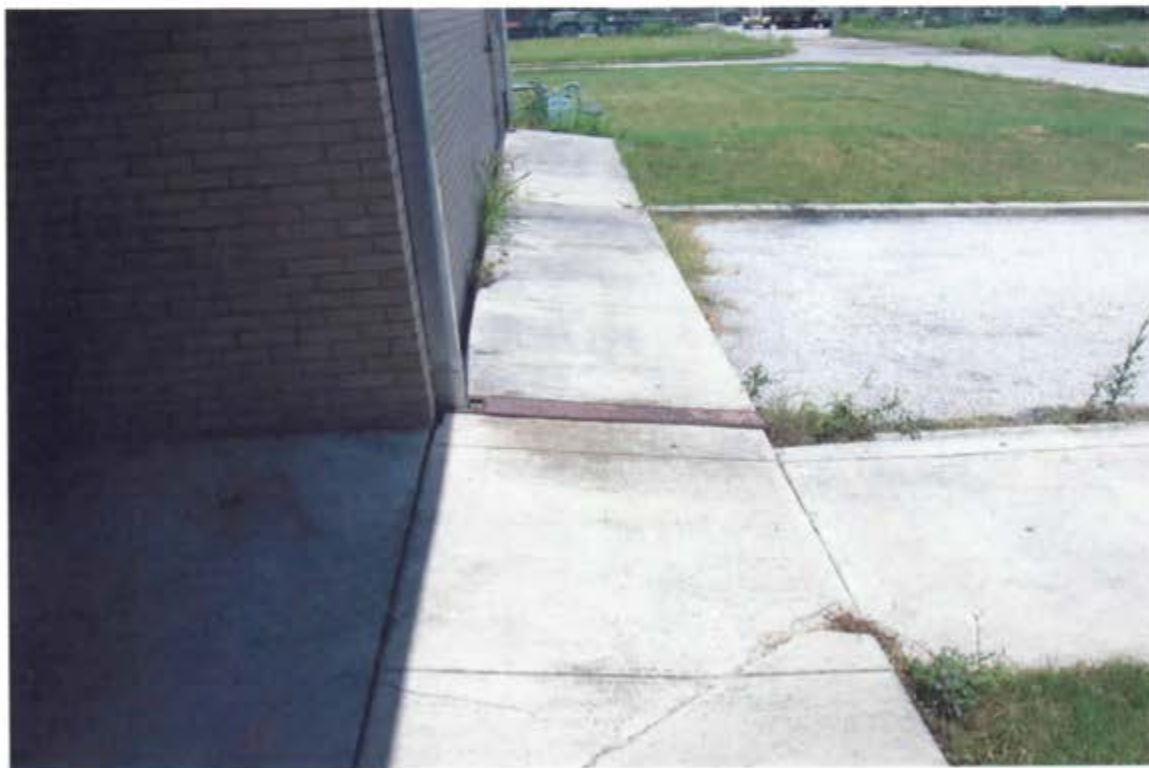
Photo #12: Sidewalk separation on the west side of the armory due to ground settling.
