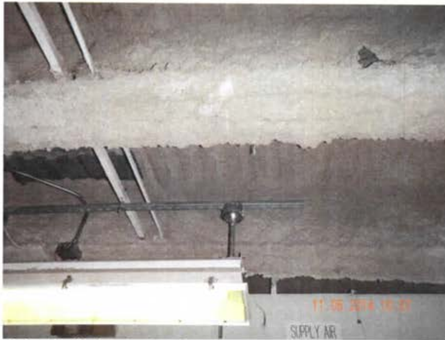
Potential Asbestos Insulation - Test Results were negative
