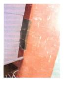
Drop ceiling below suspect asbestos tile...extensive water damage
