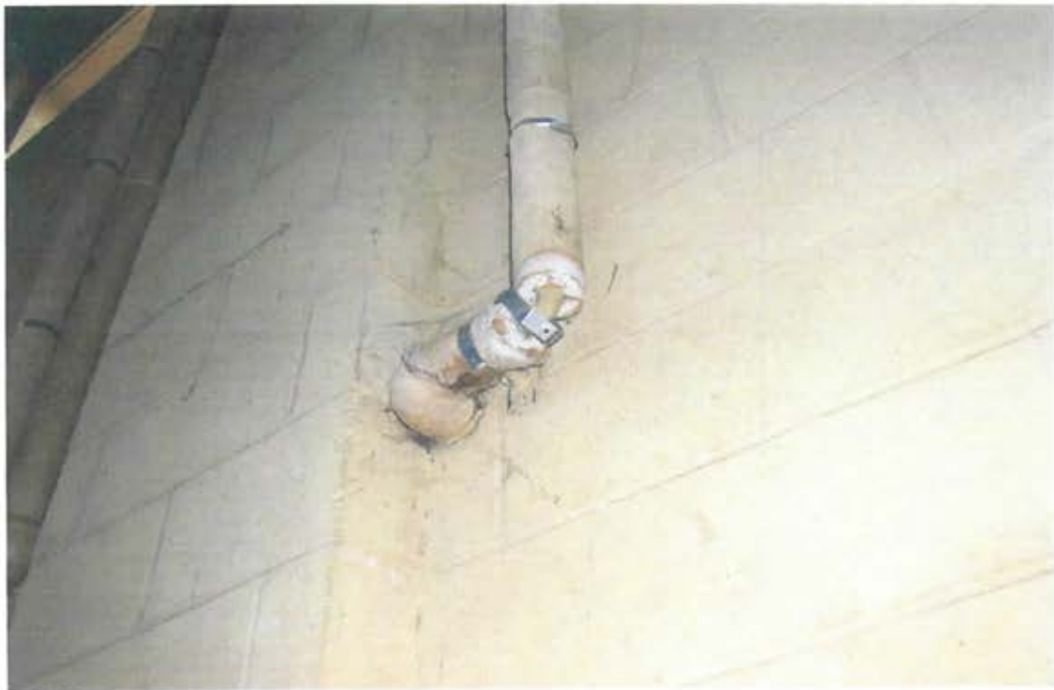
Photo 14: Thermal pipe insulation found in the drill hall.
