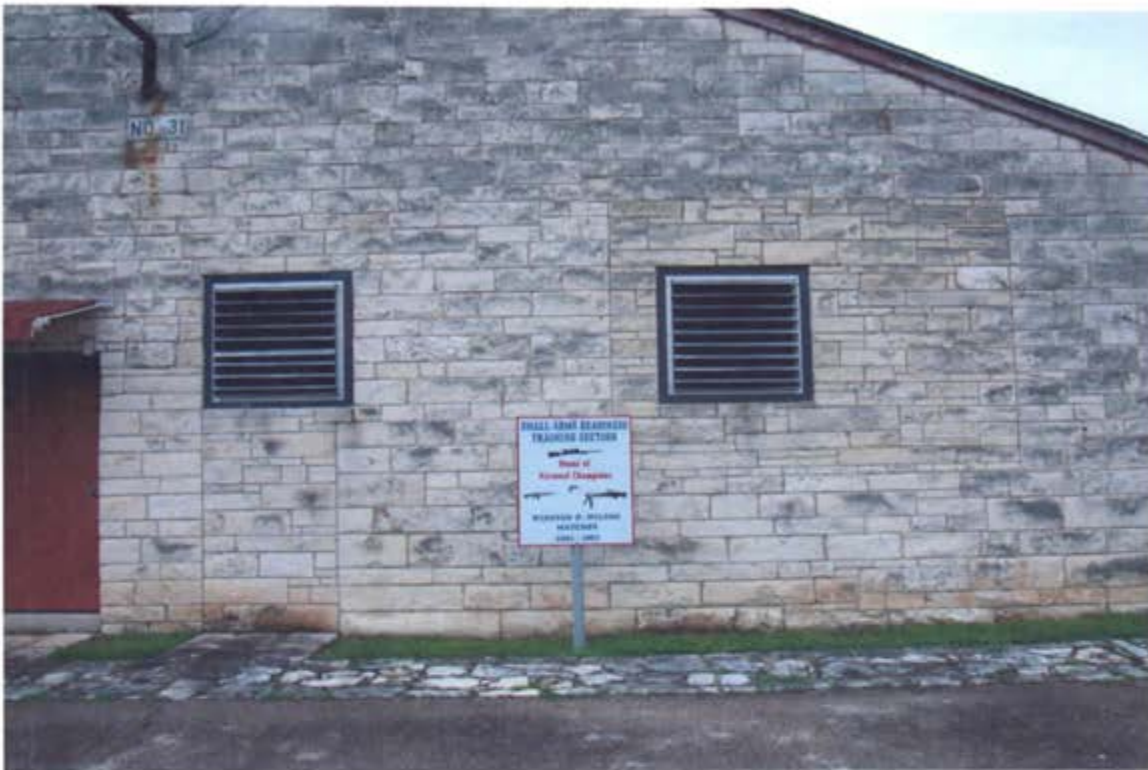
Photo 5: Exhaust fan outlets behind the bullet trap.
