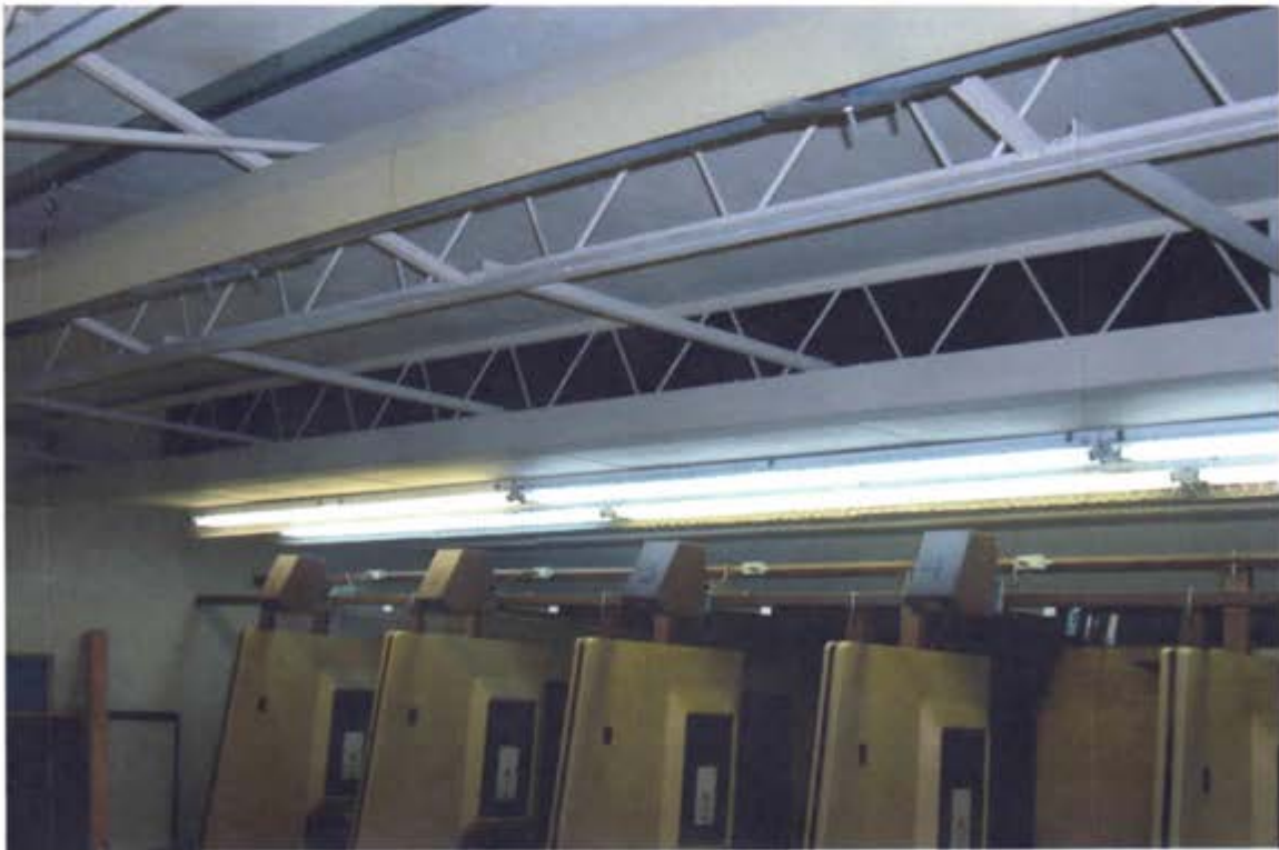
Photo 14: The dropped ceiling opening where makeup air is introduced into the range.
