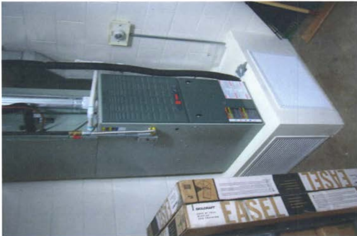
Photo #10: Furnace units showing the wooden common return plenum
