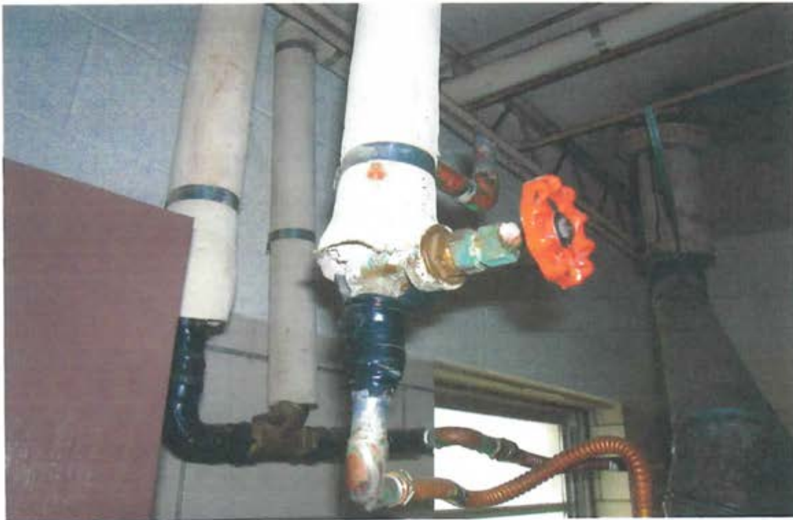
Photo 12: Sampled thermal pipe insulation found on the hot water system.
