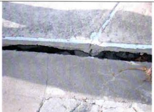
Cracked Concrete At Sinkhole, Rear Of Building
