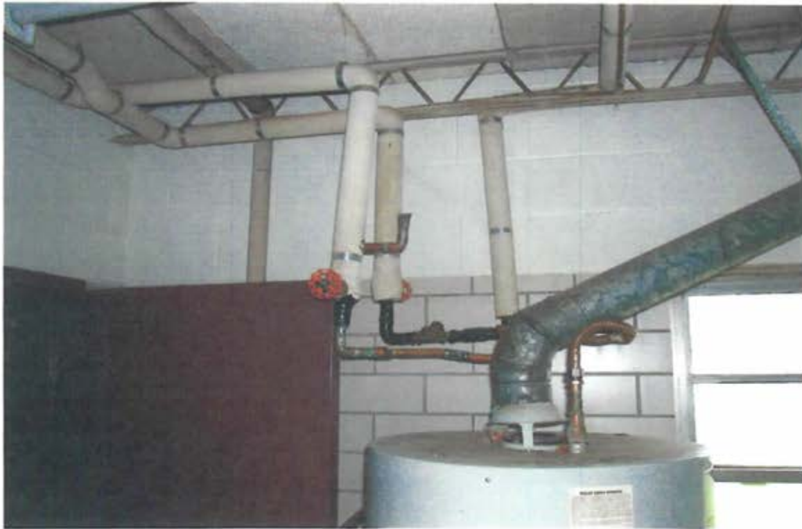
Photo 9: Hot water heater and the insulated hot water pipes.
