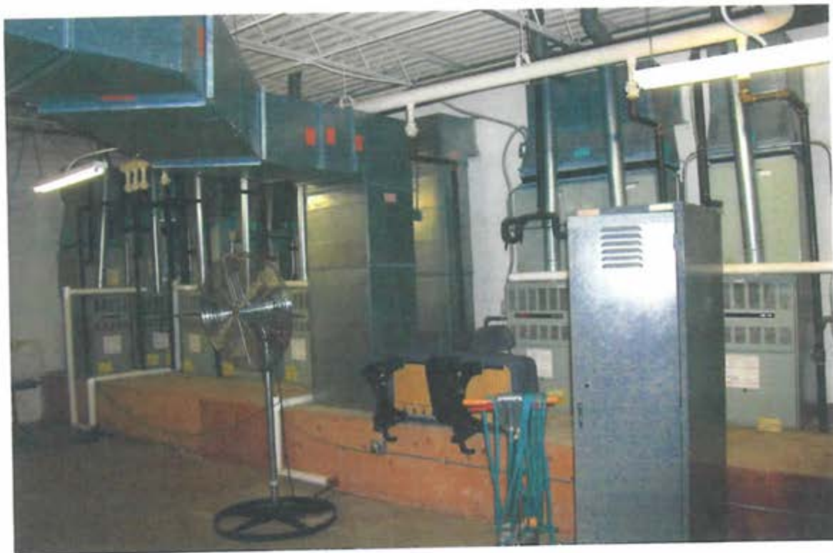
Photo 14: Air handlers in the mechanical room showing the wooden common plenum under the units.
