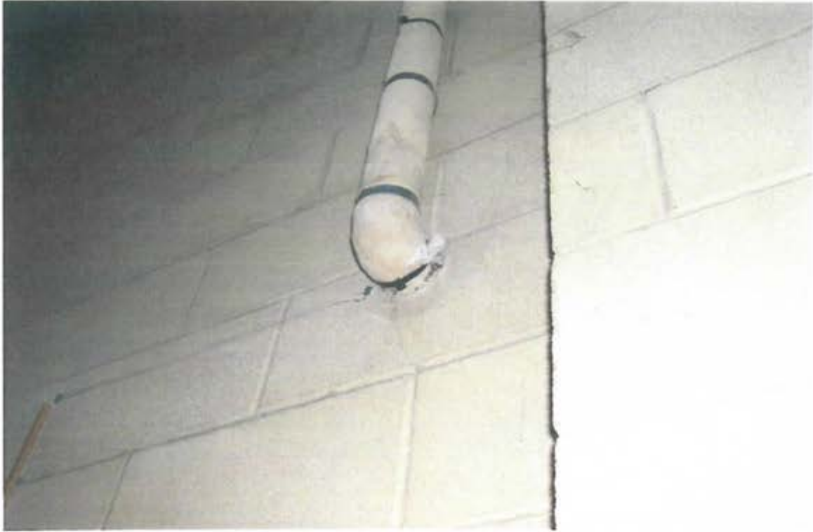
Photo 13: Sampled thermal pipe insulation found in the drill hall.
