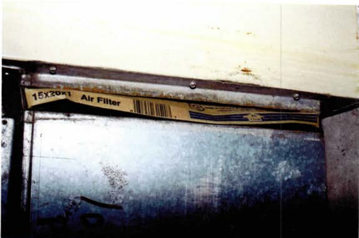
A/C-HEATING UNIT FILTER
