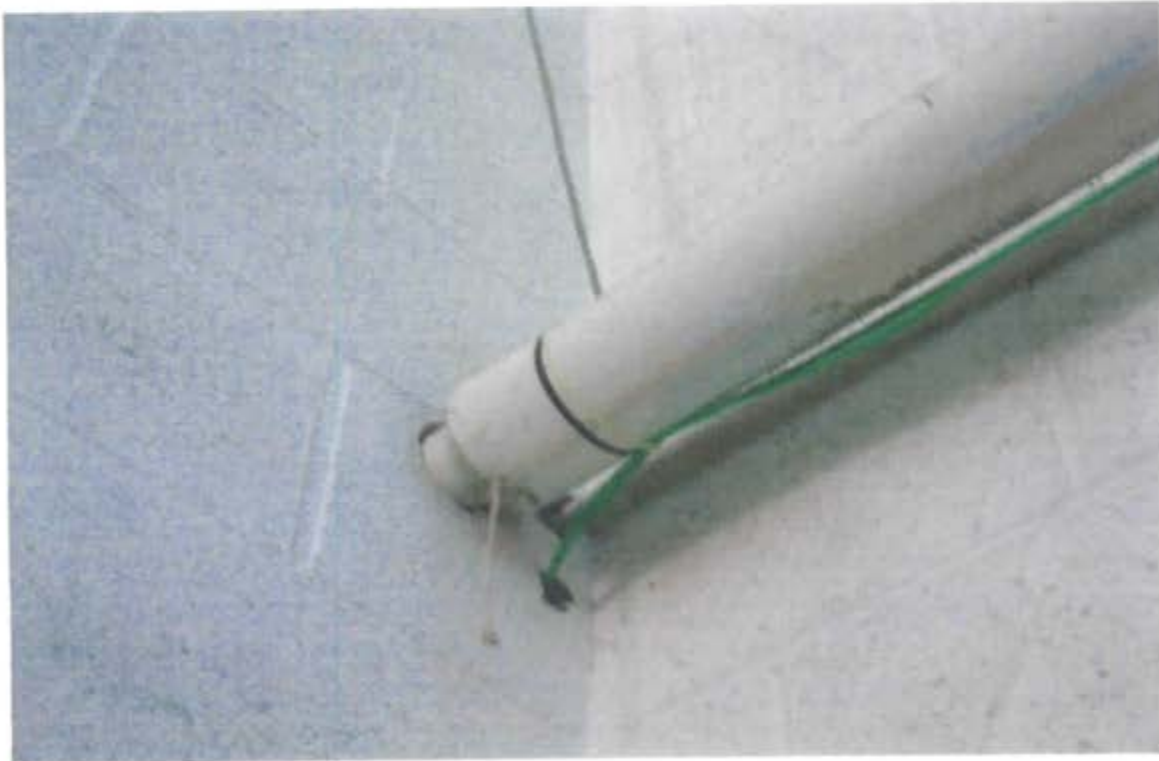
Photo 20: Thermal pipe insulation in drill hall..
