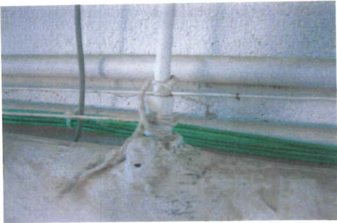
Photo 19: Thermal pipe fitting insulation in the drill hall.
