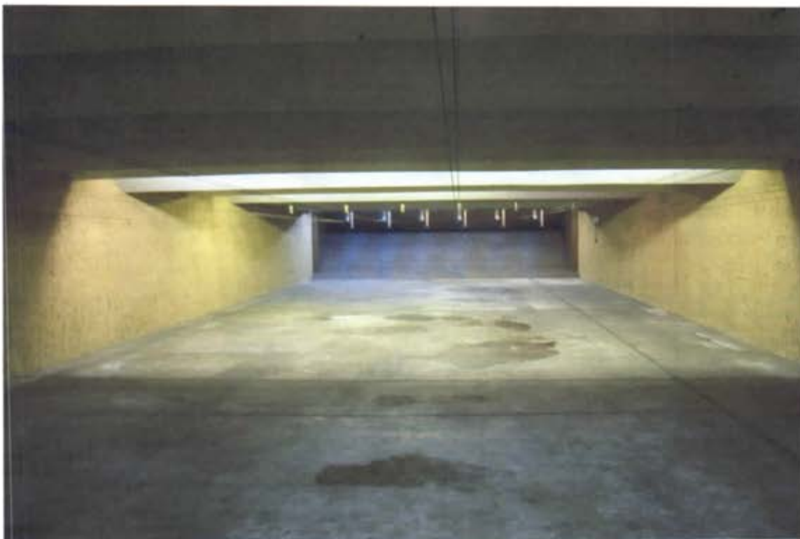
Photo 3: The bullet trap.
