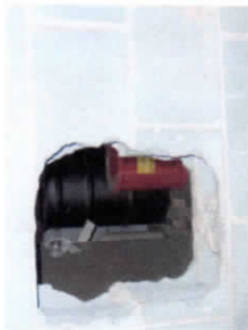
Hole knocked in wall, no ventilation present
