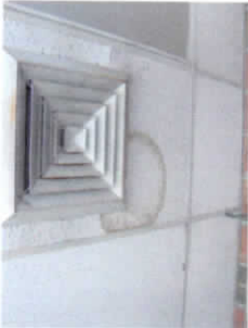
Water damaged ceiling tiles
