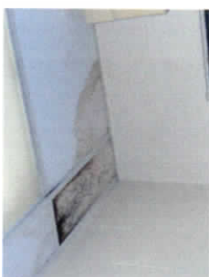
Water damaged ceiling tiles
