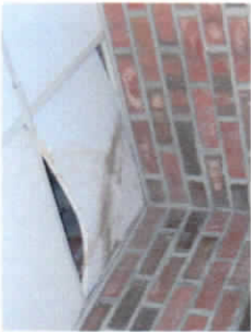
Water damaged ceiling tiles
