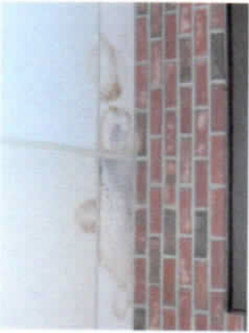
Water damaged ceiling tile
