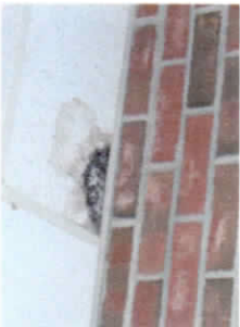
Water damaged ceiling tile
