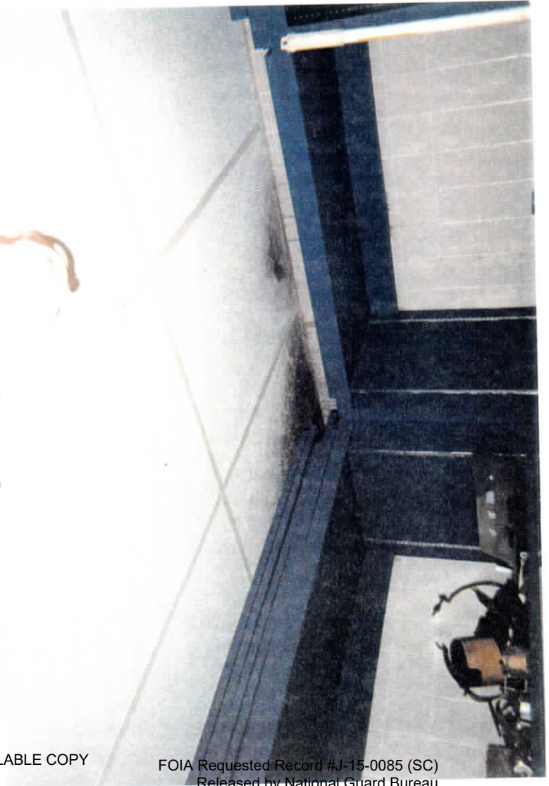
H2O damaged ceiling tile
