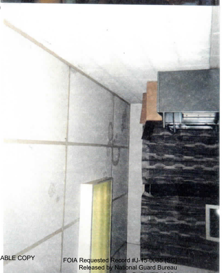
H2O damaged ceiling tile
