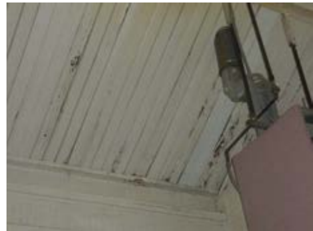
Deteriorating Paint on Drill Hall Ceiling
