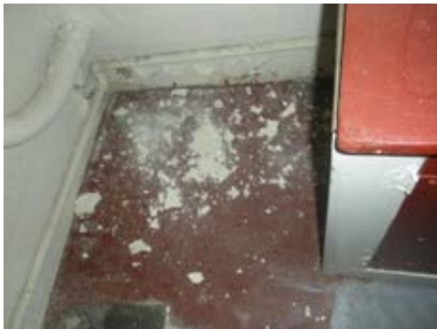
Delaminated Peeling Paint on Floor
