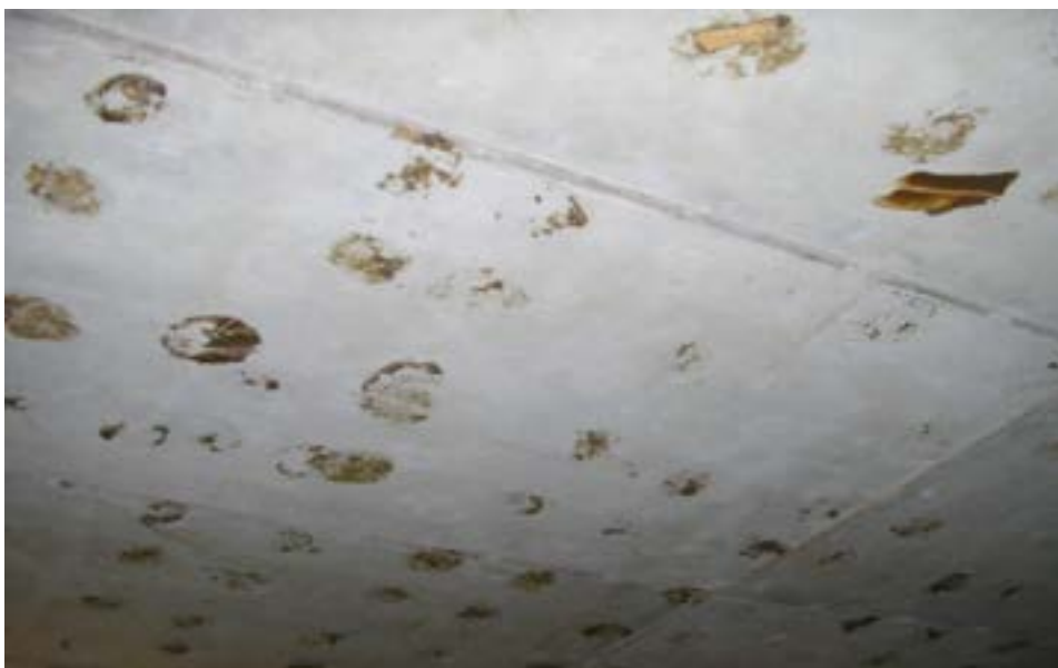
View of Damaged Ceiling Tile Adhesive in Former Fire Range
