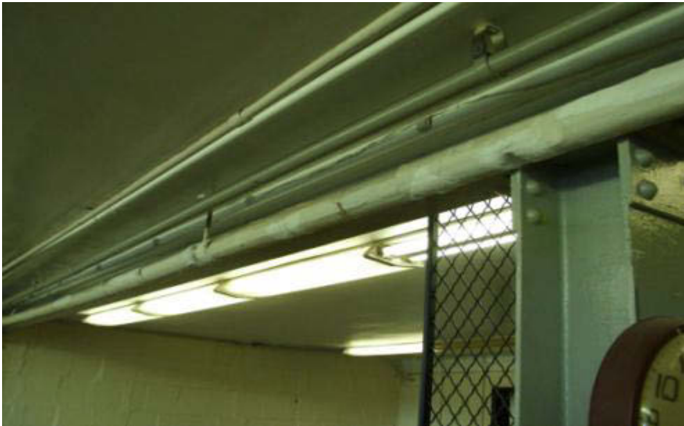
Basement Classroom - ACM Pipe Insulation
