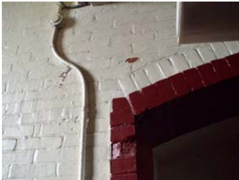
View of damaged paint in stairwell
