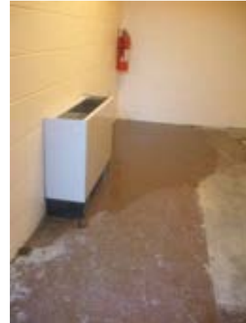
Ponded Water inside Entrance to Building with no Drainage
