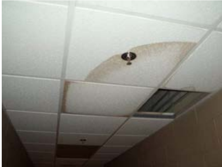
View of water damaged ceiling tile in corridor
