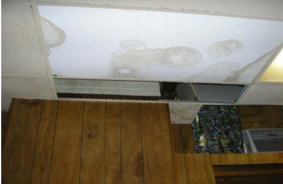
View of Water Damage in Upper Floor Office
