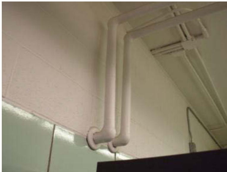
Fiberglass Pipe Insulation with ACM Fittings
