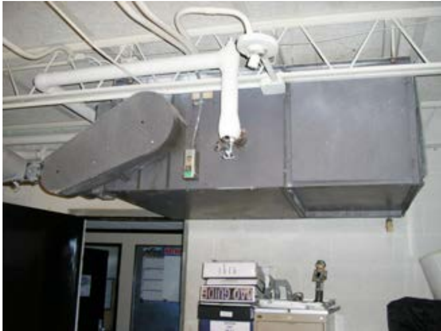
View of Suspect Asbestos Pipe Insulation and Radiant Heater in Office
