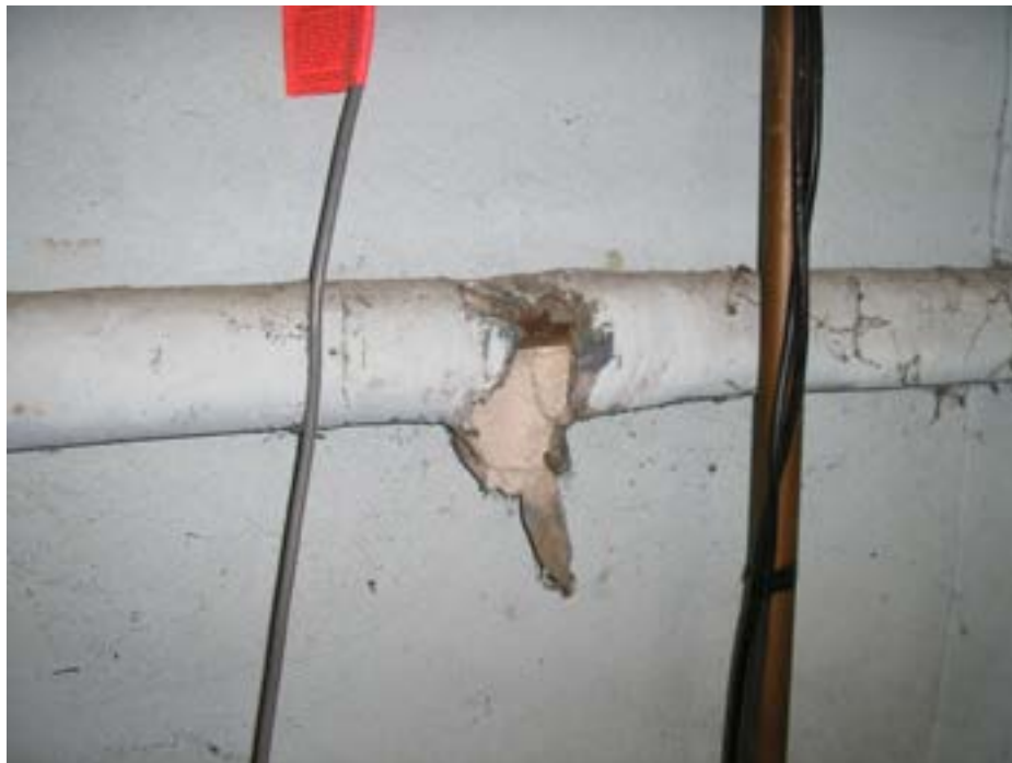
View of Damaged Pipe Insulation – Service Bay
