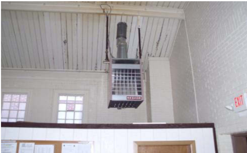
Unit Heater In Drill Hall
