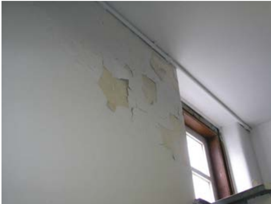
View of Peeling Paint – 2 nd floor stairway
