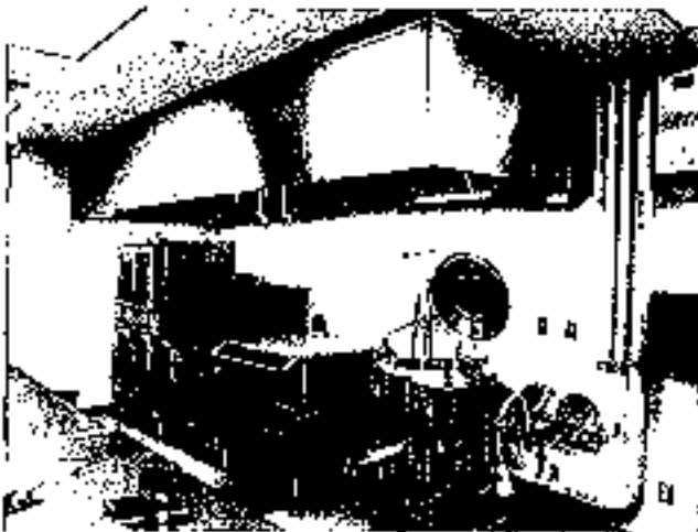
Kitchen Convection Oven with Exhaust Hood
