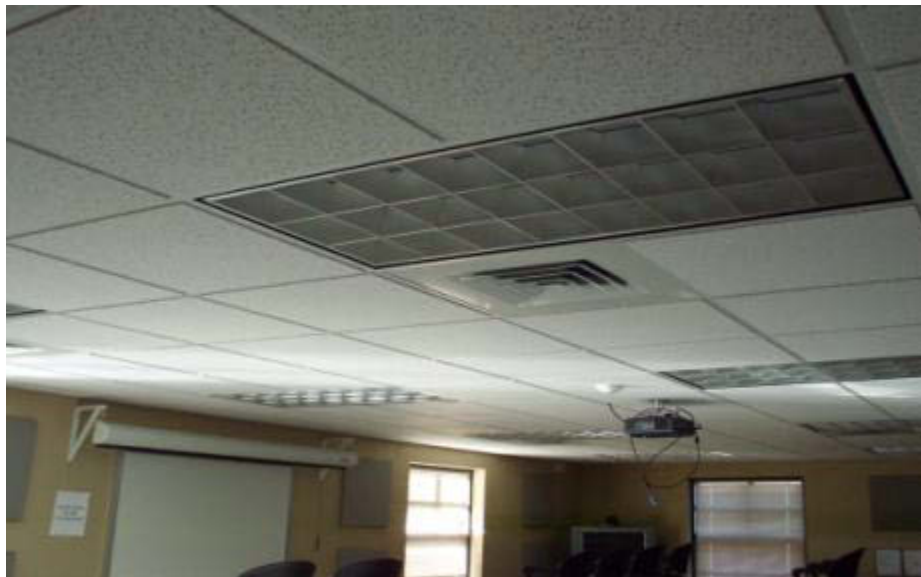
Typical HVAC Supply Grille
