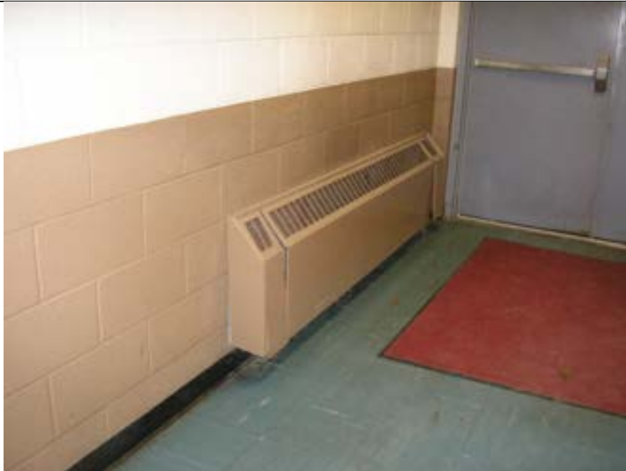
View of Radiant Heat System in Corridor
