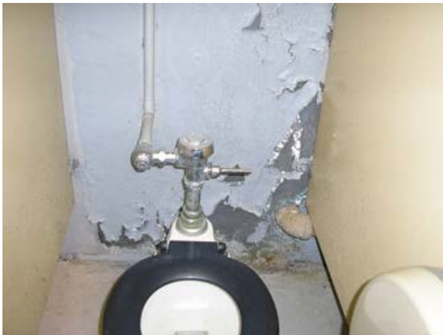
View of Peeling Paint – men's basement restroom
