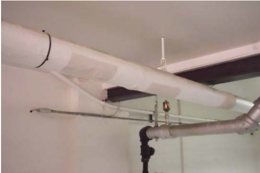
Basement Corridor - ACM Pipe Insulation
