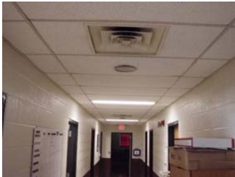
View of typical HVAC supply grille
