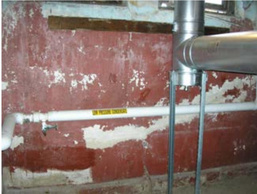
View of Peeling Paint - Boiler Room
