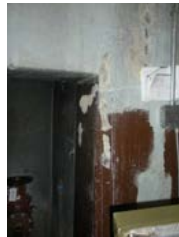
Peeling, Flaking, Chipping Paint in Mechanical Room
