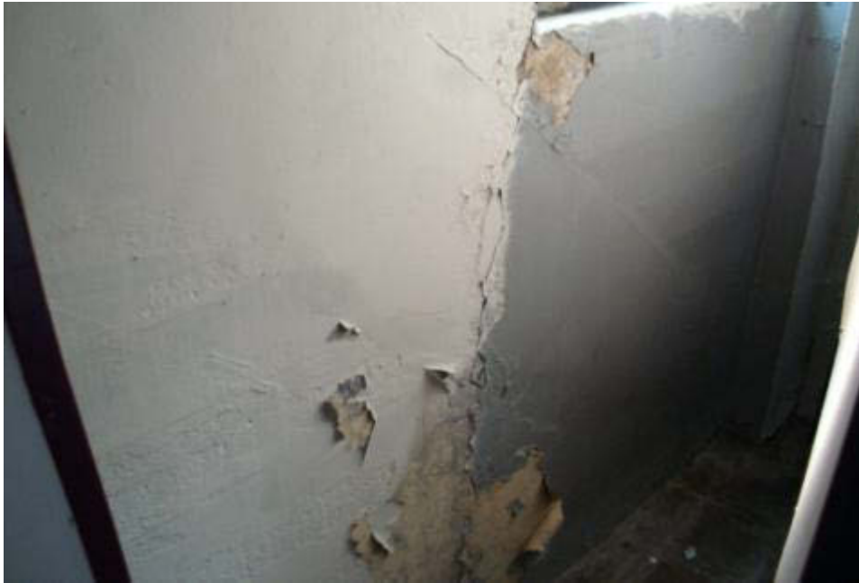
Damaged Paint Kitchen South Wall
