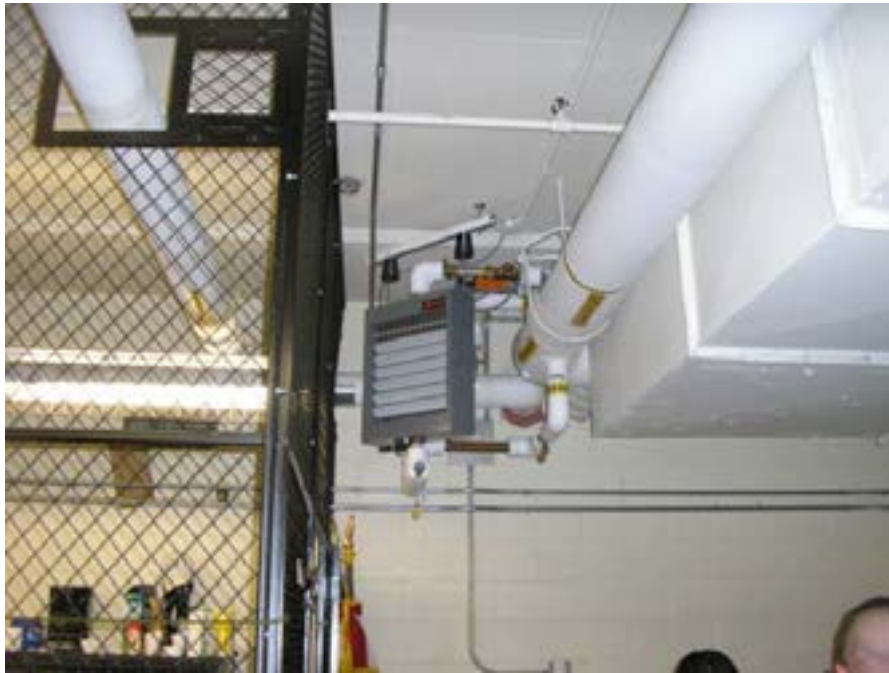
View of Typical Radiant Heater in Supply Room
