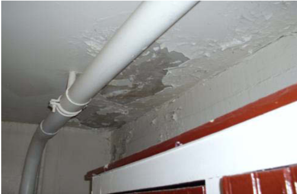
Damaged Kitchen Ceiling Plaster
