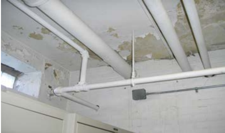
View of Peeling Paint and Water Damage in Lower Floor Office
