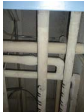
Asbestos Containing Thermal System Insulation
