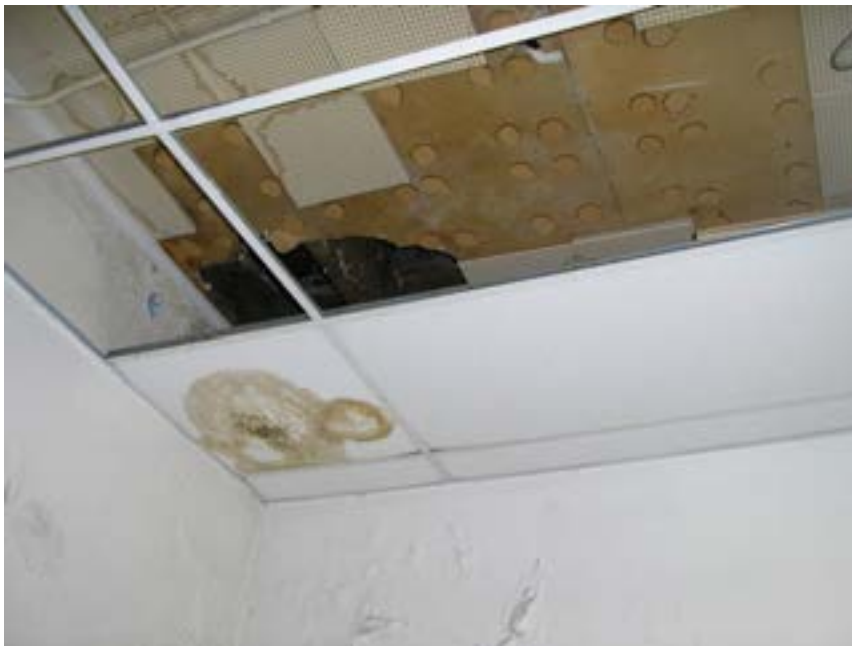
View of Water Damage – 2 nd floor meeting room
