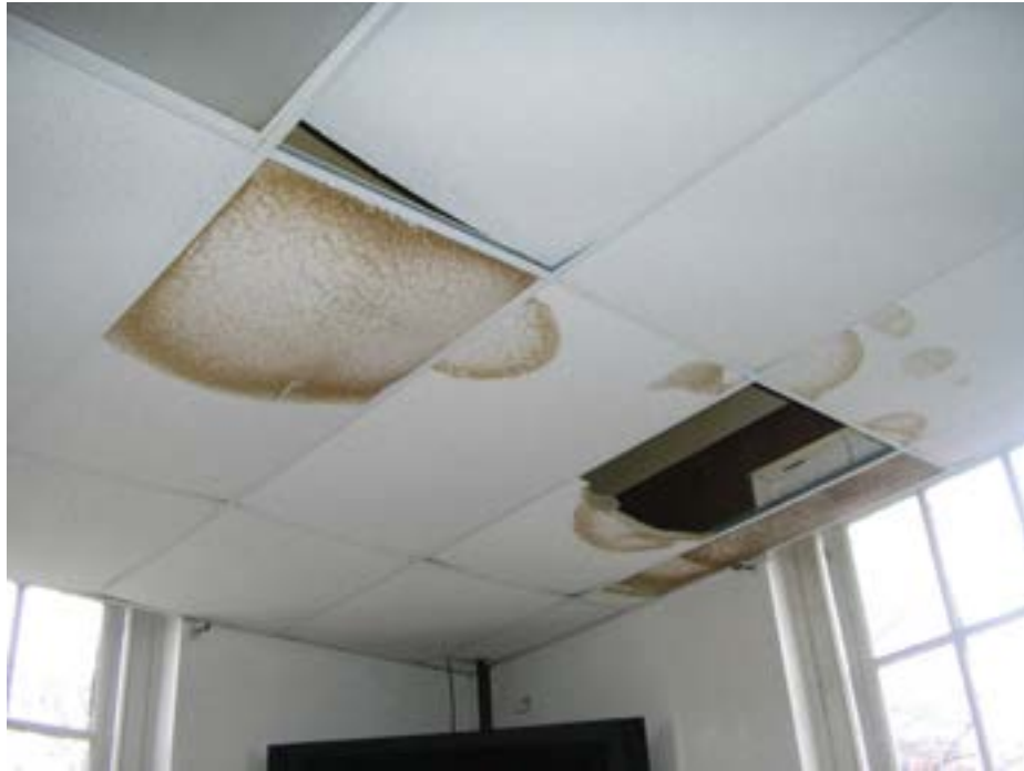
View of Water Damage in Break room
