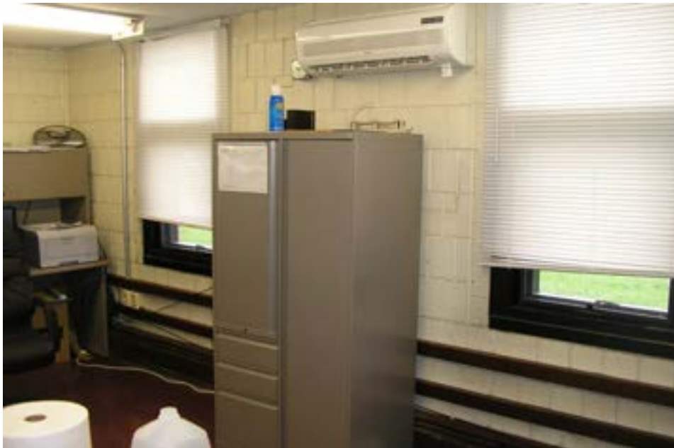
View of Wall-Mounted Air Conditioning Unit in Typical Office
