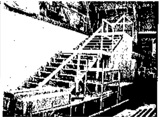
Safety - Mid Rail Missing on Stair Railing
