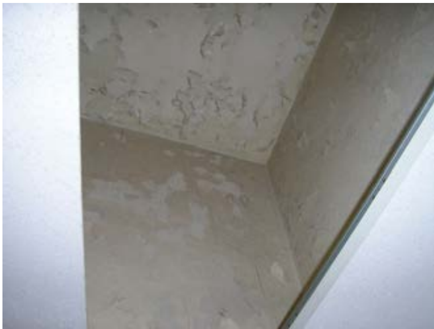
View of Peeling Paint – Assembly Hall Restroom
