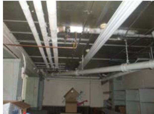
Asbestos Thermal System Insulation on 3 Pipes in F&E Store Rom
