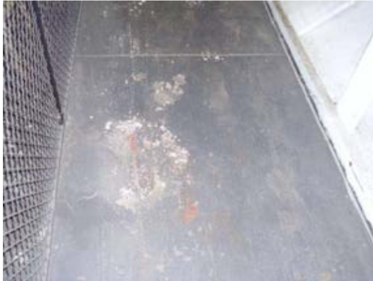
View of basement floor – damaged gray paint
