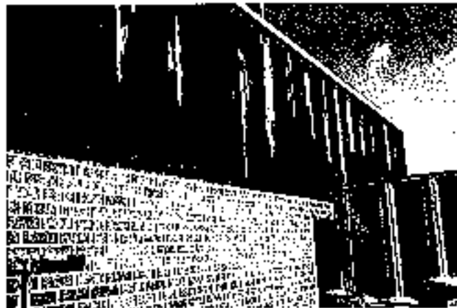
Exterior Peeling Paint
