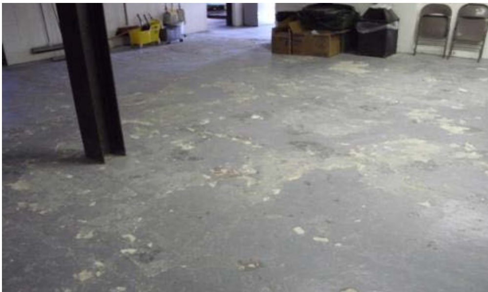
Damaged Paint Basement Floor
