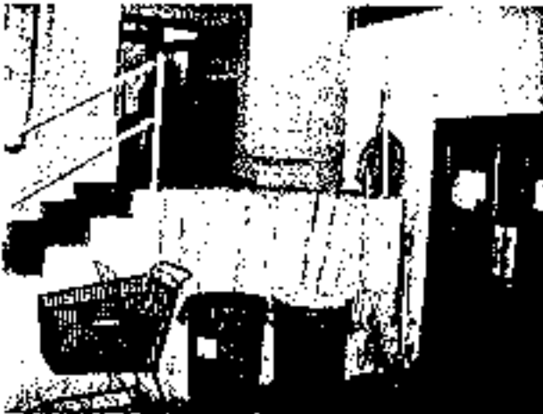
Safety - No Railing on Landing >4-Fect
