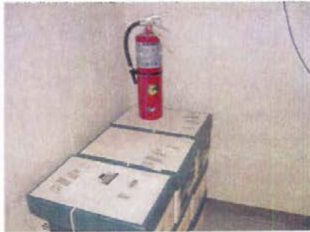
Photograph 18 Safety – Un-mounted fire extinguisher
