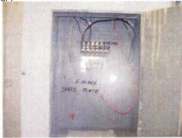
Photograph 20 Safety – Electrical panel box in mechanical room with exposed electrical wiring
