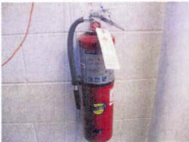
Photograph 17 Safety – Fire extinguisher without current annual or monthly inspections
