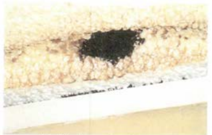
View of black substance (possible product from burning) located on the styrofoam ceiling tile in an office
