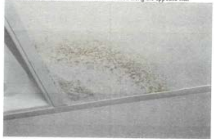
Mold and water stained ceiling tiles located in the main conference room
