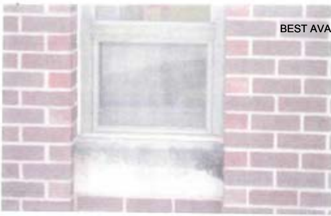
View of mold growth around concrete under window
