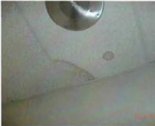
Damaged/Stained Ceiling tiles
