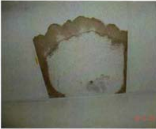
Damaged/Stained Ceiling tiles
