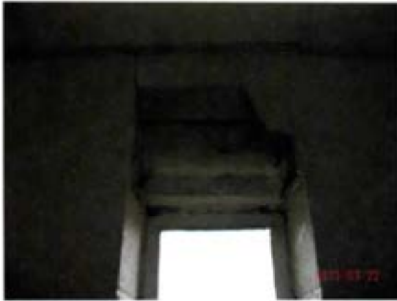
Broken cinder block above office window
