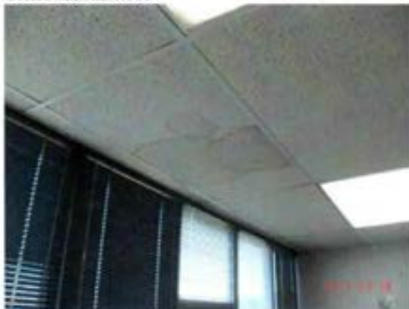
Damaged Ceiling Tiles
