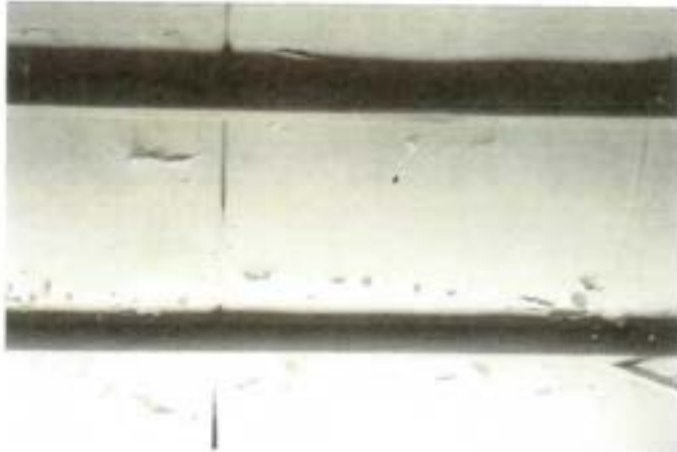
View of heavily peeling painted plastic ceiling of the drill hall.
