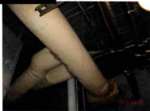
Insulation/no fraying or crumbling
