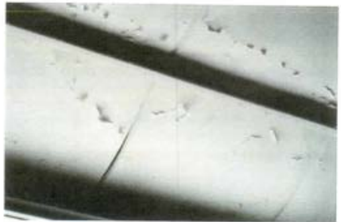
View of heavily peeling painted plastic ceiling of the drill hall.
