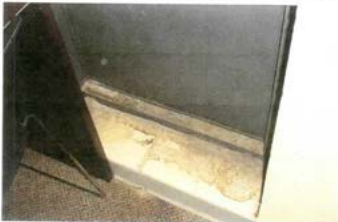
View of water infiltration under the sill in the office.
