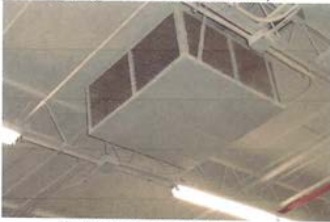
View of the room exhaust located within the fan cover
