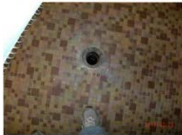
Drain cover missing/Could be a hazard
