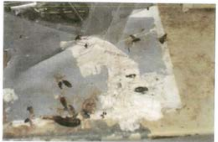
View of rodent droppings on air conditioning unit in HVAC room
