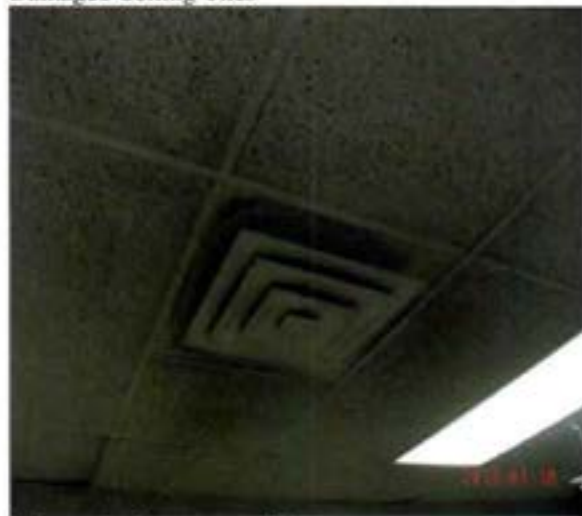
Exhaust/Intakes covered in soot
