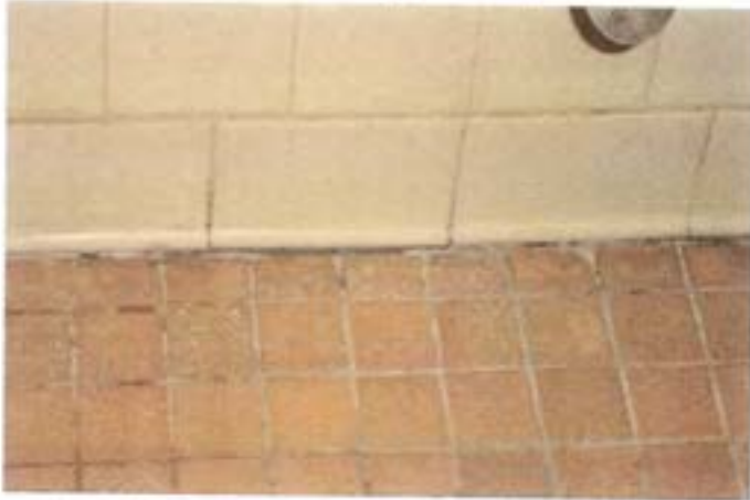
View of male latrine shower floor where water pools in the corner
