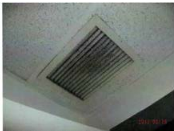
Exhaust/Intakes covered in soot
