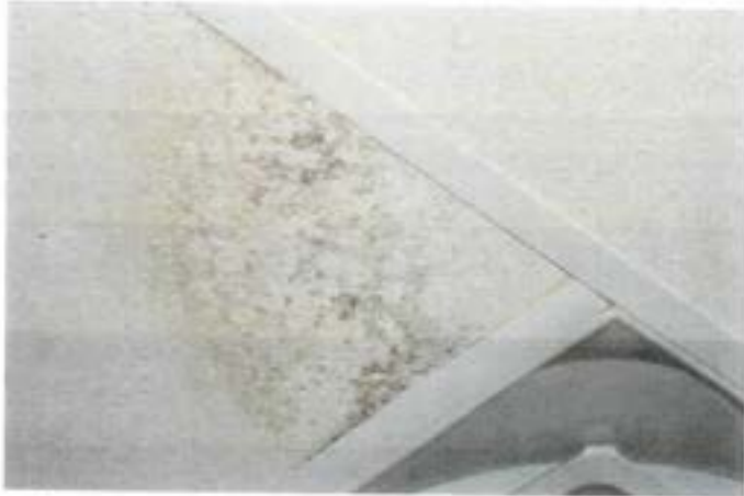
Mold and water stained ceiling tiles located in the main conference room
