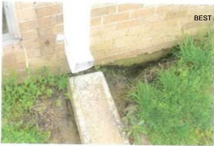
View of soil erosion at the buildings foundation
