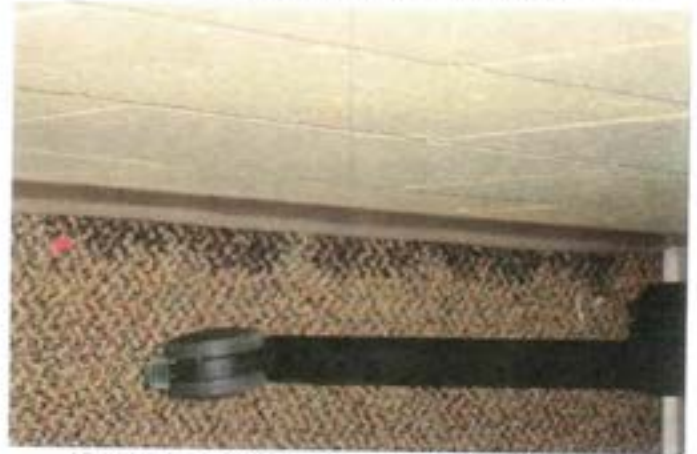
View of water infiltration (wet carpet) onto carpet in the main classroom water is from the shower located along the opposite wall
