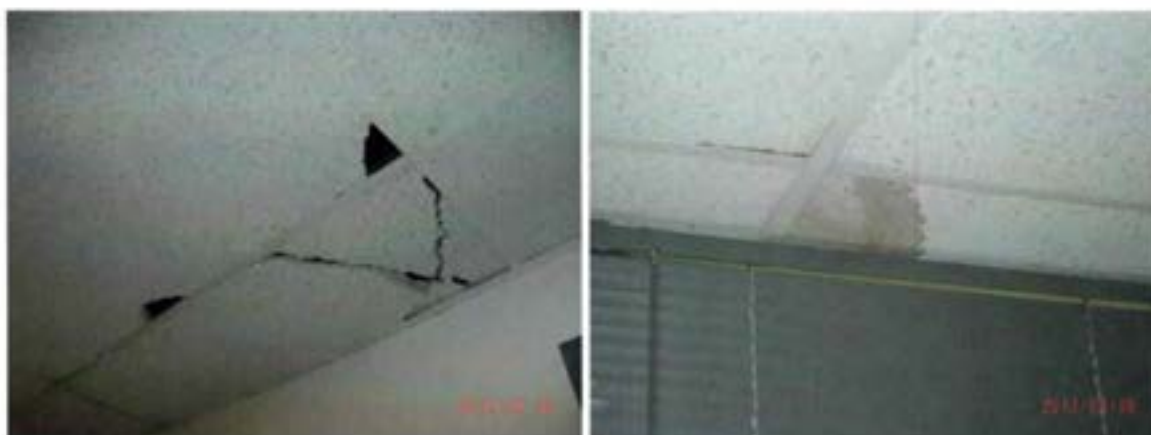
Ceiling tiles damaged and stained
