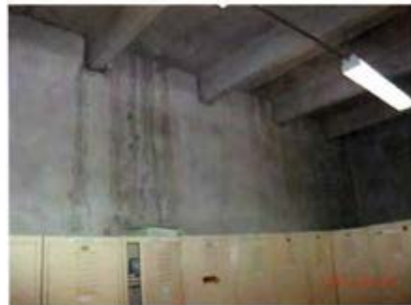
Basement/leak along wall
