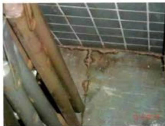
Water damaged floor in kitchen
