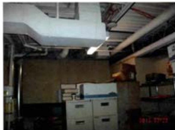
New Insulation covering pipes
