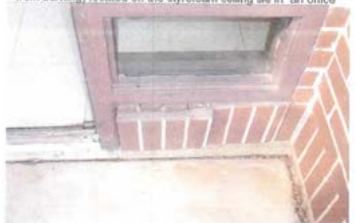
View of loose brick at entrance under window
