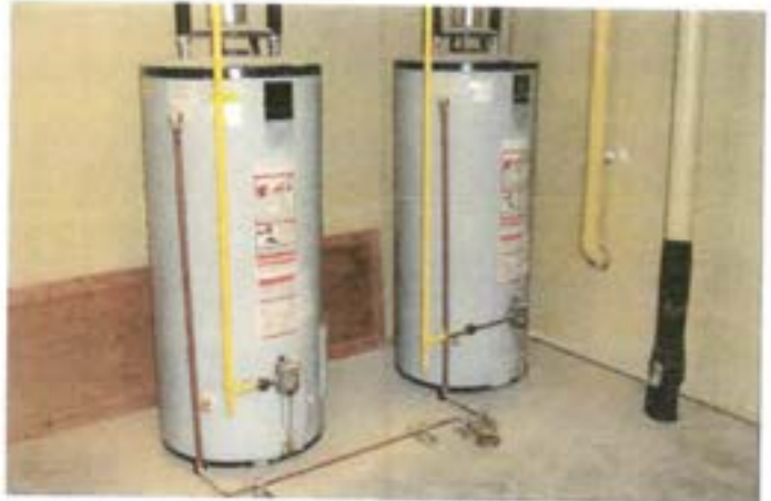
View of the hot water heater located in the HVAC room
