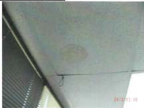
Damaged Ceiling Tiles
