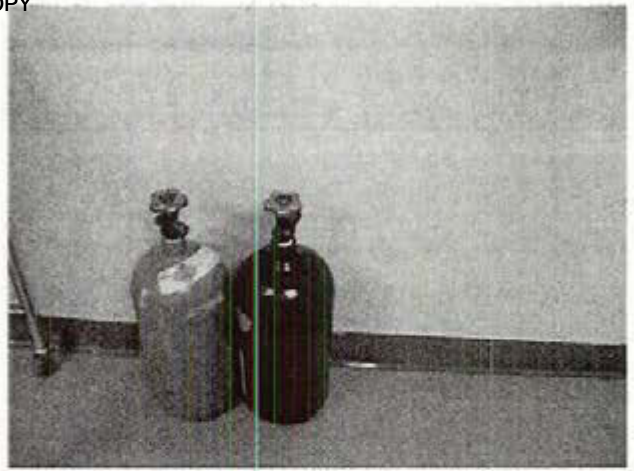
Photograph 26 Safety: unsecured compressed oxygen cylinders
