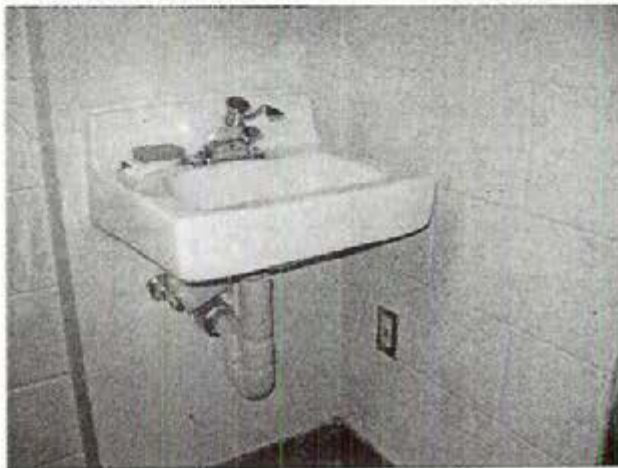
Photograph 27 Safety: GFCI within six feet of a water source did not interrupt the circuit when tested
