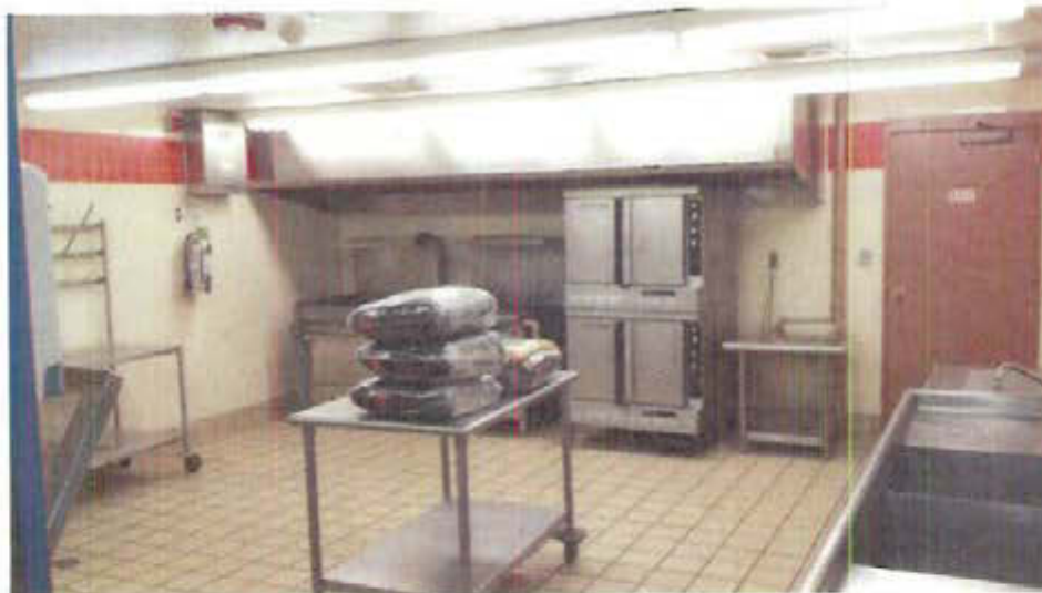
Photo 6: Kitchen with canopy hoods above range and ovens. Ventilation measurements were collected from the three (3) kitchen hoods.
