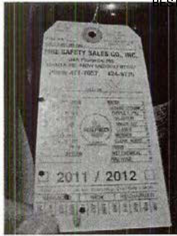
Photograph 25 Safety: fire extinguisher annual inspections were expired
