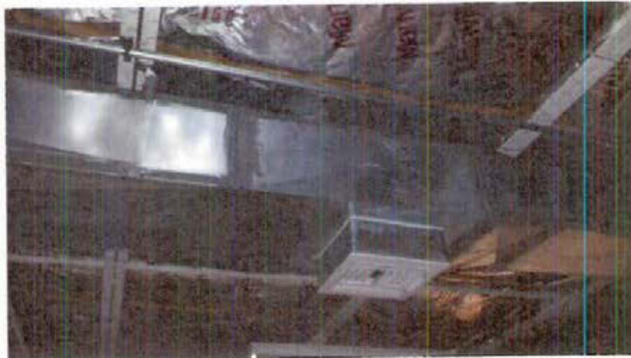
Photo 5: HVAC ducting in the converted IFR. Lead wipe sample 61214-32-G was collected from the top of the HVAC ducting on the west end.
