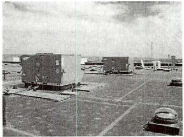
Photograph 22 Packaged combination heating and cooling units on the roof
