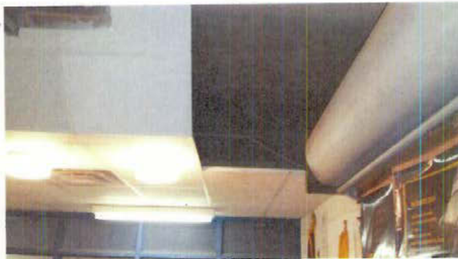
Photo 8: Drop ceiling in the State Guard Office covering the existing IFR concrete shell.
