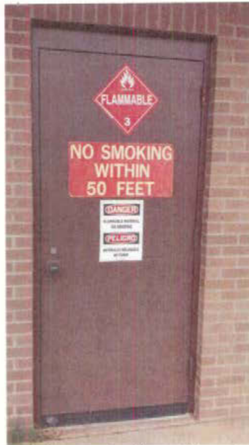
Photo 7: Entrance door to the flammable materials storage room, missing NFPA diamond placarding.
