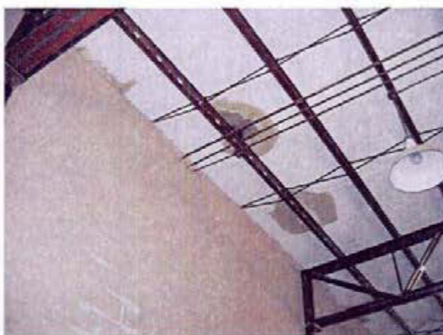
Photograph 6 Severe water damage and mold throughout building
