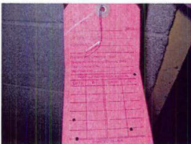
Photograph 5 Fire extinguishers without monthly inspections
