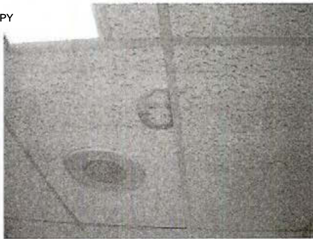
Photograph 8 Stained ceiling tile
