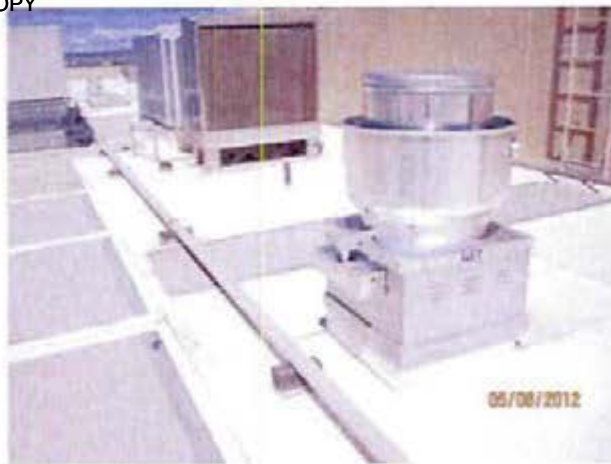
Photograph 20 View kitchen exhaust fan on roof and air conditioning unit, exterior
