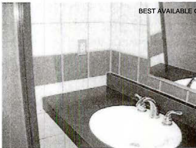
Photograph 7 Non-working GFCI outlet within 6 feet of water supply
