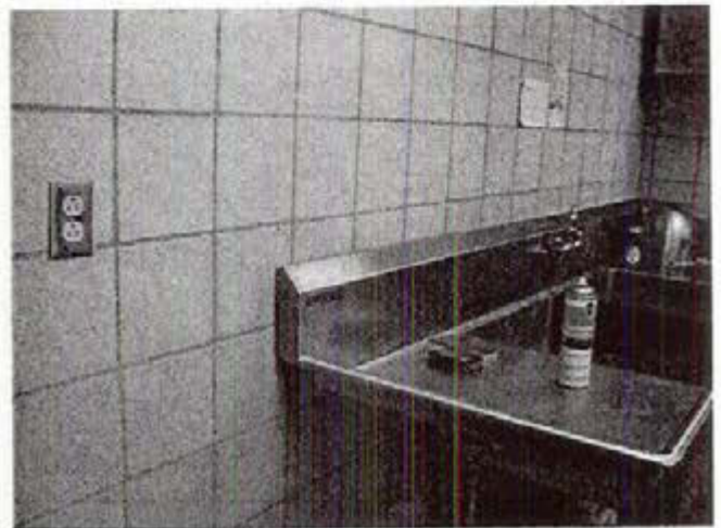
Photograph 10 Safety: No GCFI within 6 feet of a water source.
