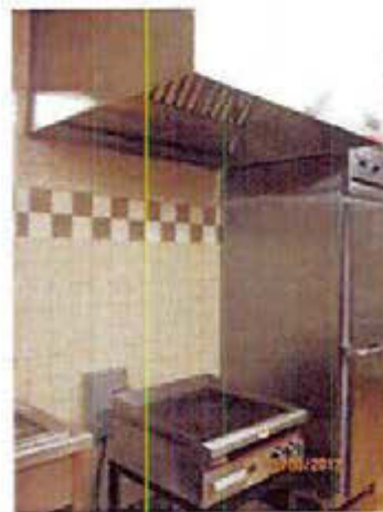
Photograph 22 Kitchen exhaust hood, interior
