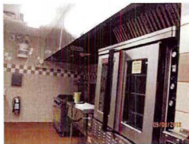
Photograph 23 Kitchen exhaust hood over stove oven, interior
