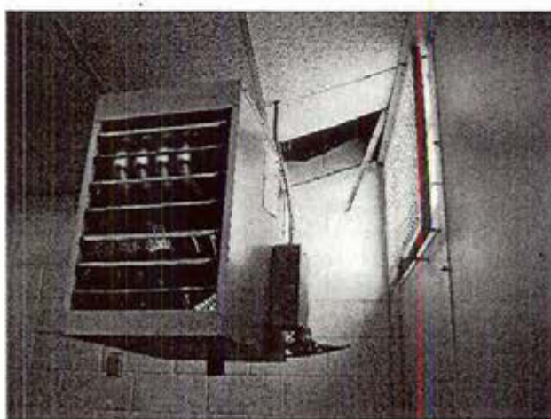
Photograph 16 Natural gas-heating unit, dormitory
