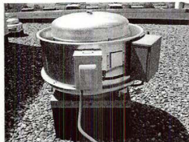
Photograph 6 Stove/oven exhaust duct, exterior
