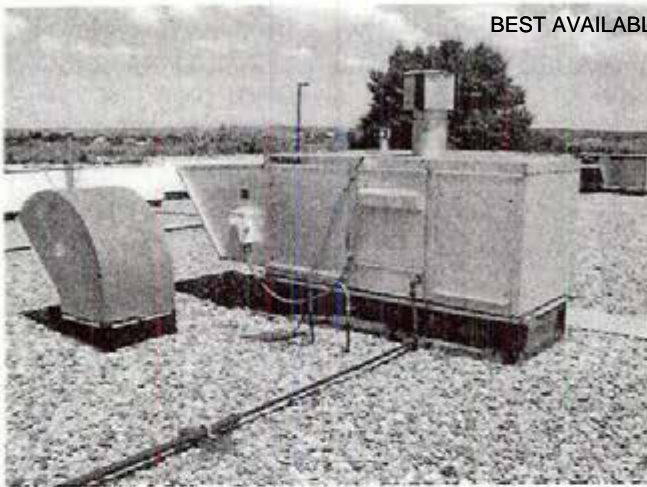
Photograph 7 Air handling unit on roof
