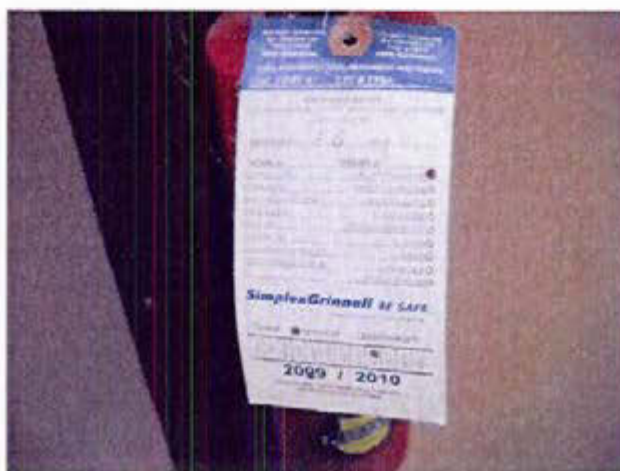
Photograph 4 Firing extinguishers without annual inspections
