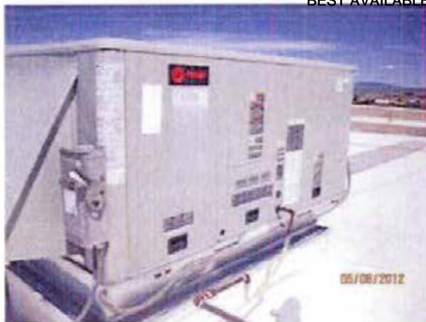
Photograph 19 View of combination heating and cooling packaged HVAC unit, exterior
