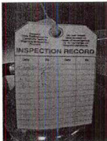
Photograph 9 Safety: monthly and annual fire extinguisher dates not current
