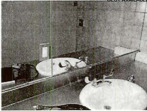
Photograph 19 Safety – GFCI did not function when tested in the women's restroom
