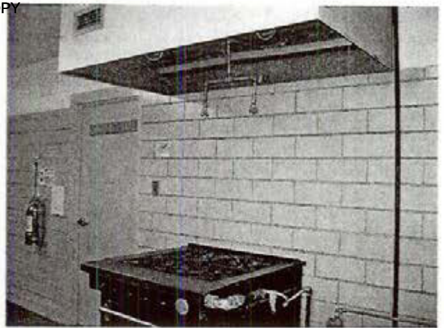
Photograph 20 Kitchen exhaust hood over stove/oven
