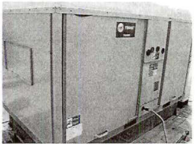
Photograph 22 Combination heating and cooling unit, roof exterior
