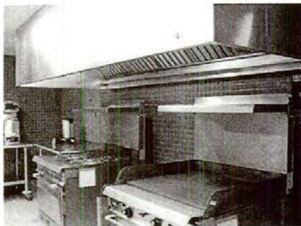
Photograph 23 Kitchen exhaust hood servicing the stove/oven
