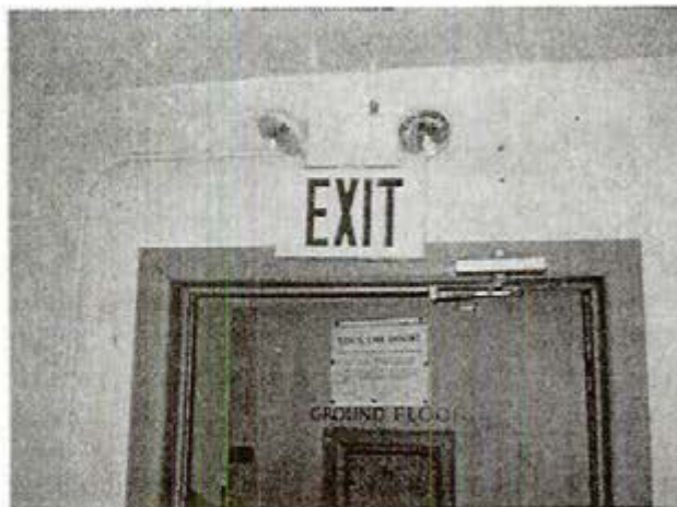
Photograph 17 Safety - Typical emergency exit with emergency lighting that failed to function when tested
