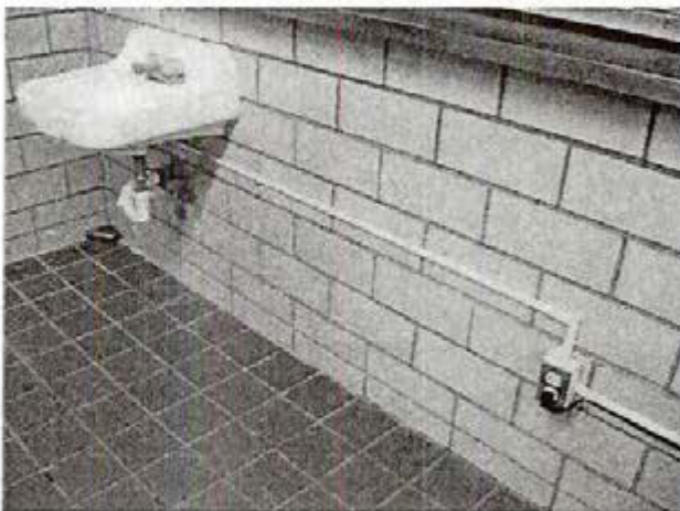
Photograph 29 Safety: Non-functional GFCI within six feet of a water source
