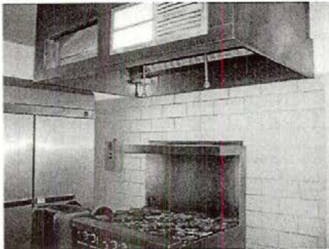
Photograph 15 Kitchen exhaust hood, interior
