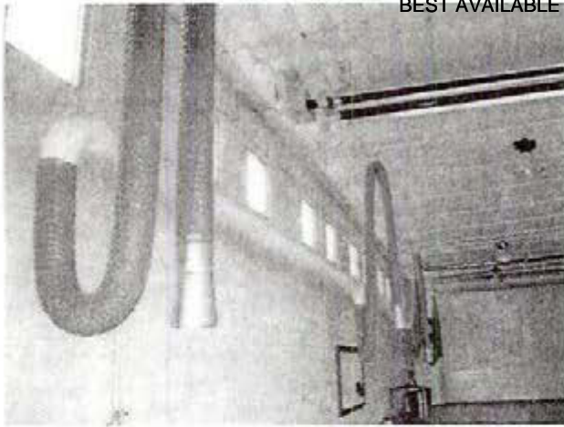
Photograph 13 Ventilation - Drop-Down Tailpipe Exhaust System
