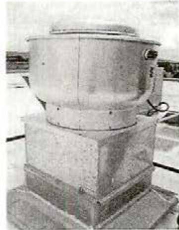
Photograph 24 Exhaust duct for hood servicing the stove/oven
