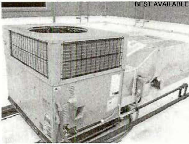
Photograph 27 Package heating and cooling combination unit
