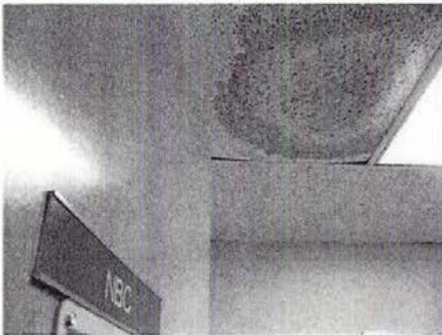
Photograph 21 Water stained ceiling tile in NBC Room
