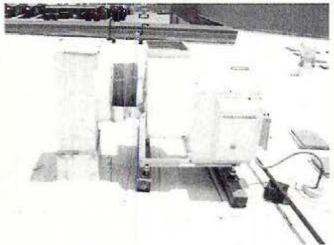
Photograph 16 Roof fan for exhaust hood over stove/oven and food warmer
