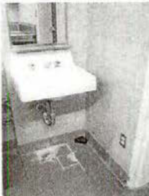
Photograph 17 No GFCI installed within 6 feet of a water source
