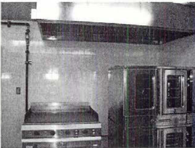
Photograph 15 Kitchen exhaust hood over stove/oven and food warmer
