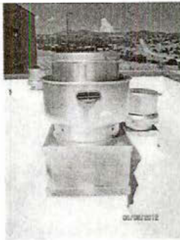
Photograph 15 Roof exhaust fan for kitchen stove/oven
