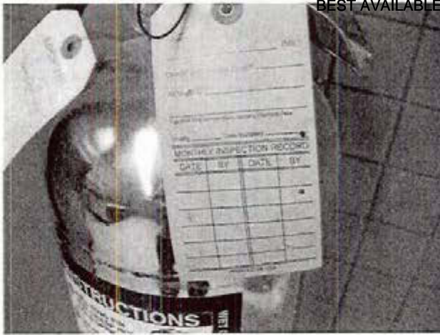
Photograph 13 Fire extinguisher in kitchen without inspections
