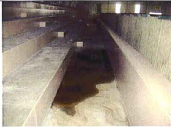
Photo 0021: Drill Hall Bleacher Area – Standing water from roof leak
