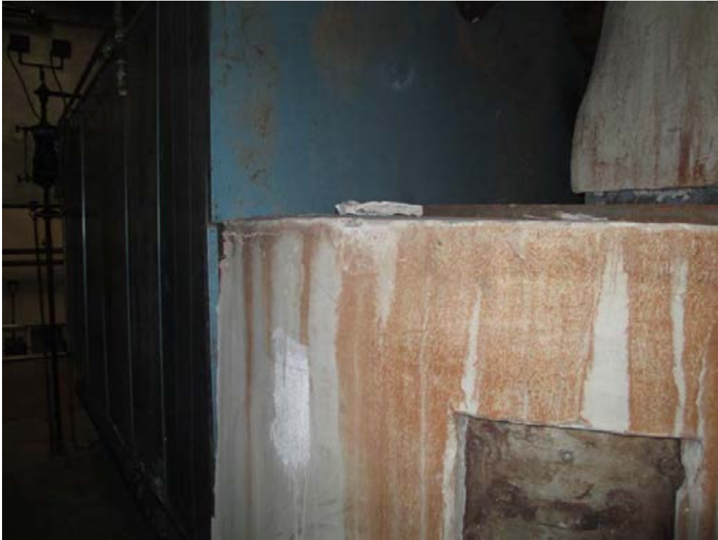
Boiler Room Boiler Breach Suspected ACM
