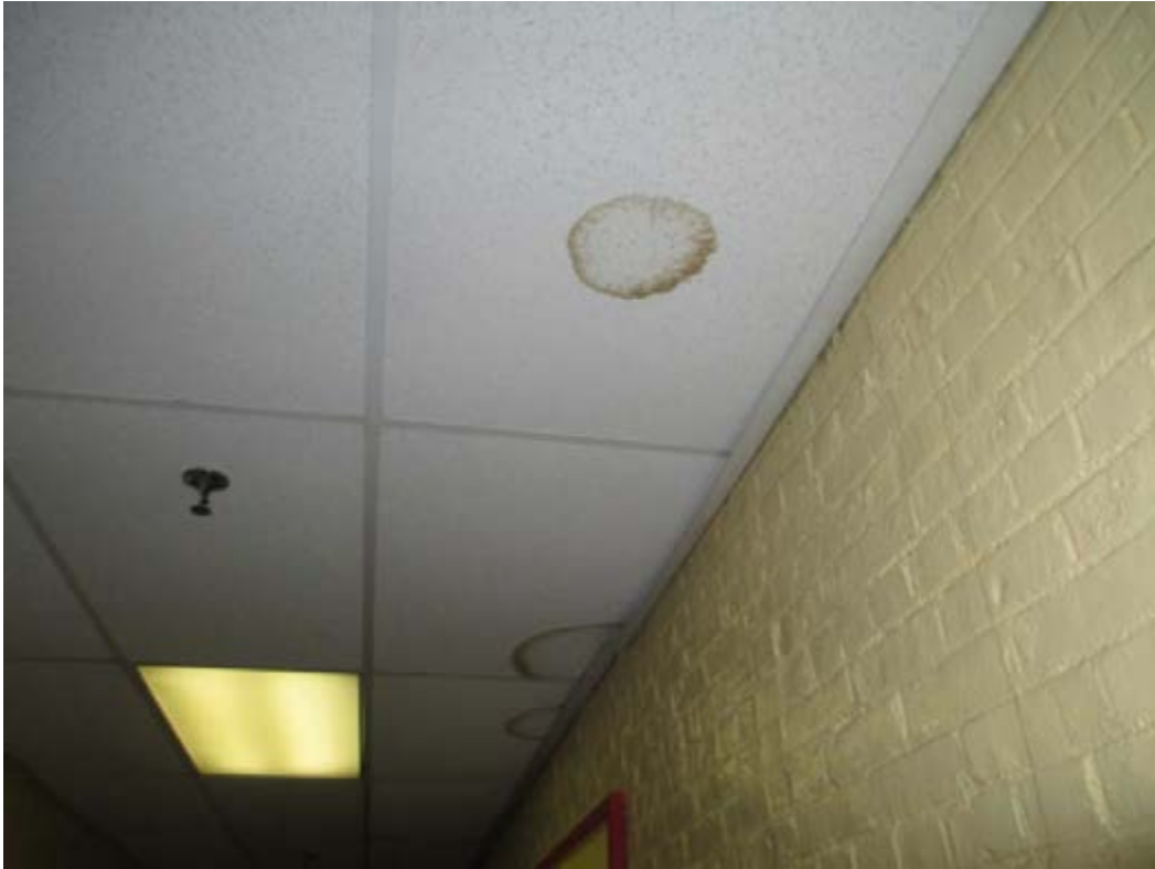
Water Stained Ceiling Tiles
