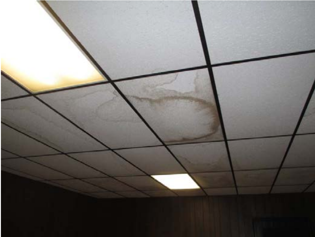
C19 Water stained Ceiling Tiles
