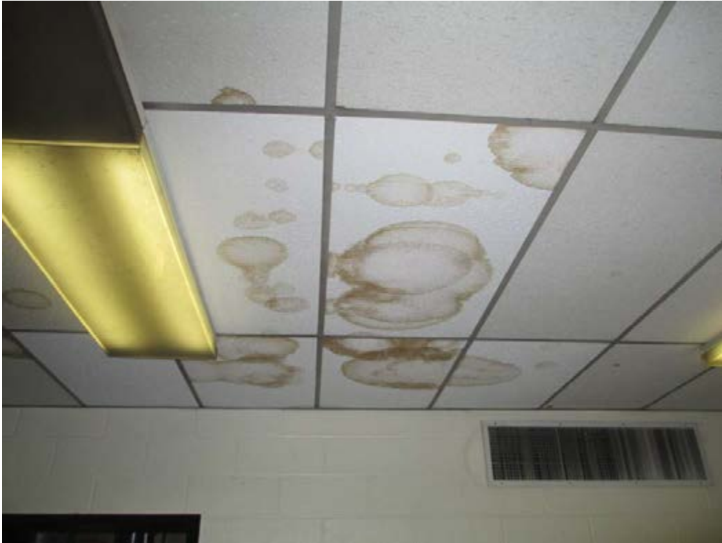
Water Stained Ceiling Tiles
