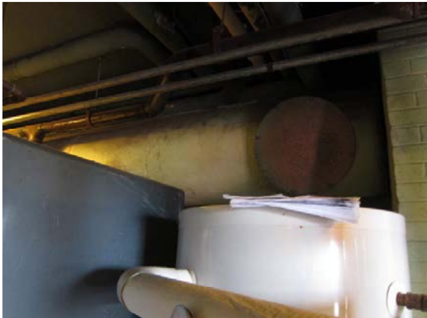
Suspect asbestos boiler breeching in the boiler room
