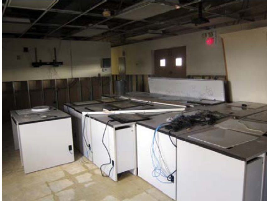
Distributed learning section of the building where the majority of the roof damaged occurred this area is currently not occupied and water is still infiltrating into the building
