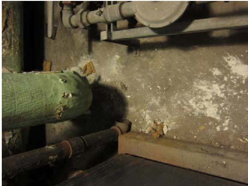
Suspect asbestos mudded joint fitting in poor condition with suspect asbestos debris on the floor in the boiler room
