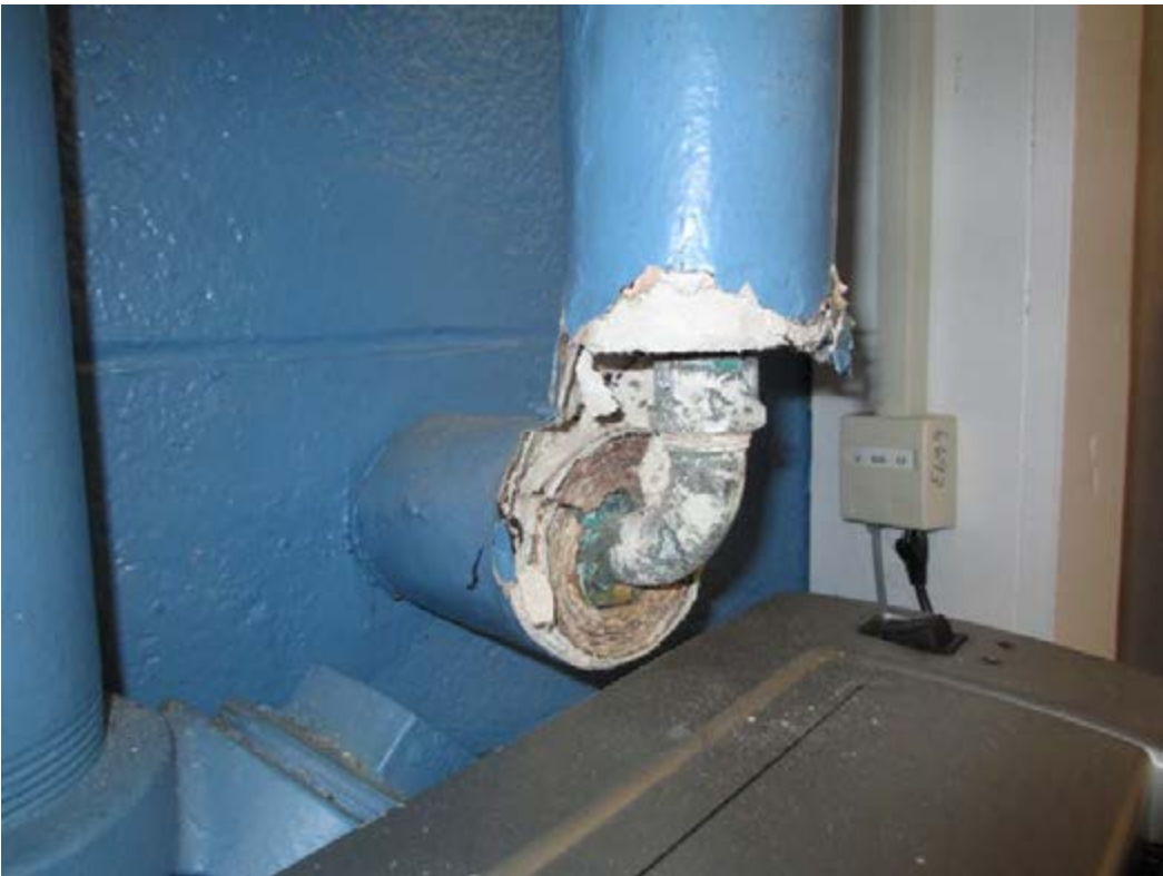
Office 126 Suspected ACM Pipe Insulation
