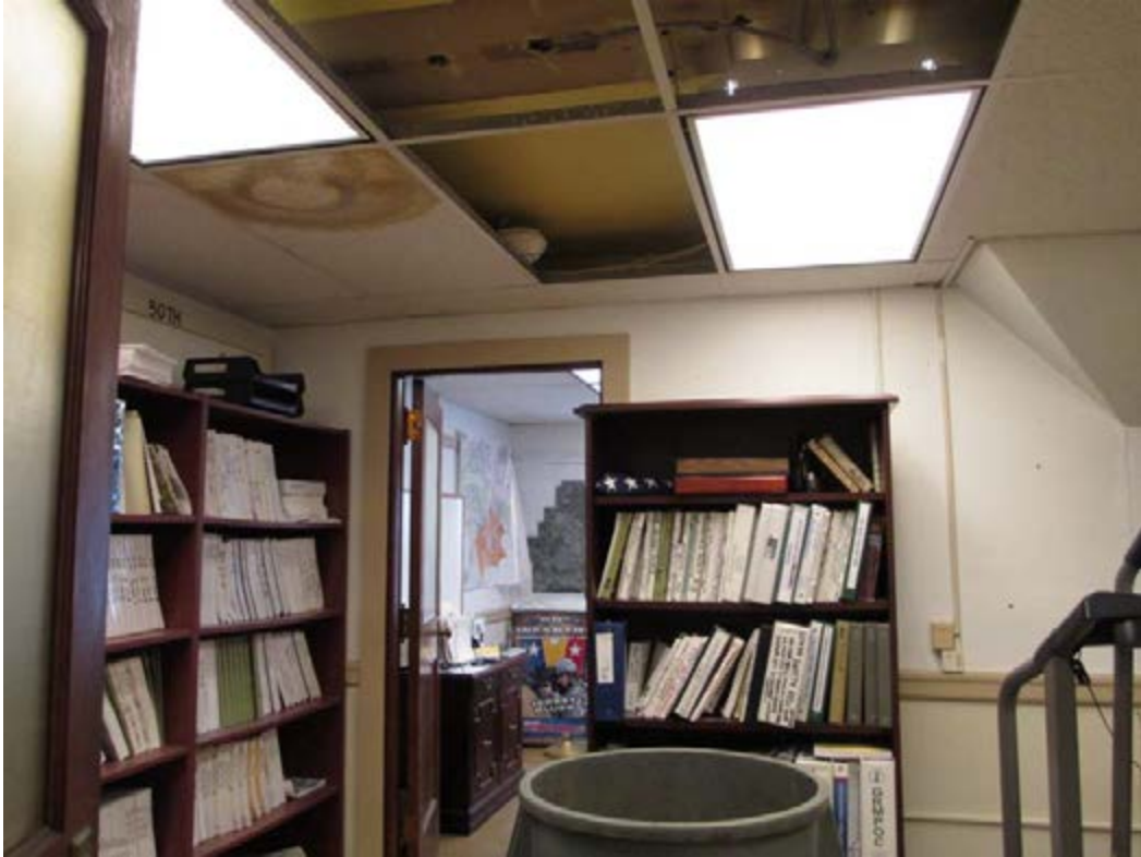
Office 205 Water damage
