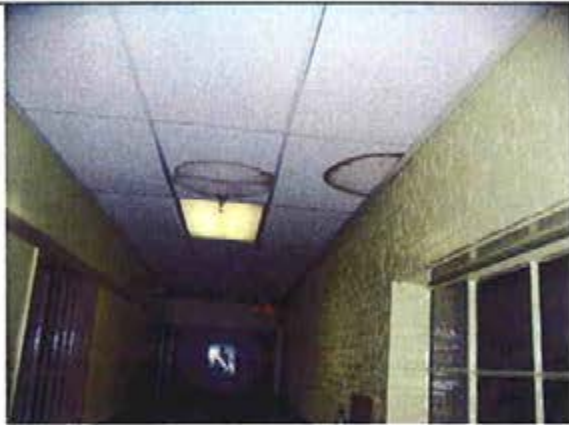
Photo 0018: 2 nd Floor Hall – Water stained ceiling Tiles
