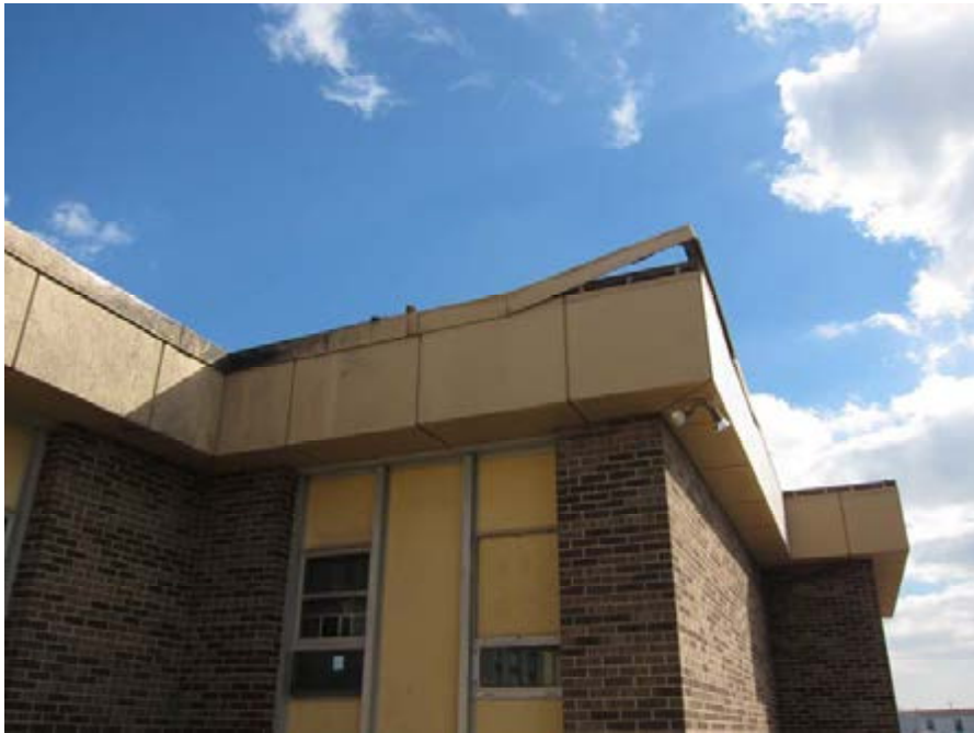
Roof damage sustained by Hurricane Sandy
