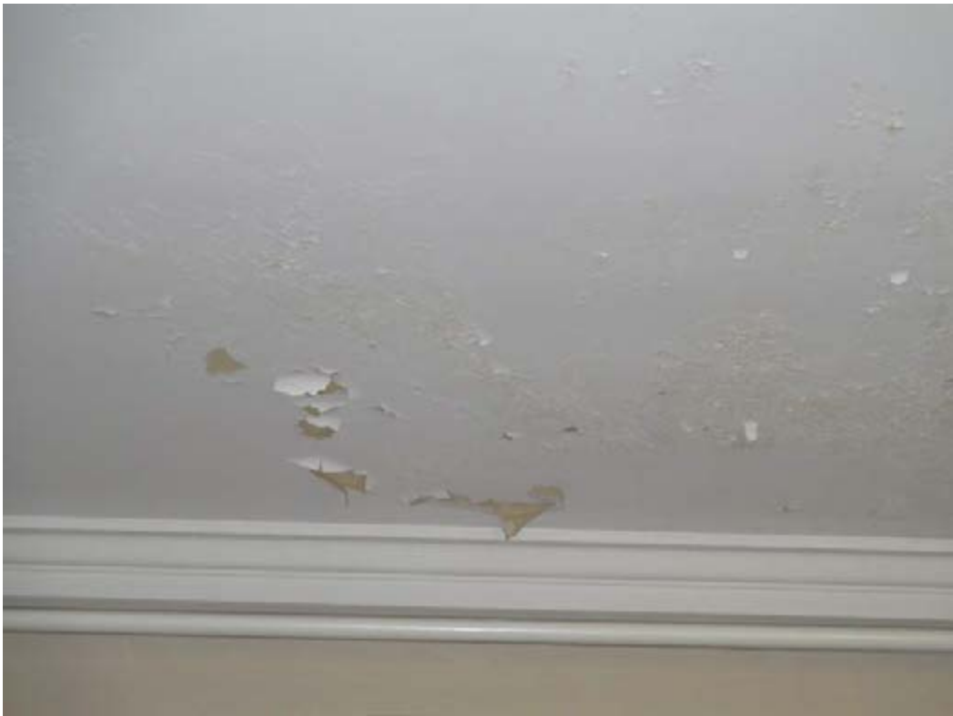
C15 Deteriorated Paint on Ceiling
