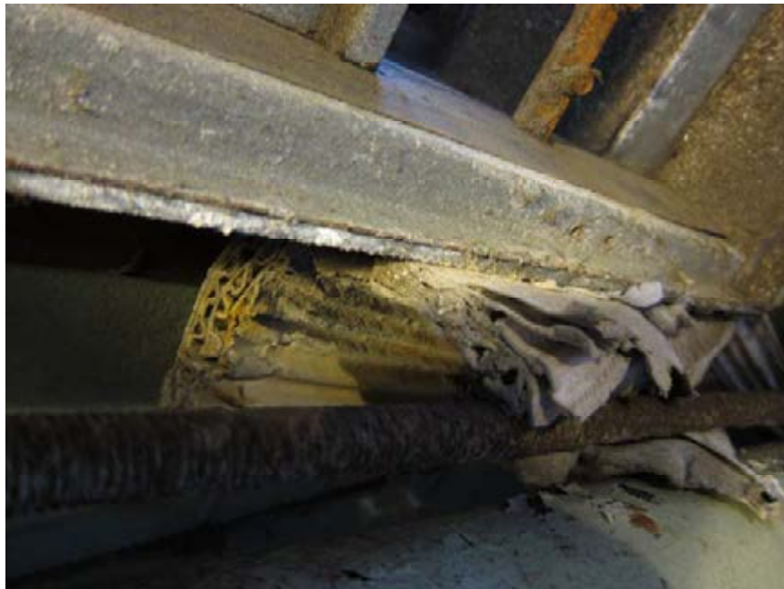
Suspect asbestos pipe insulation in poor condition shoved into a corner in the boiler room
