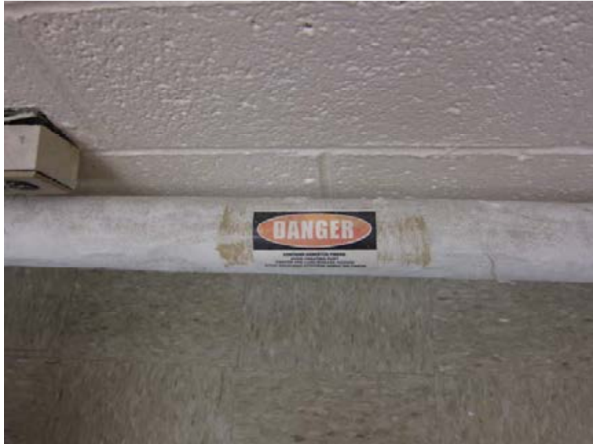
Asbestos pipe insulation and mudded joint fitting, labeled in some areas
