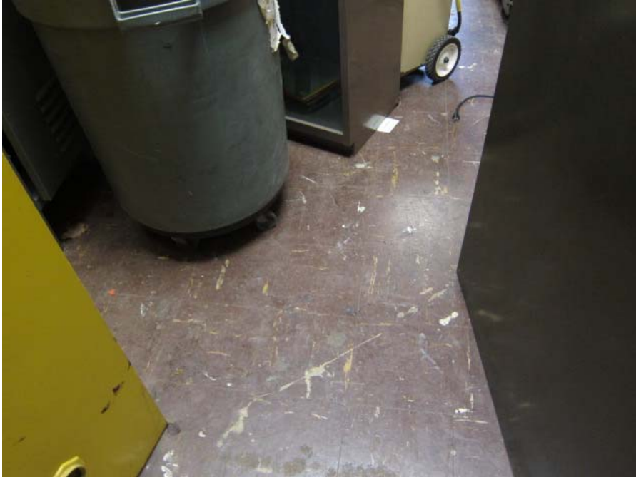
Suspect asbestos 9"X9" brown floor tile
