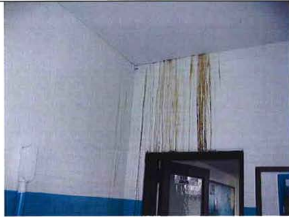
Photo 0742: Foyer – Evidence of a roof leak
