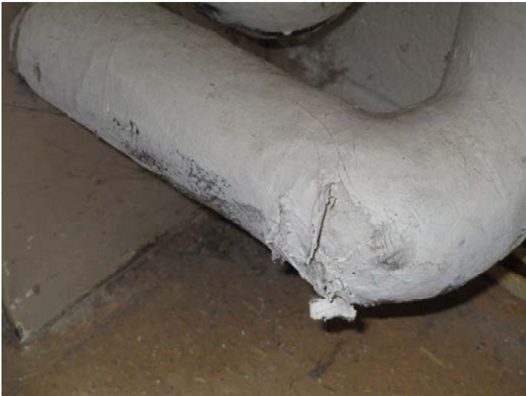
Laundry Hall Suspected Pipe Insulation
