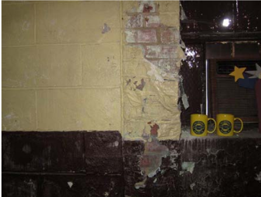
Inside garage number three peeling paint on exterior wall
