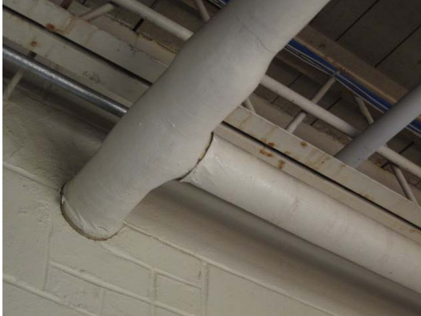
Suspect asbestos pipe insulation and mudded joint fittings
