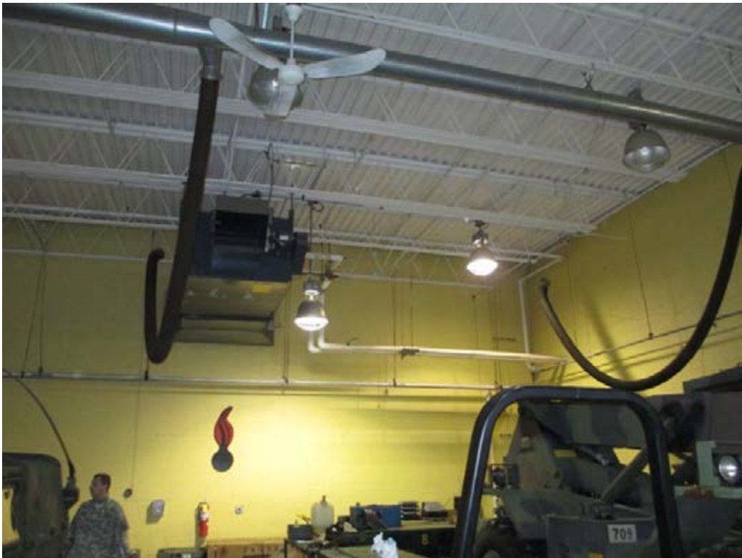
Vehicle Maintenance Exhaust Vents
