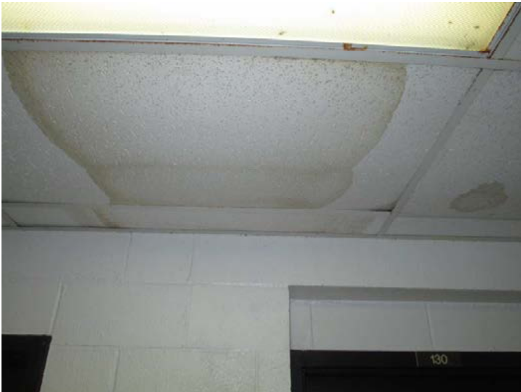
Water Damaged Ceiling Tile at Office 130
