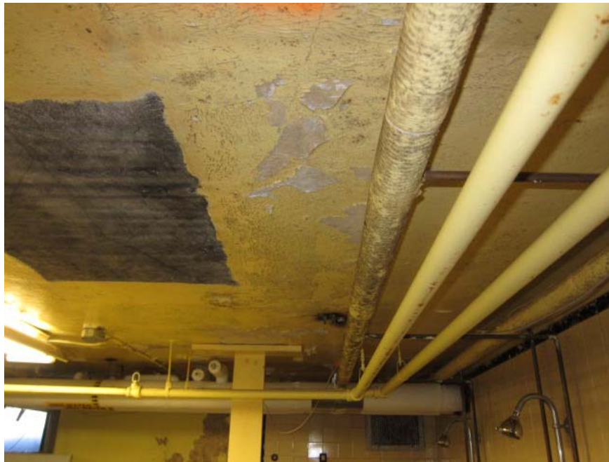
Basement bathroom peeling paint and visible fungal growth
