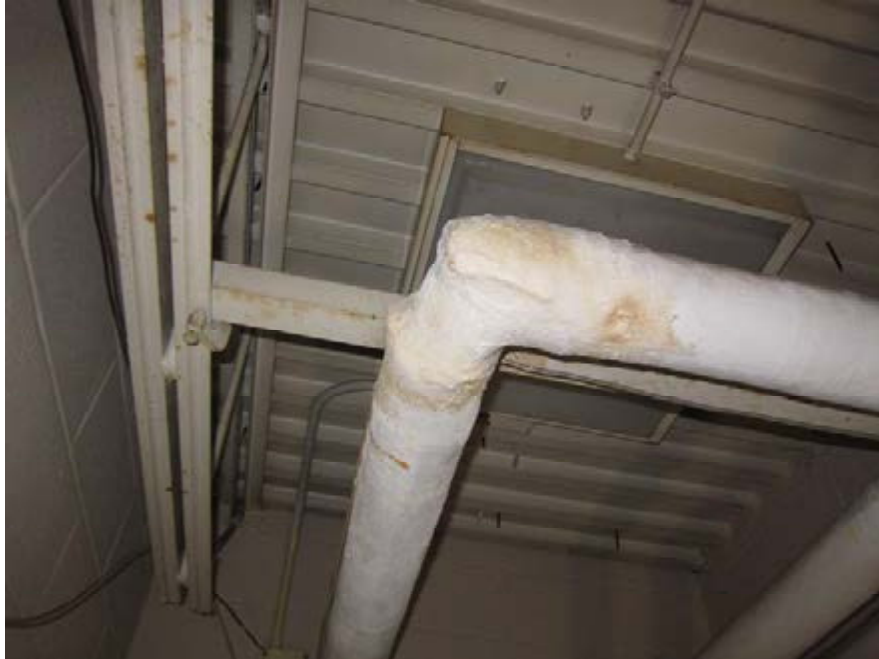
Suspect asbestos mudded joint fittings
