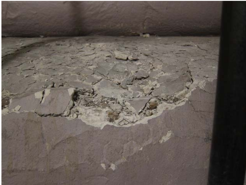
Suspect asbestos friable boiler insulation damaged and in poor condition
