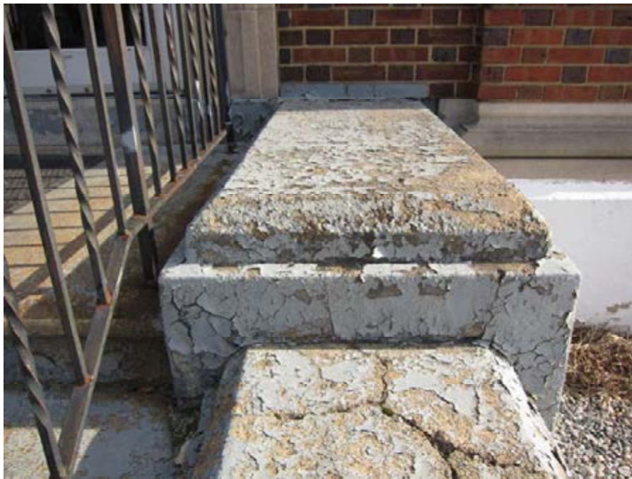
Exterior front steps peeling paint
