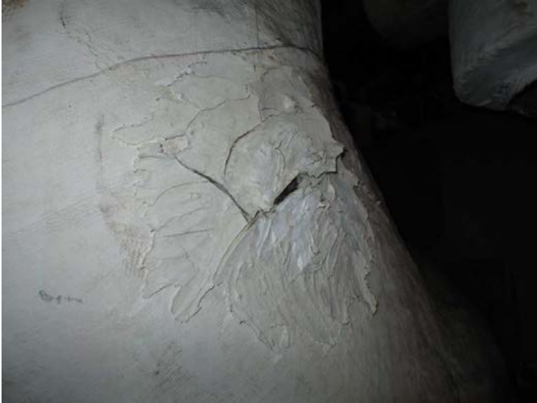
Boiler Room Suspect ACM Patch Material
