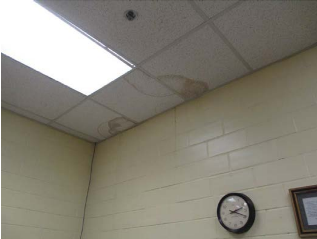
Water Stained Ceiling Tiles
