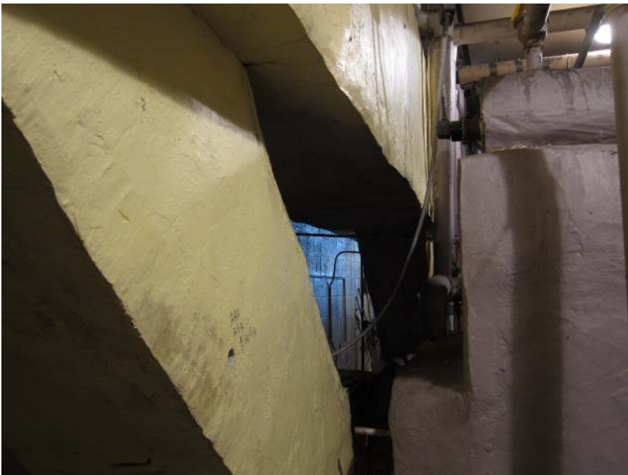
Suspect asbestos boiler breeching insulation
