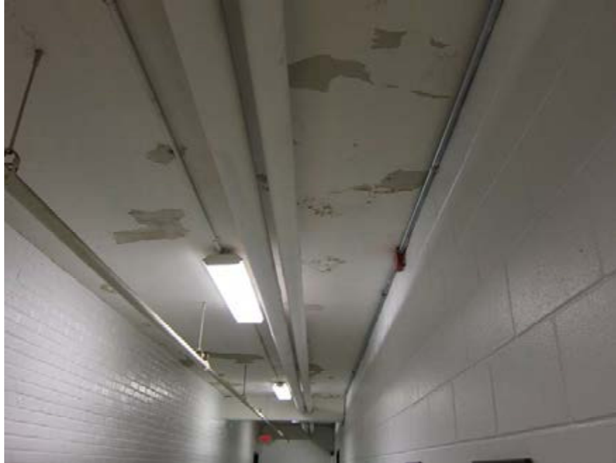
Lower level hallway peeling paint
