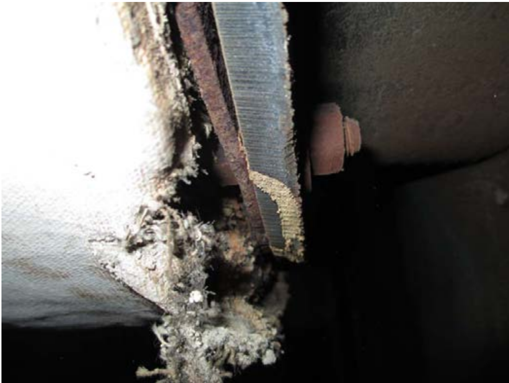
Boiler Room Suspect ACM Pipe Insulation
