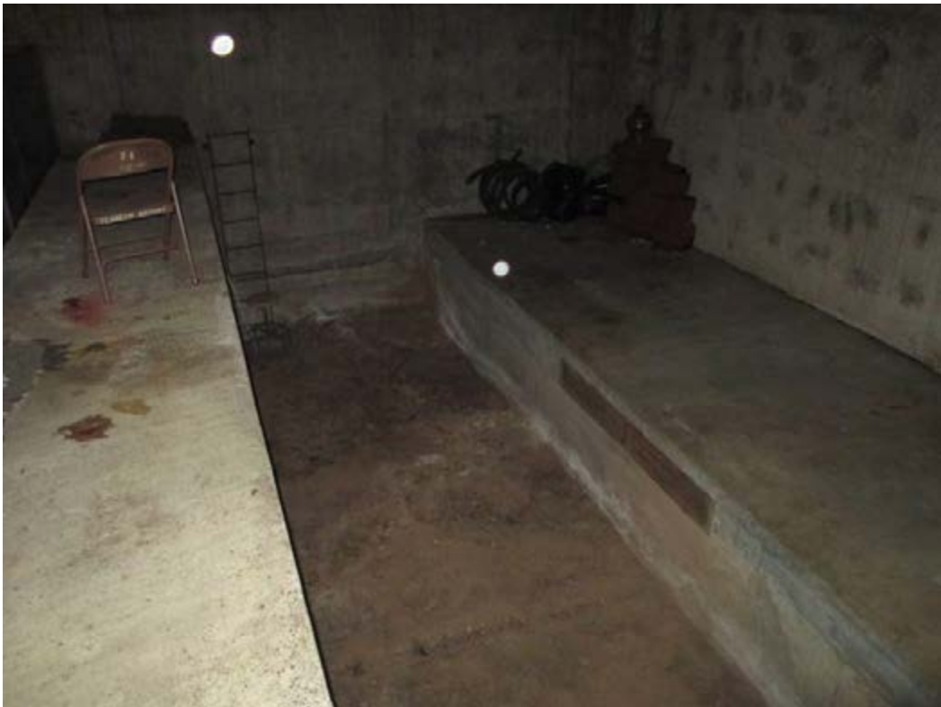
Converted Firing Range Bullet Trap
