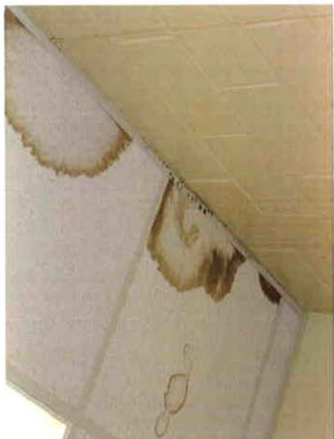
Photo 6: Water Damaged Ceiling Tile
