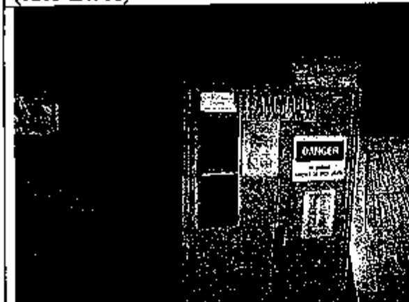
Photo 2879: FDC #9 Flammable cabinet unlocked and fire extinguisher not labeled
