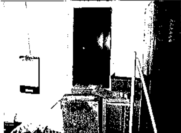
Photo 2989: Janitor room #24 -- Obstructed electrical panel
