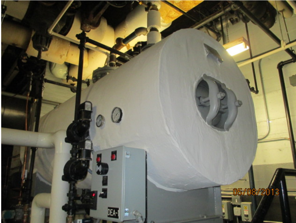
Boiler Insulation Suspect ACM
