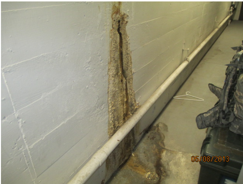
Converted Firing Range Water Infiltration
