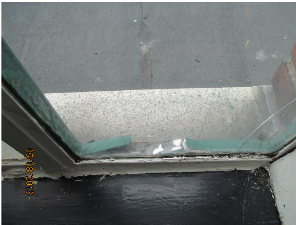
3 rd Floor Conference Window Glazing Suspect ACM
