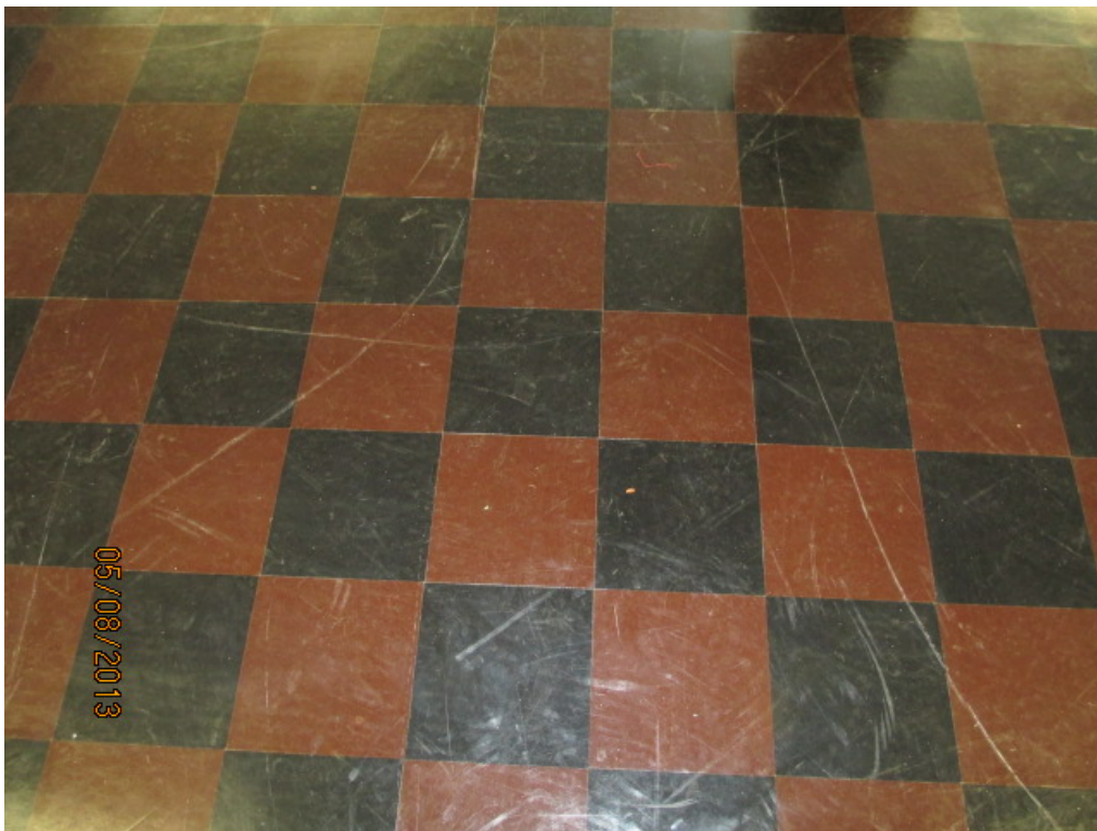
9"x9" Floor Tile Suspect ACM
