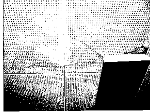
Photo2954: Office #18 - Water stained ceiling tiles
