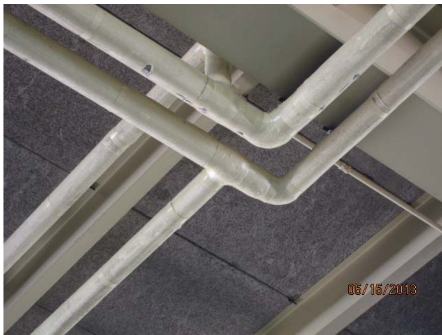
Suspect asbestos pipe insulation and muddled joint fittings
