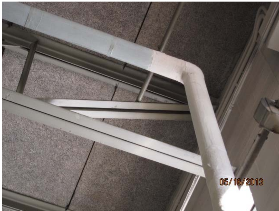
Suspect asbestos pipe insulation and muddled joint fittings in the drill hall
