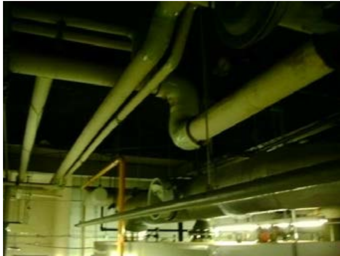
Fiberglass Insulation in Boiler Room
