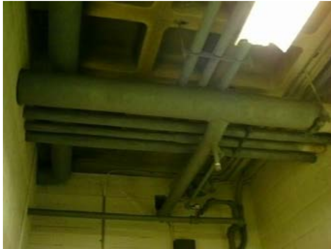
Typical ACM Pipe Insulation
