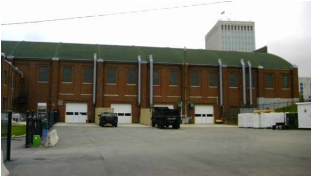
Building Exterior – Rear – Note LEV exhaust ducts venting at roof level
