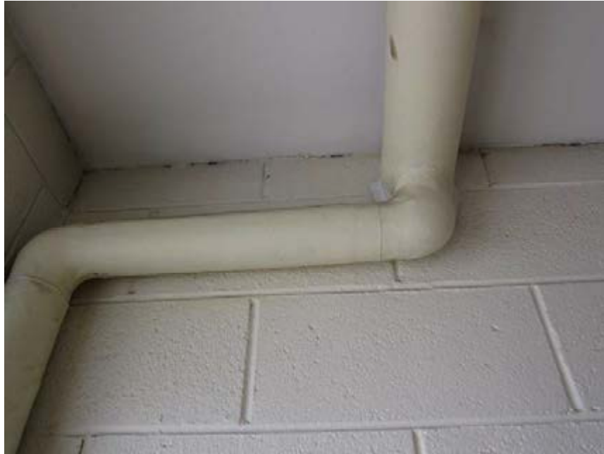
Suspect mudded joint fittings throughout the facility
