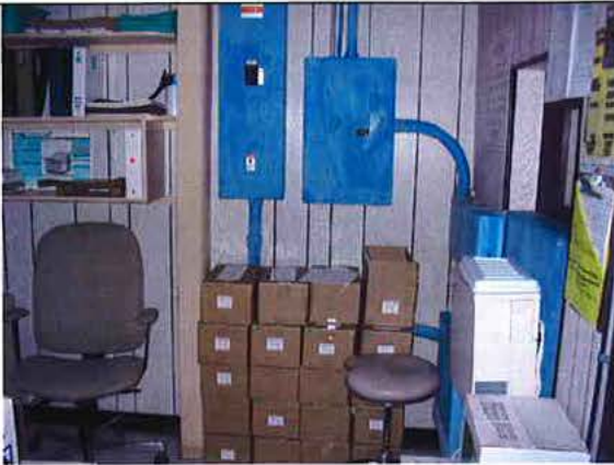
Photo 740: X-Ray Processing- Obstructed Electrical Panel
