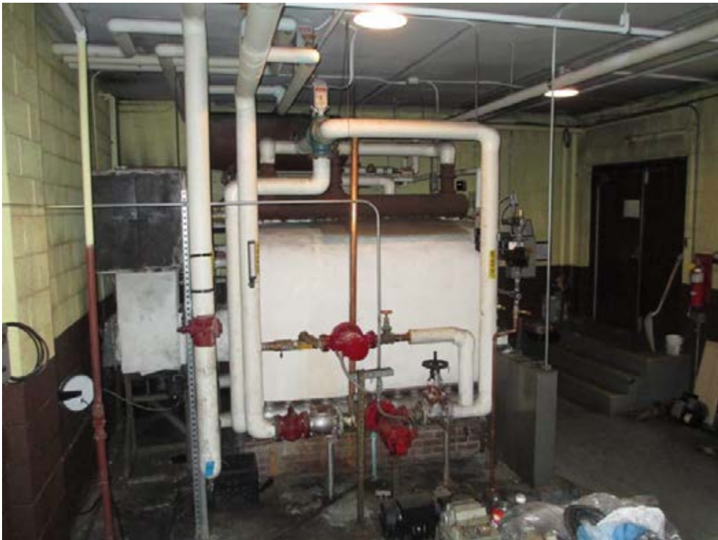
Suspect ACM Boiler Breech Material
