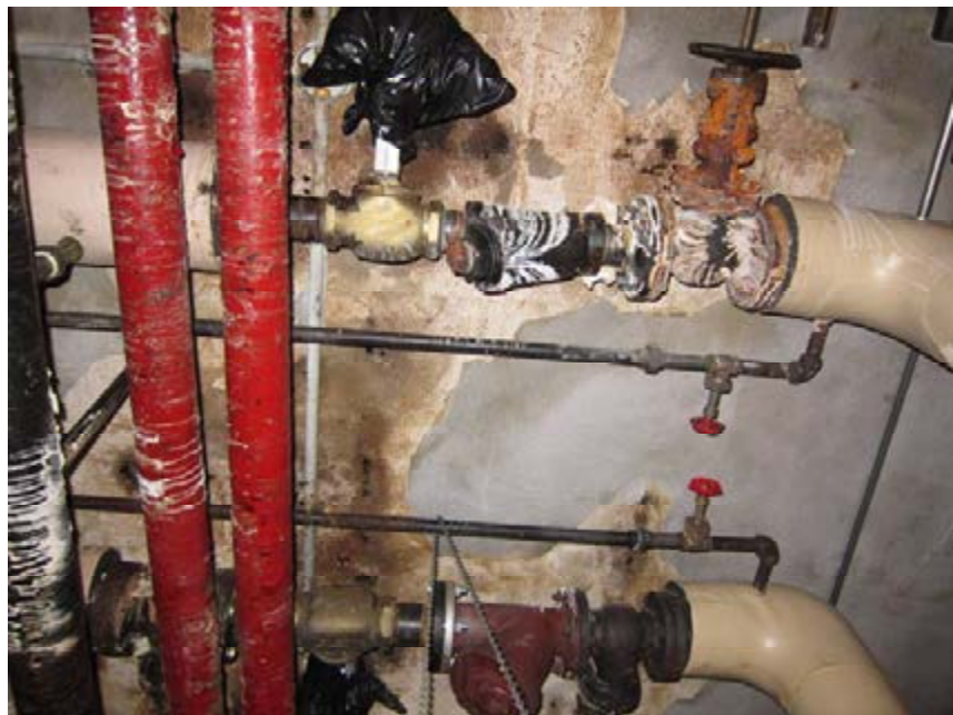
Boiler room water damage from roof leaks
