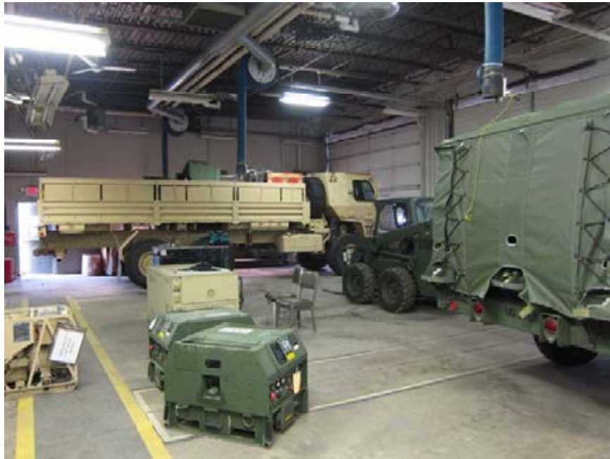
Inside detached garage/storage with overhead vehicle exhaust system
