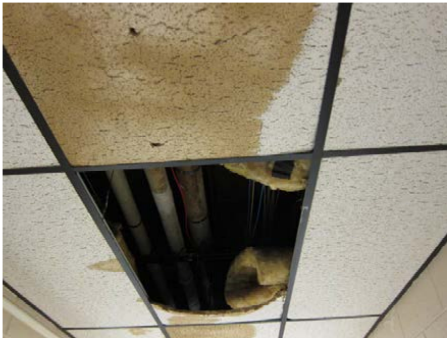
Main hallway water damage from roof leaks and suspect asbestos pipe insulation above ceiling tiles
