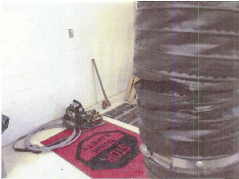
Photo 7: Tear in North Exhaust Vent.
