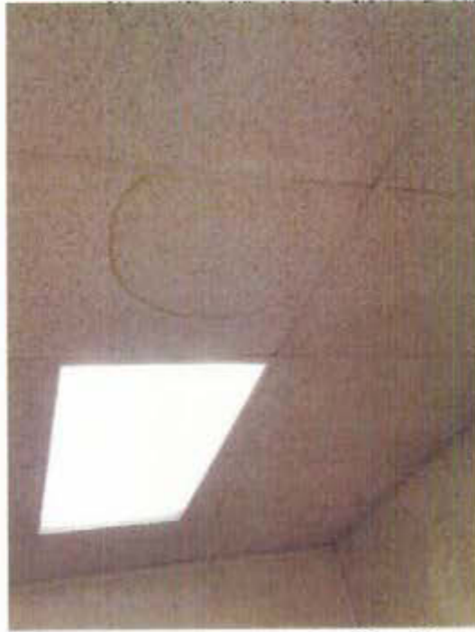
Photo 11: Water stained ceiling tiles.
