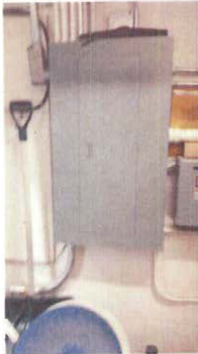
Photo 13: Breaker panel located in mechanical room; blocked by buckets on floor.
