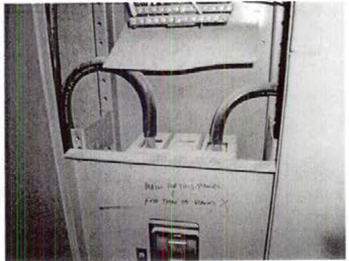
Photo 14: Supply Room #4; close-up view of exposed wires in breaker panel on East wall.
