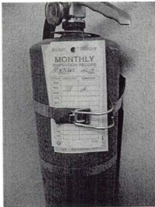
Photo 5: Fire extinguisher in locker room with outdated inspection tag; dated February 2014.
