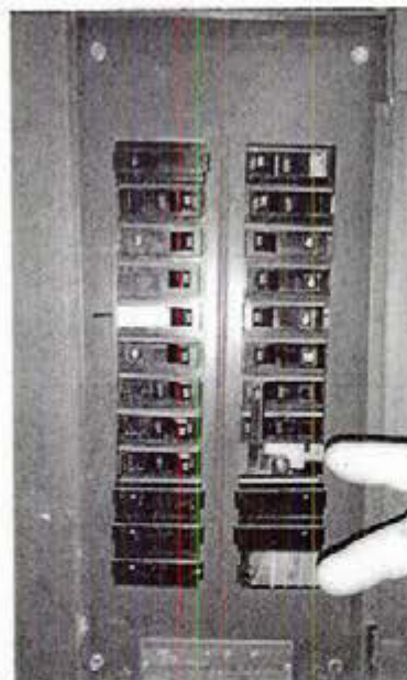
Photo 12: Supply Room #4; close-up view of exposed conductors in breaker panel.
