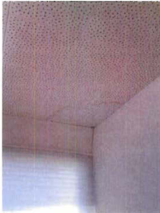
Photo 11: Water damaged ceiling tiles in PSG office, 1'x1' ceiling tiles are suspected to have asbestos containing mastic.
