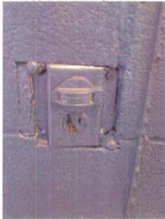
Photo 5: Damaged electrical outlet located on the western wall of the drill floor.
