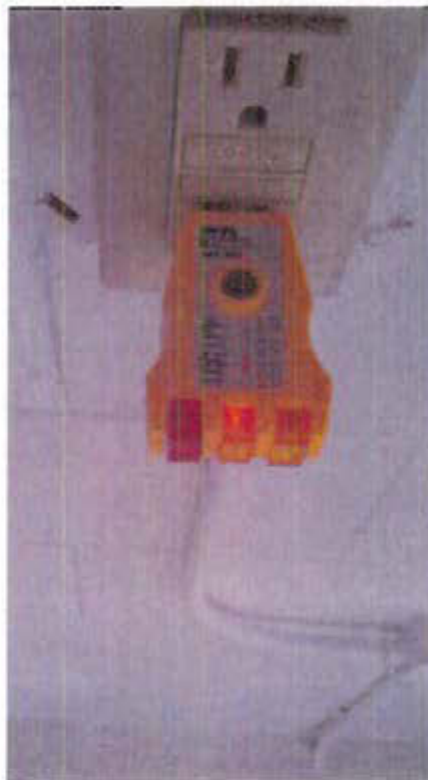
Photo 10: GFCI tester indicates "Open Ground" in Supply Closet (labeled LAV).
