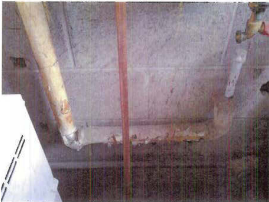
Photo 21: Bulk asbestos sample 81513-HMLTIARM-Bulk 2 collected from hot water pipe insulation.
