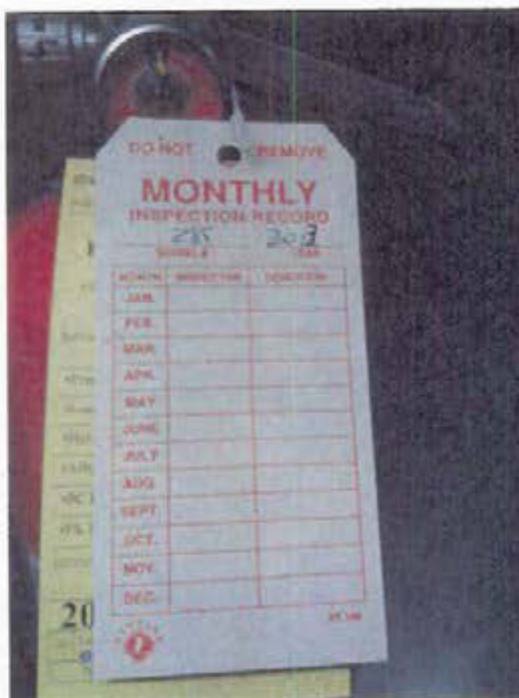
Photo 10: Fire extinguisher with expired monthly inspection tag.
