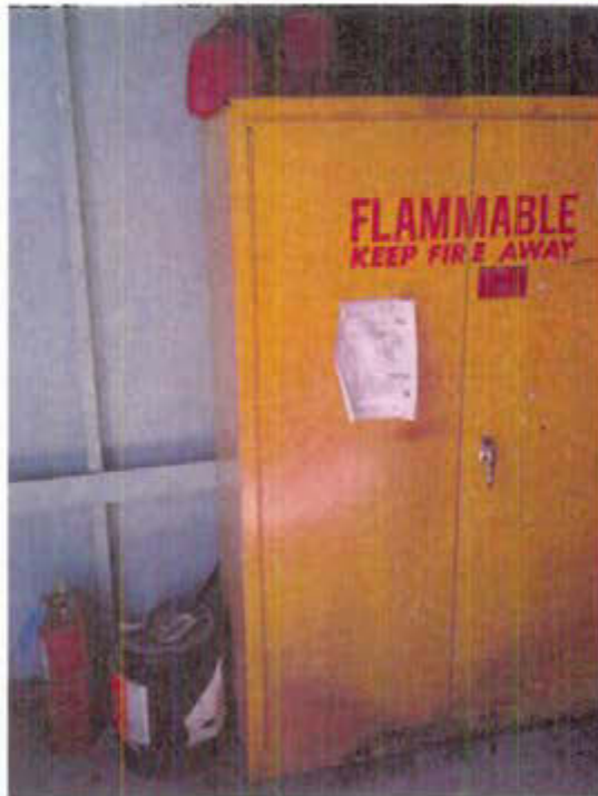
Photo 7: Flame cabinet in POL shed, self-closing feature non-operational, fuel stored on top of cabinet.
