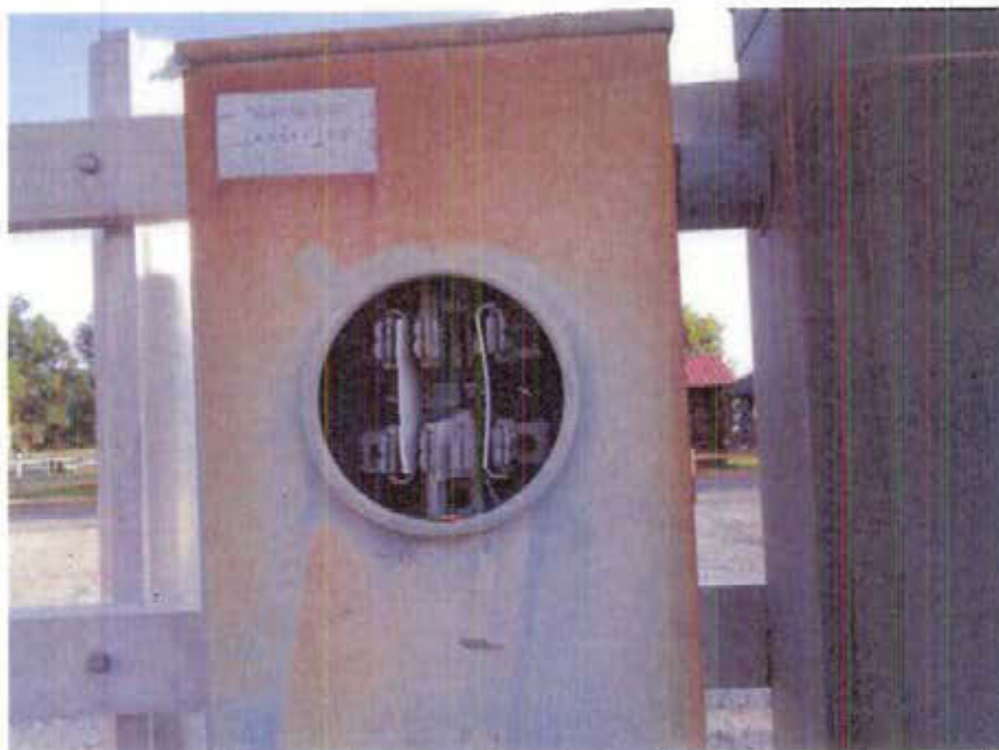
Photo 4: Electrical box missing meter panel, possible access to live conductors.
