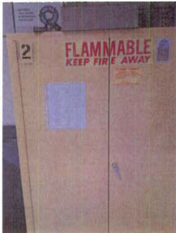
Photo 6: Flame cabinet in Supply room, self-closing feature non-operational.
