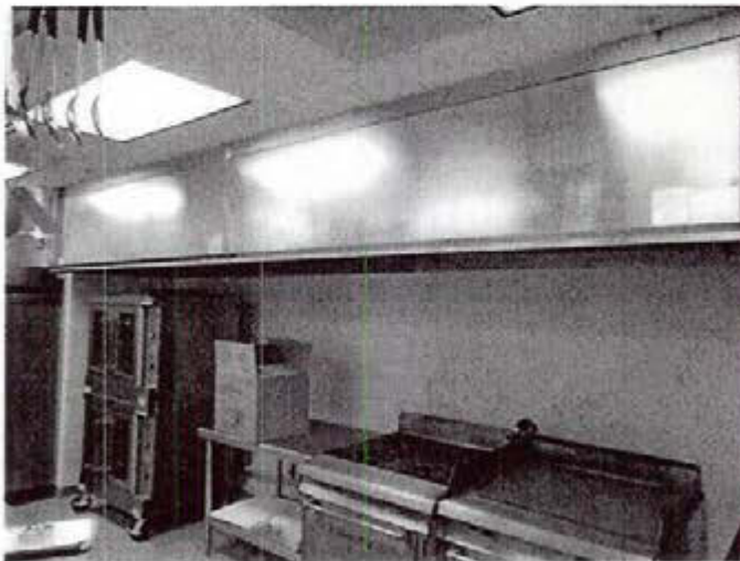
Photo 17: Non-operational kitchen canopy hood over range.
