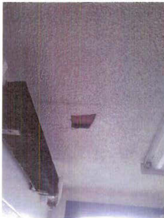
Photo 22: Bulk asbestos sample 81513-HMLTIARM-Bulk 3 and Bulk 4 collected from ceiling in the supply closet (labeled LAV). Bulk 3 acoustic material - Bulk 4 transite board.
