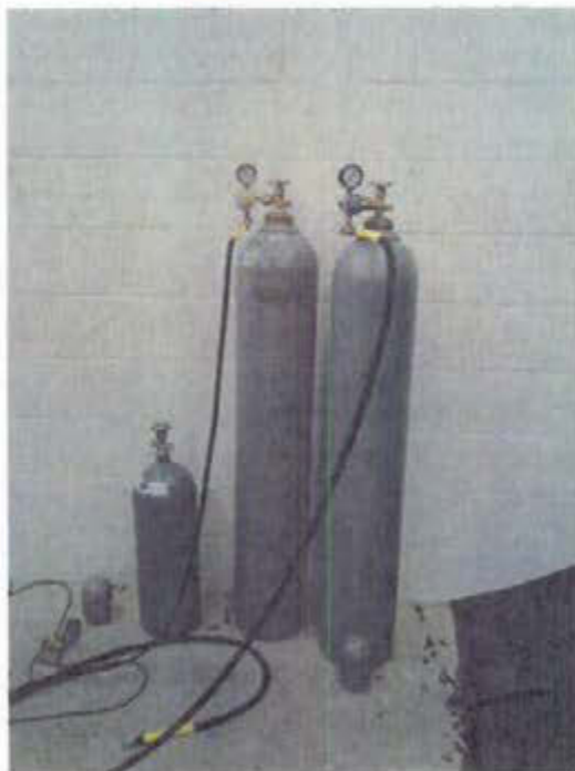
Photo 9: Unsecure CO 2 cylinders located near bullet trap. No safety collars are used while cylinders are not in use. One cylinder was left open.
