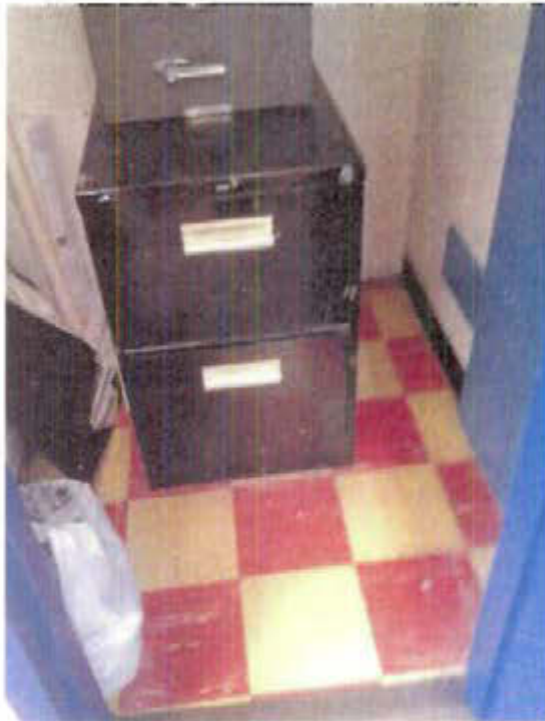
Photo 12: 9"x9" floor tiles are suspected to be asbestos containing material.
