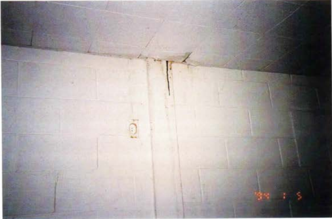
Water Damage located on the Ceiling inside of Classrooms
