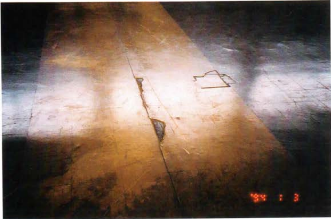
Views of Cracked and Broken Floor Tiles Puddle Located in the Armory Drill Hall
