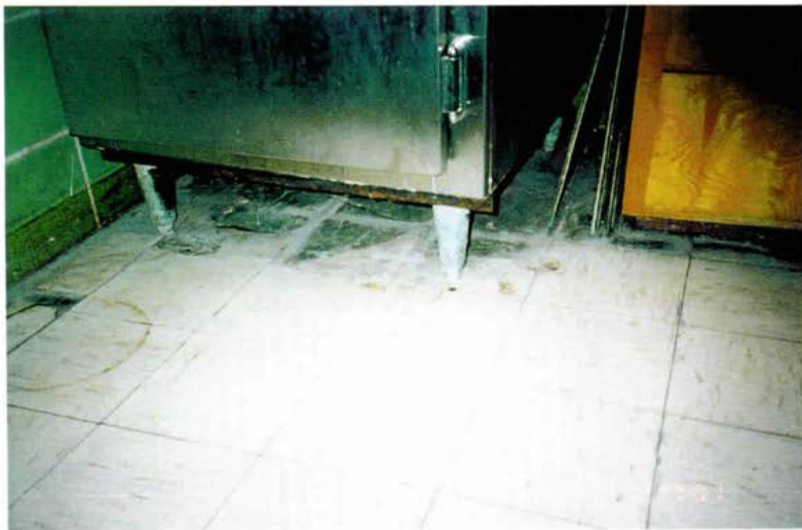
Damaged/Missing Floor Tile in the Kitchen/Mess
