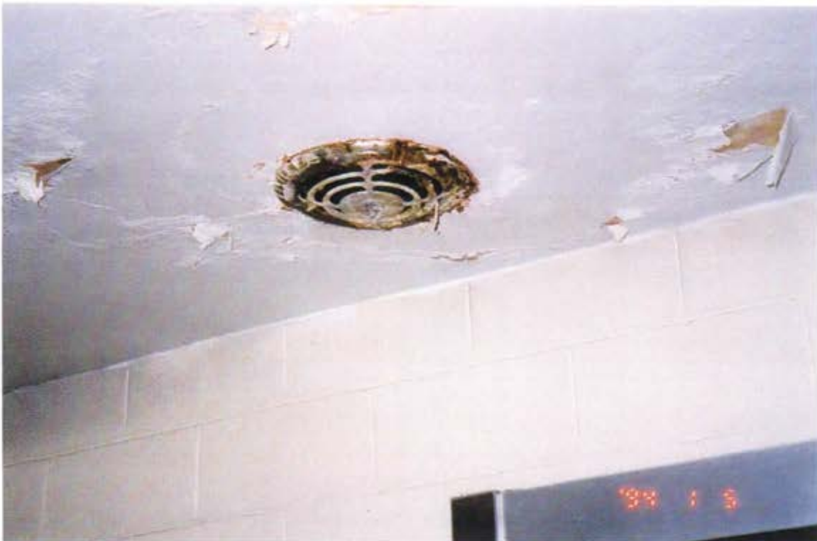
Water Damage Around Exhaust Vent in Mess Kitchen
