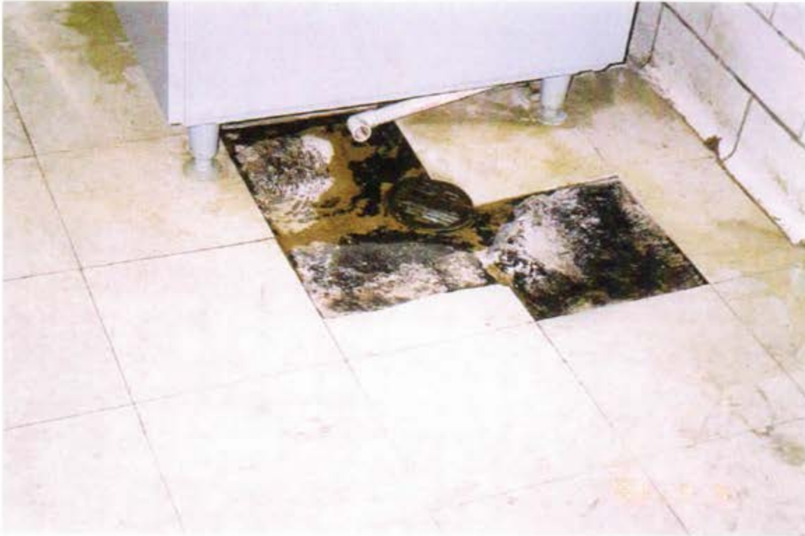
Missing Floor Tiles in Mess Kitchen
