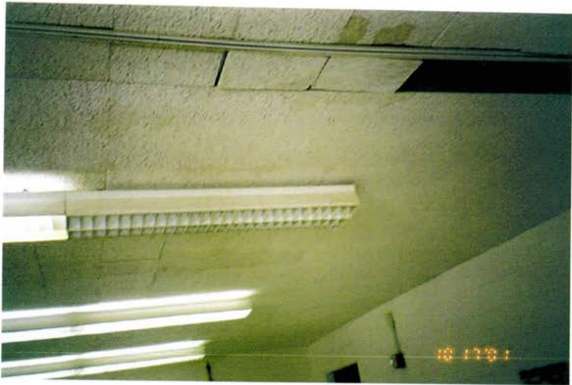
Views of Damage Ceiling Tiles In the Classroom
