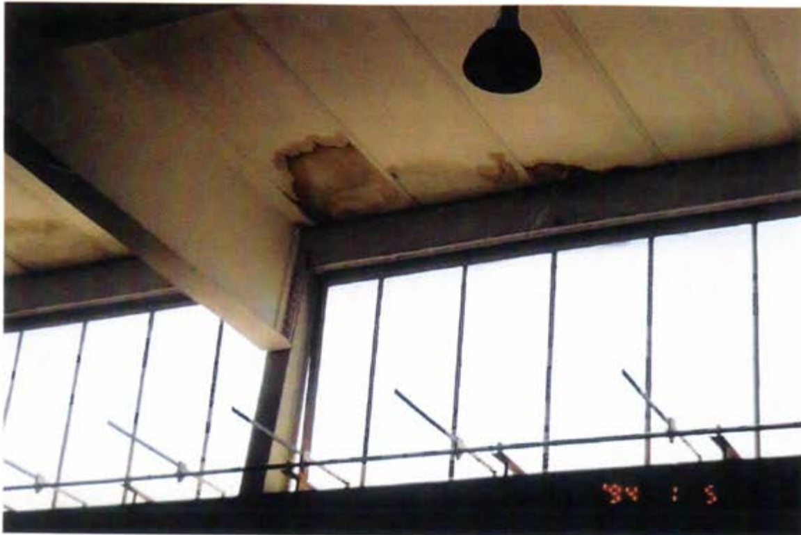
Views of Water Damage of Ceiling in Drill Hall
