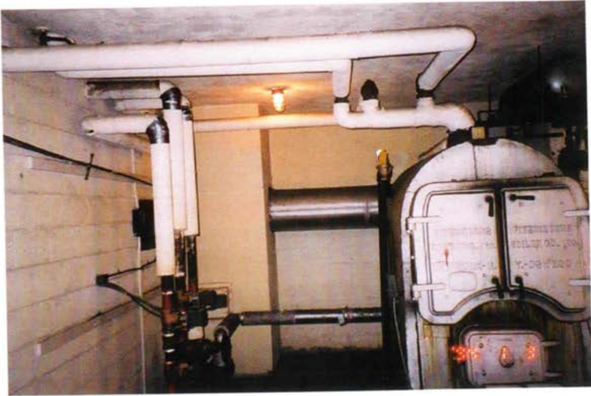
Views of ACM on Boiler and Pipes
