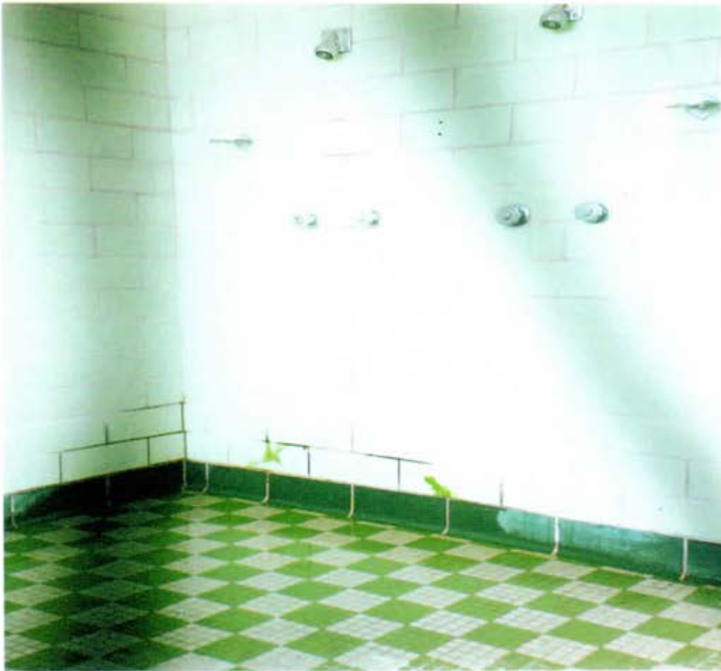
View of green Mold along bottom of wall in the Shower at the Smithfield NG Armory
