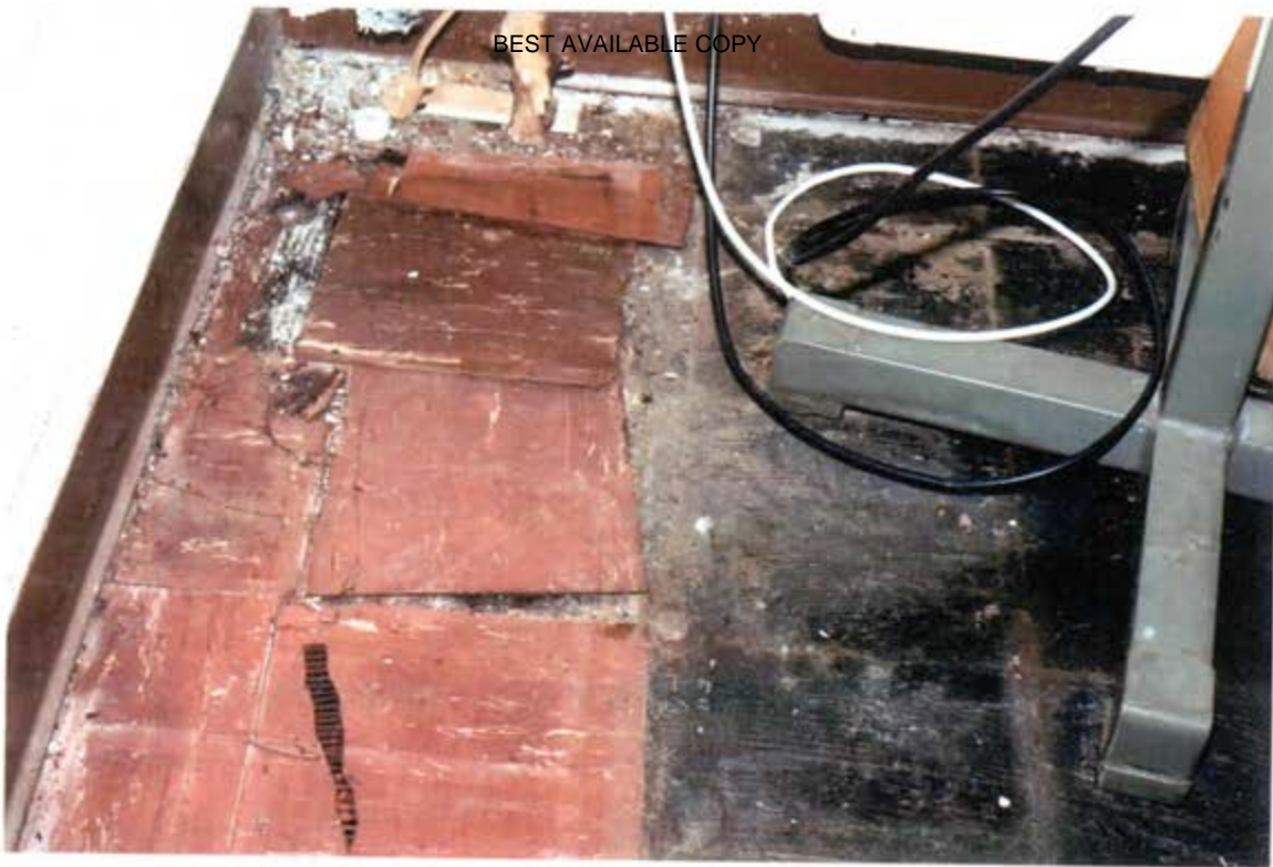
882nd Office Broken Floor Tiles
