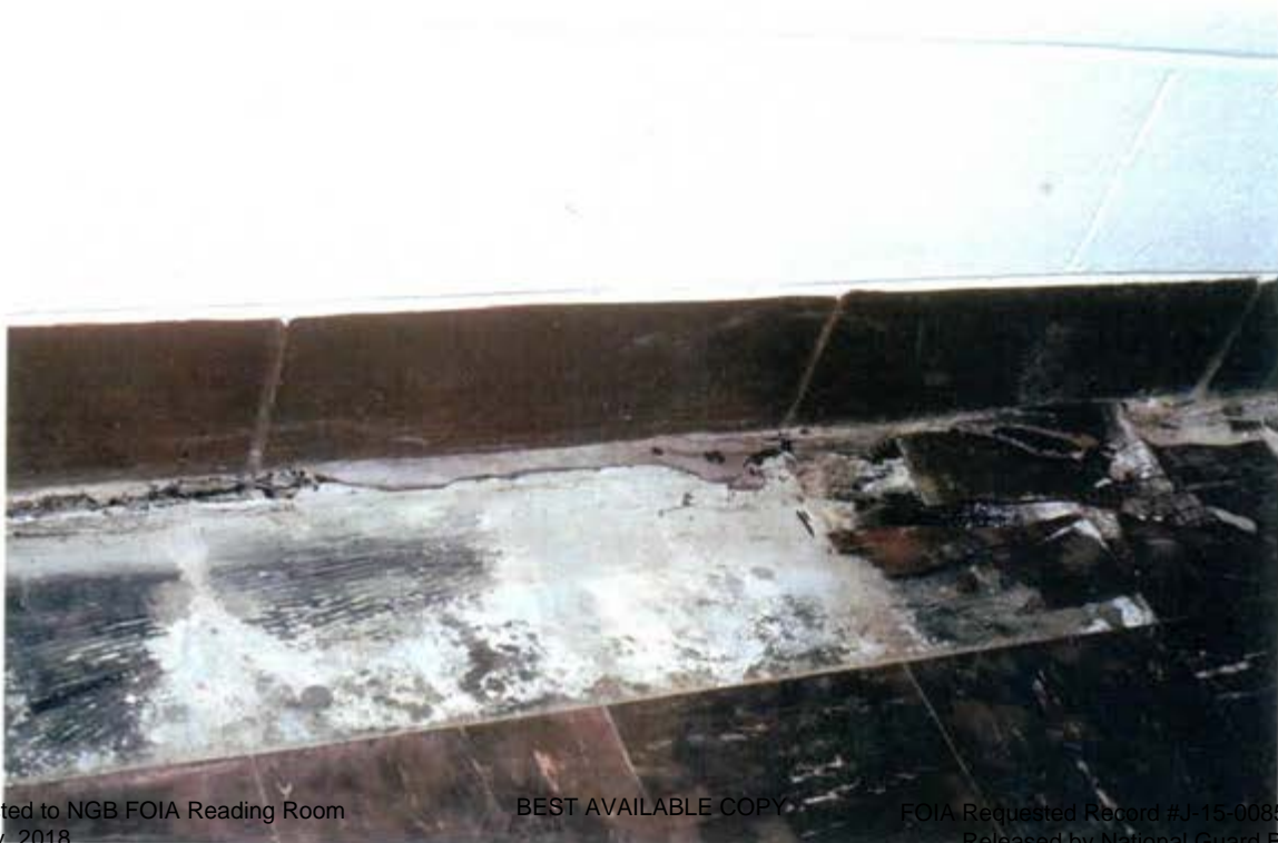
Weight Room Broken & Missing Floor Tiles
