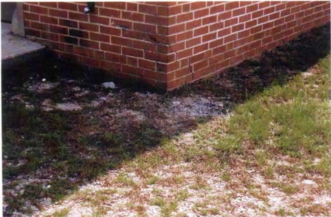
Views Exterior Foundation and Brick Water Damage
