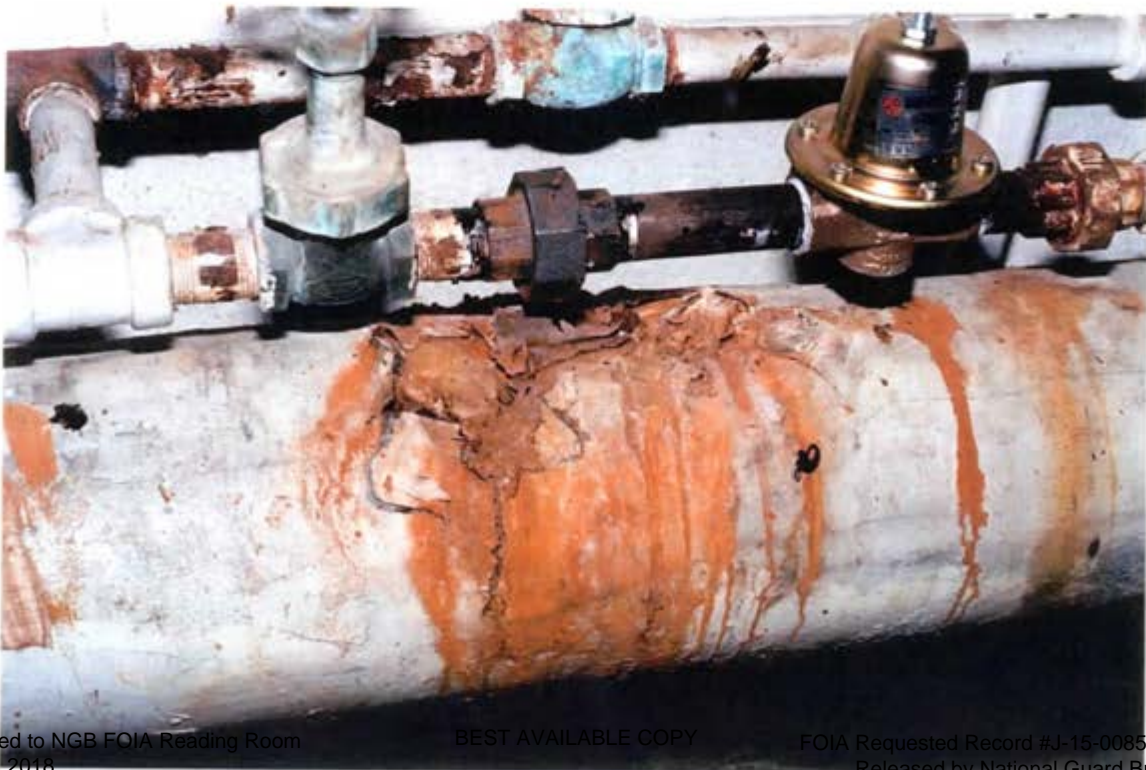
Broken Pipe Wrapping
