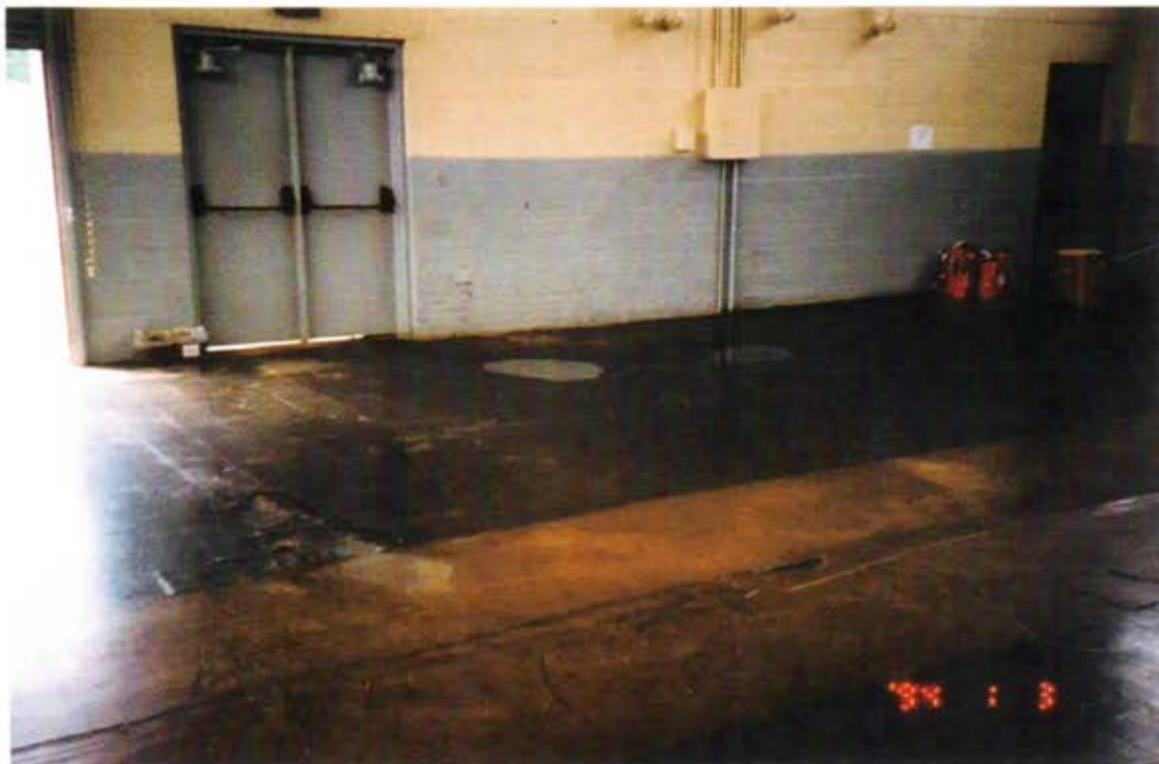
Views of Entrances of Rain and Water Puddles in the Red Springs Armory Drill Hall
