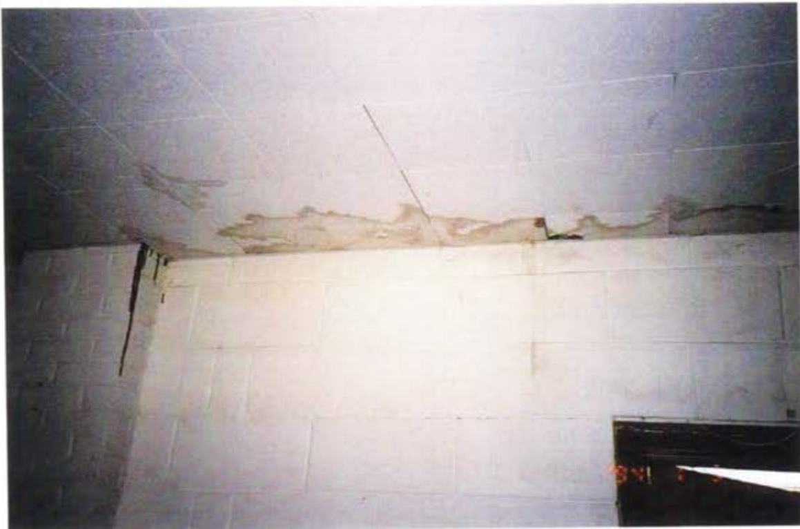
Water Damage located on the Ceiling inside of Classrooms
