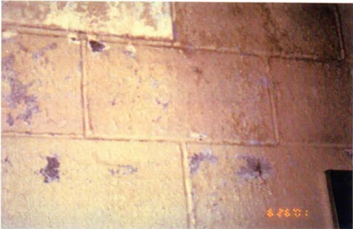
PARKTON NG ENLISTED BATHROOM DAMAGE FROM WATER LEAK
