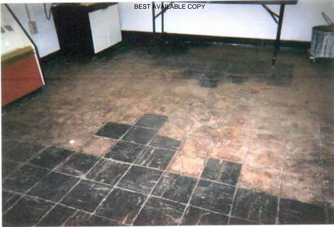
Missing, Broken Floor Tiles, Library
