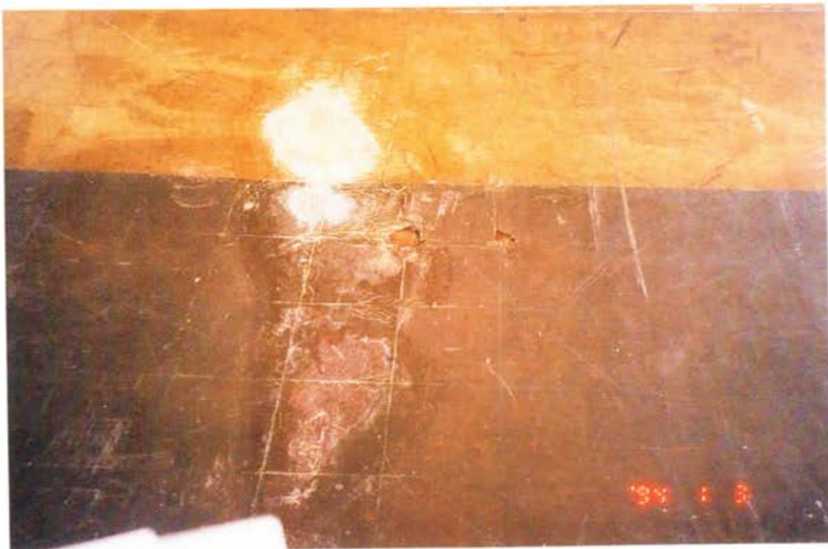
Views of Cracked and Broken Floor Tiles Puddle Located in the Armory Drill Hall
