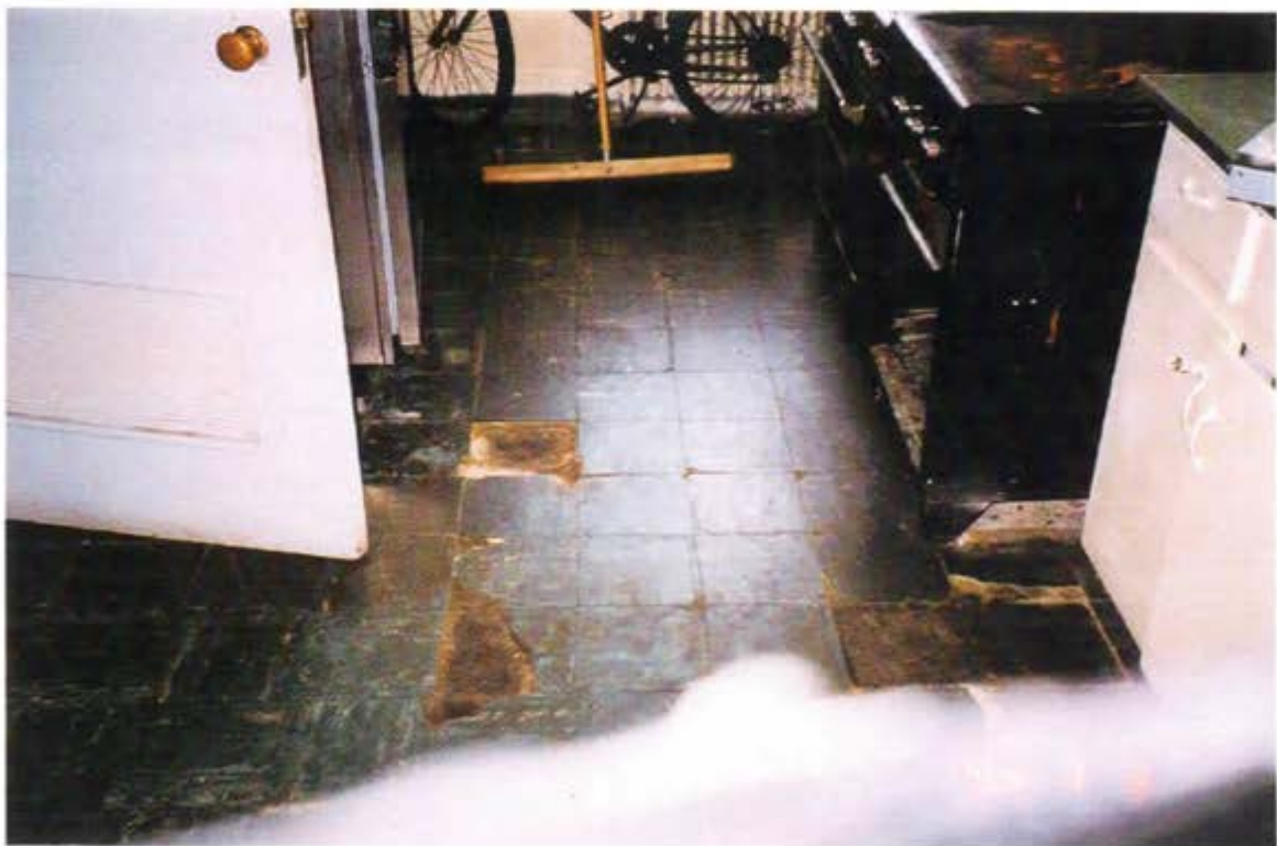
Views of Kitchen Broken and Missing Floor Tiles and Dated Mess Kitchen
