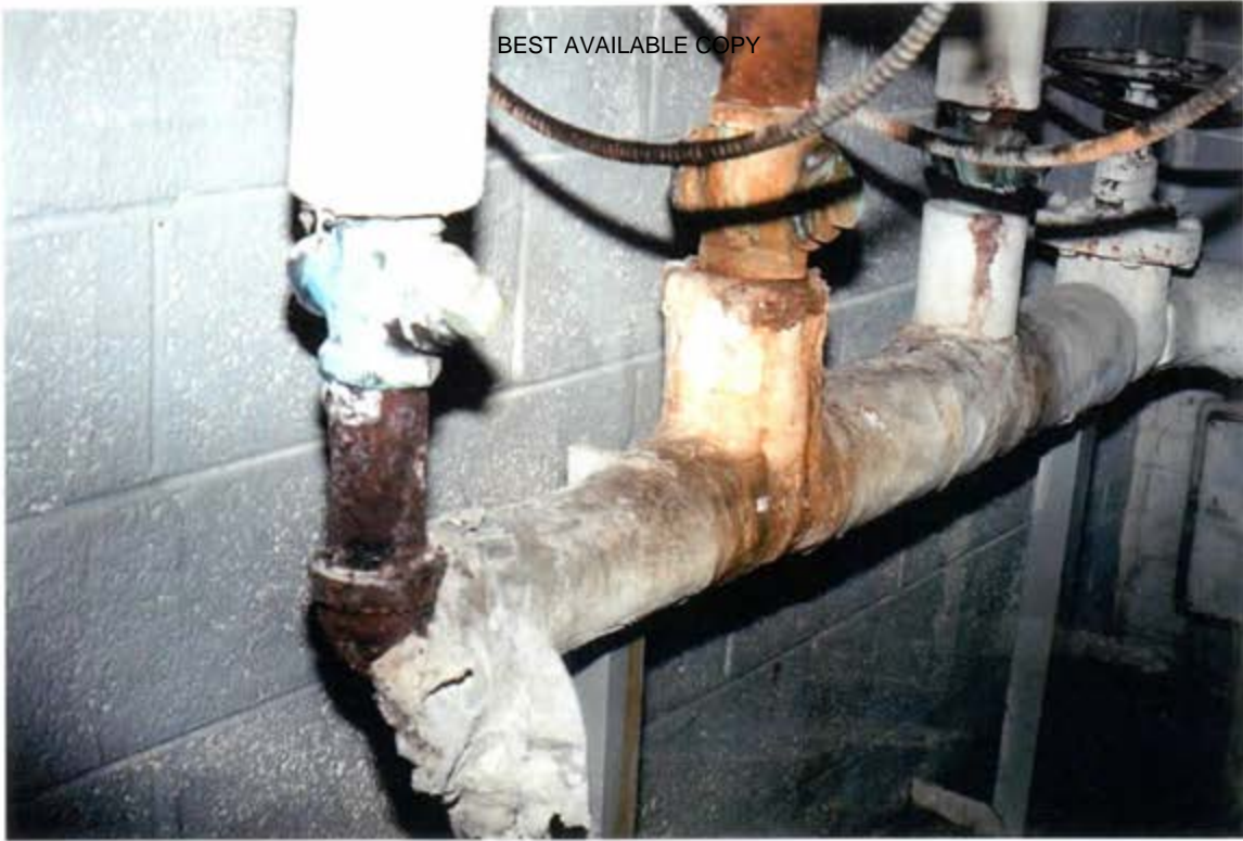
Broken Pipe Wrapping Boiler Room
