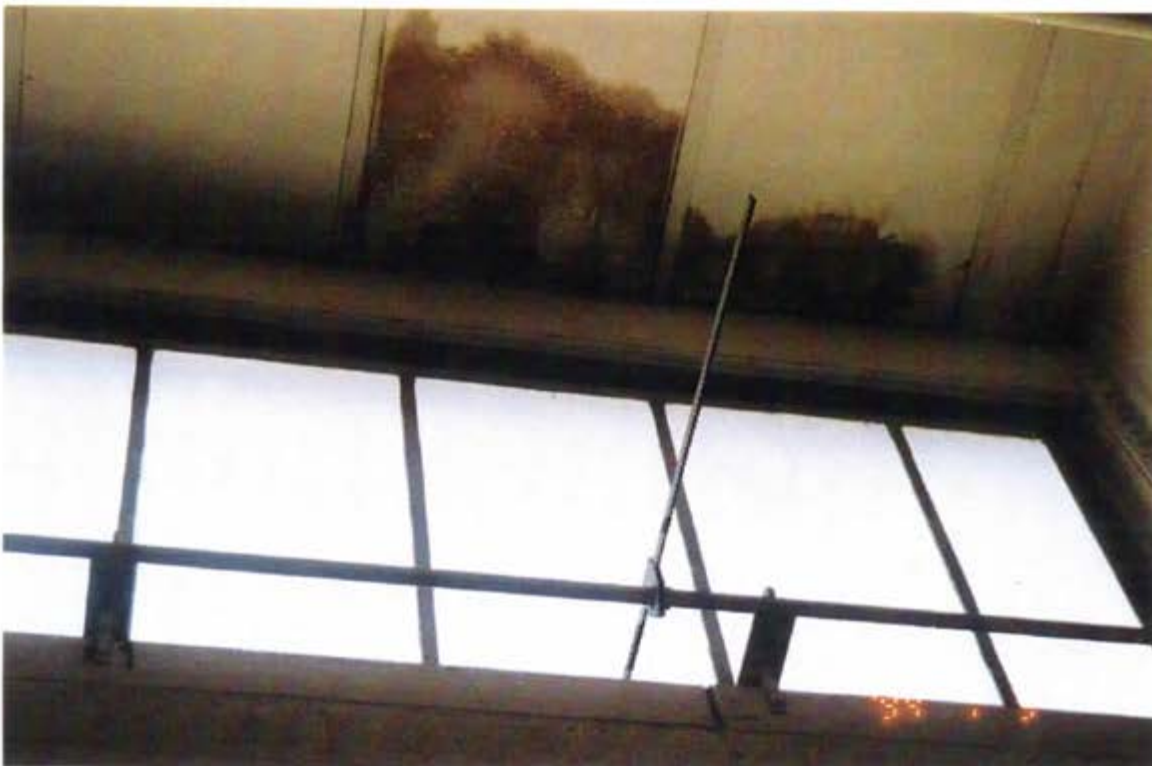
Views of Water Damage of Ceiling in Drill Hall
