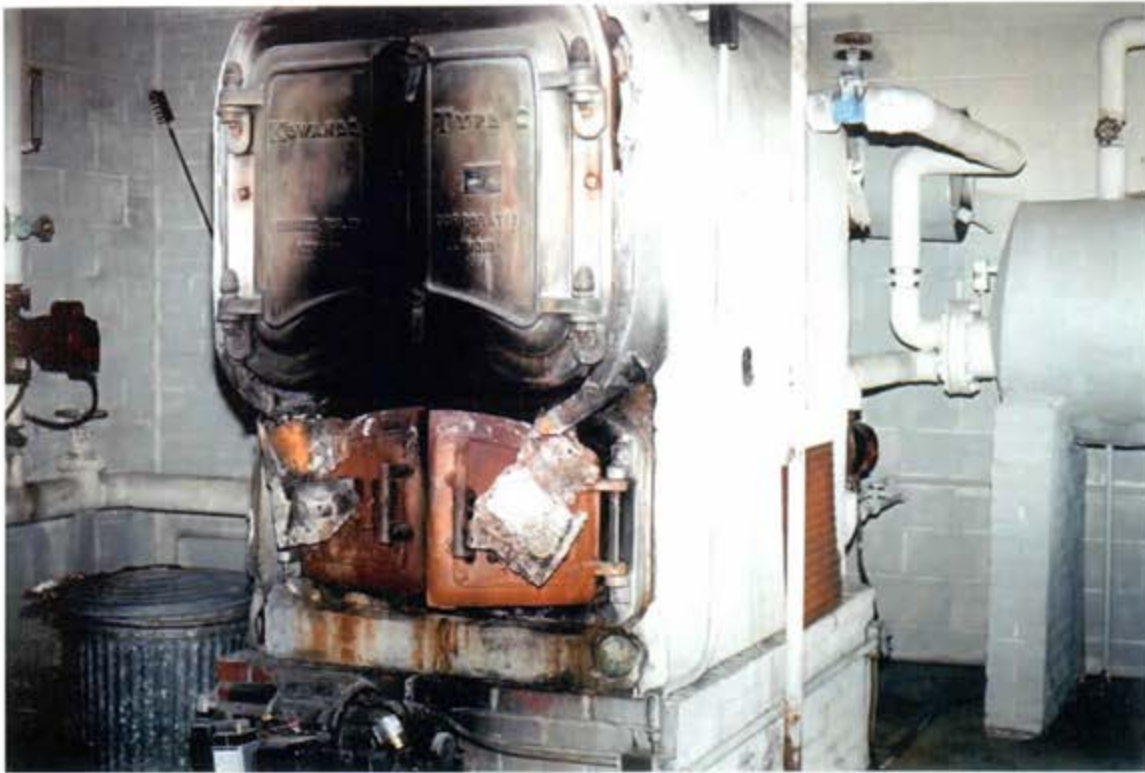
Broken Wrapping Boiler
