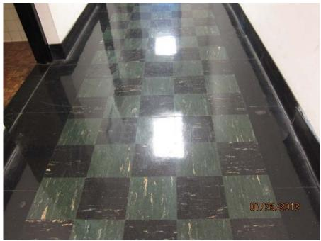
Suspect asbestos floor tile in good condition
