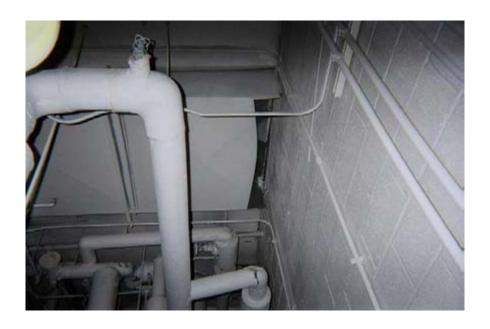
Photograph #10 – Boiler Room – Abandoned duct from old firing range (currently separated from HHC Lower Level Storage by block wall)
