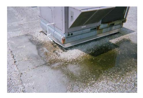
Photograph #4 – Roof-mounted Package HVAC unit, intake area, pooled water
