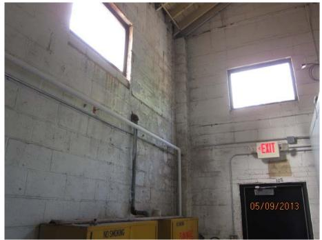
Effloresces on the exterior walls of the converted maintenance bay
