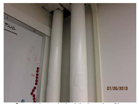
Suspect asbestos pipe insulation in good condition
