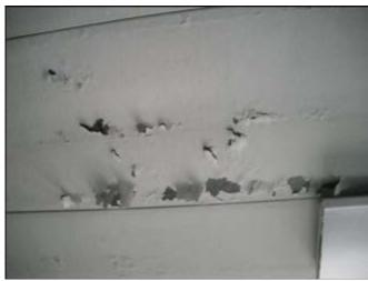
Rm. 201, peeling lead based paint on ceiling
