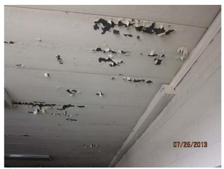
Second floor wall locker storage area peeling paint on ceiling
