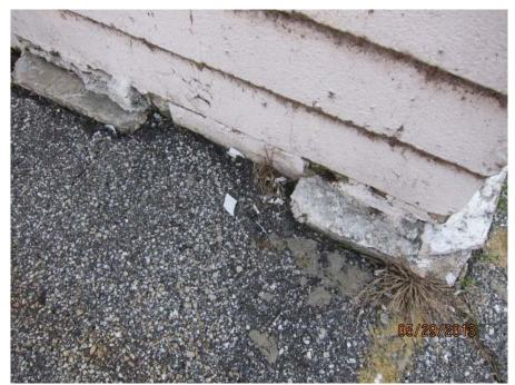
Exterior of facility suspect asbestos shingles and suspect lead-based paint on ground at drip line around the facility
