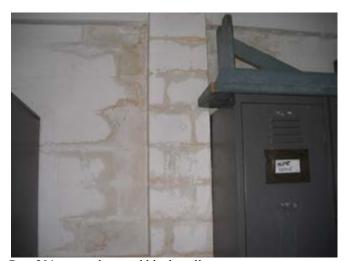
Rm. 201, water damaged block wall
