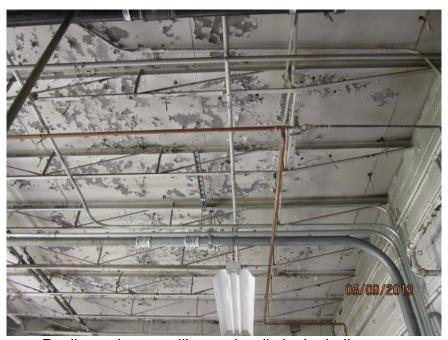
Peeling paint on ceiling and walls in the boiler room
