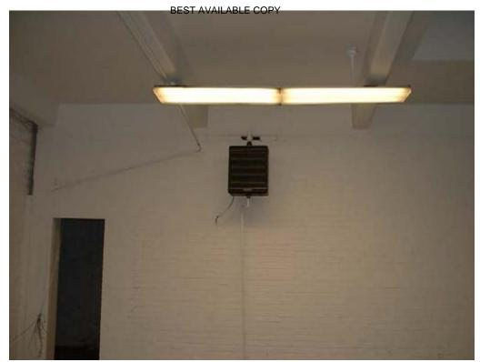
Wall mounted heater located in 212. Elevated levels of surface lead on heater blades.
