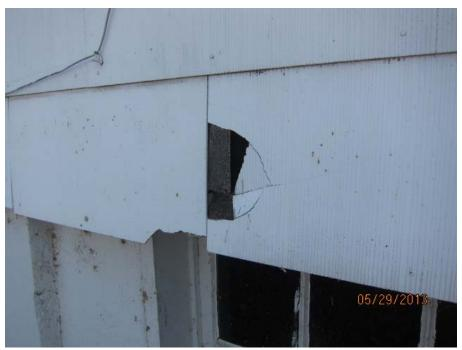
Exterior damaged suspect asbestos shingles
