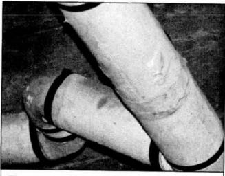
Figure F-8. Garage, pipes with TSI
