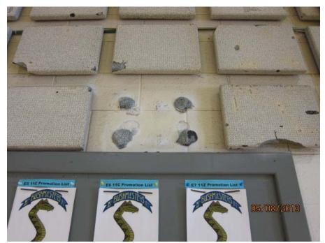
Suspect asbestos black mastic dots on walls and ceiling in the drill hall
