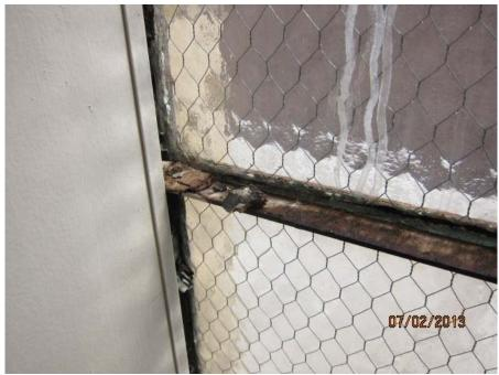
Suspect asbestos window glazing damaged and in poor condition in the weight room.
