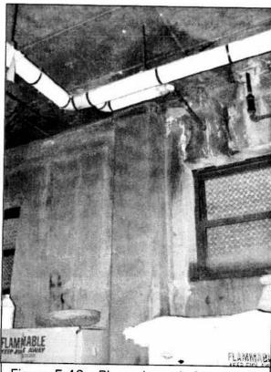
Figure F-49. Pipes through foundation causing water intrusion
