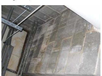
Boiler Rm., SE corner, water damage from ceiling down
