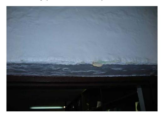
Photograph #6 – Water Damage at Entrance to Supervisor's Office
