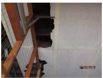
Inside one of the old stables/storage area suspect asbestos damaged transite board
