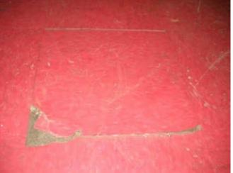
Room 15, damaged presumed asbestos containing 12"x12" floor tile
