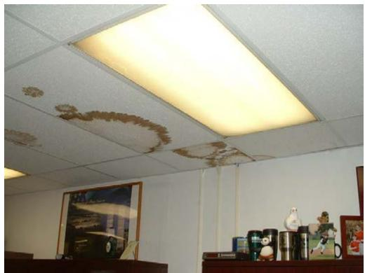
Water damaged ceiling panels in Room 12 (2<sup>nd</sup> Floor)
