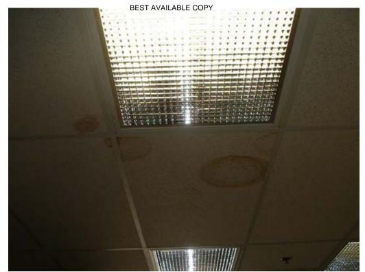
Water damaged ceiling panels, Room 4
