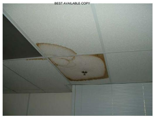
Water damaged ceiling panels, Room 27
