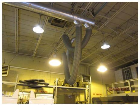
Overhead vehicle exhaust system (not functional)
