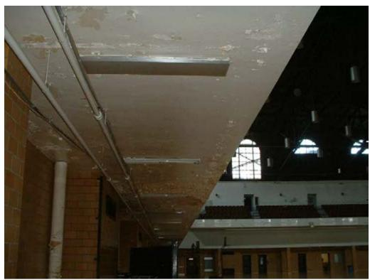
Deteriorated paint on Drill Floor at Room D25
