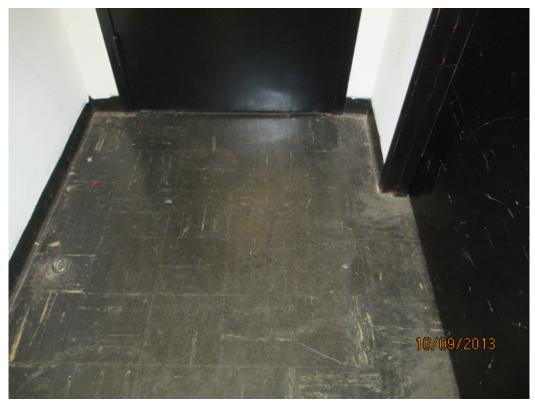
Suspect Asbestos Containing Material 9"x9" Floor Tile
