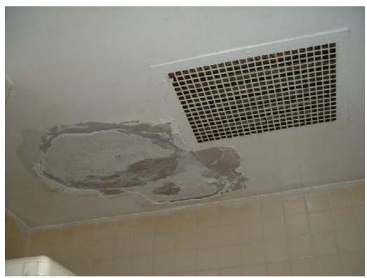
Water damaged plaster in latrine
