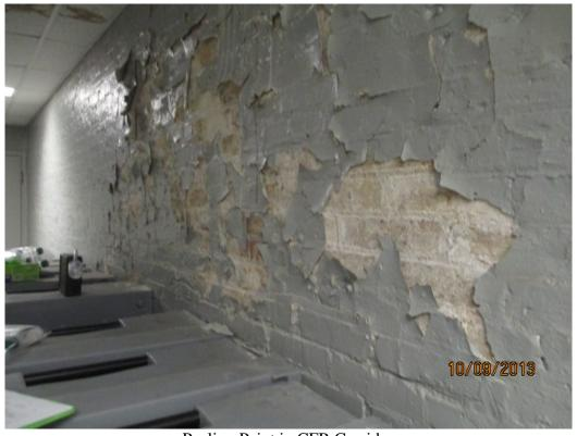
Peeling Paint in CFR Corridor
