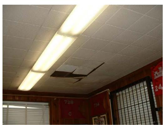
Water damaged ceiling tiles in the main level kitchen
