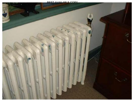
Deteriorated paint on radiator, M25
