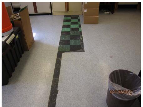
Suspect asbestos floor tile in good condition
