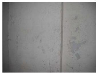
Boiler Room, west wall, peeling lead based paint
