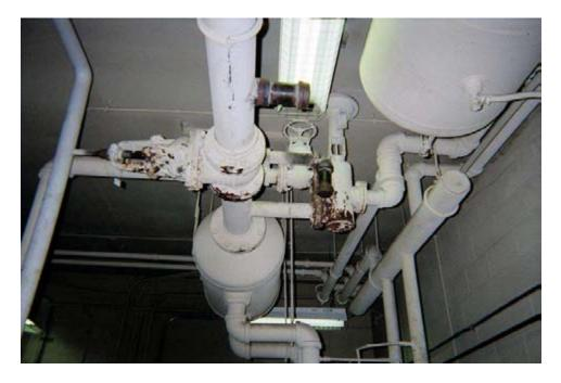
Basement, Boiler Room, delaminating paint from valves
