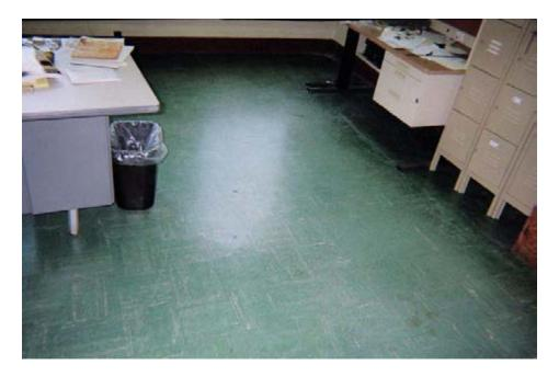
Main Floor, Old Signal Command Office, view of 9 inch square floor tile (presumed asbestos-containing)
