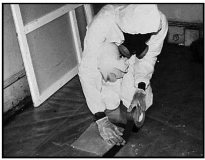
Figure 14.7 Plastic Sheeting Should Be Repaired as Part of Daily Cleanup.
