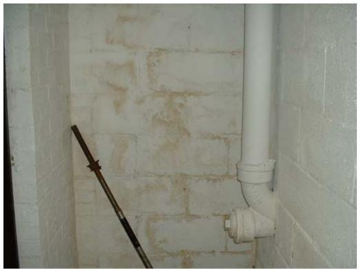
Water intrusion through subgrade wall (Room B1)
