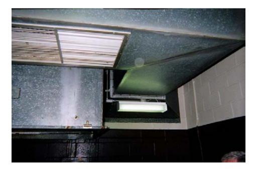
Photograph #9 – Kitchen, outdoor/make-up air duct/vent
