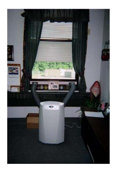
Photograph #10 – Distance Learning Center office, portable "drainless" air-conditioner, (vent intake and exhaust to outdoors)
