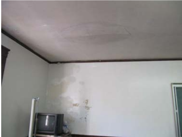
Water Damaged Wall and Ceiling in Classroom
