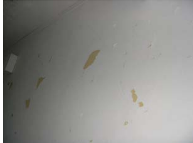
Flaking Paint on Walls
