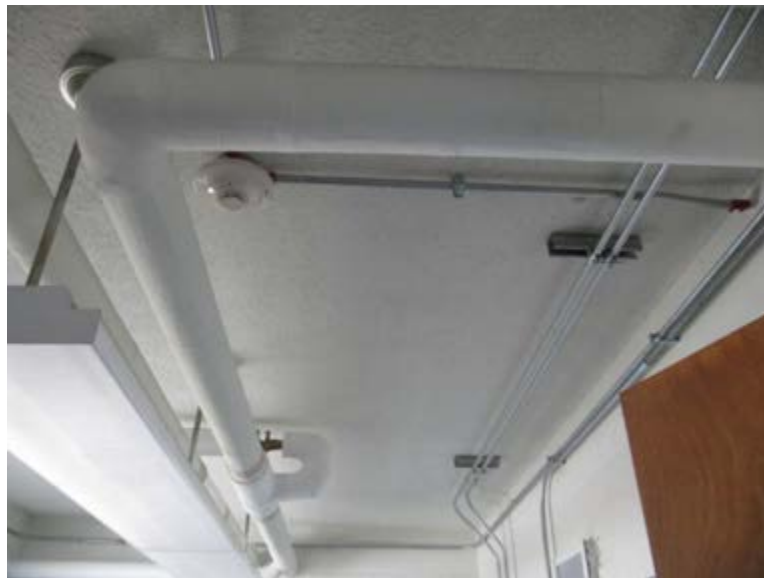
Fiberglass Pipe Insulation
