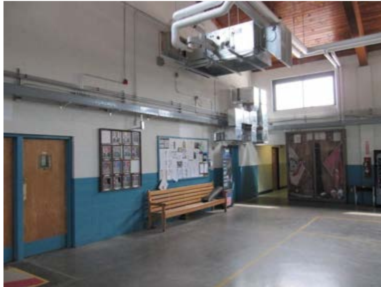
Air Handling Unit in Drill Shed
