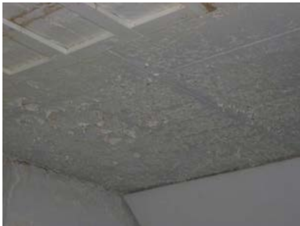
Flaking Paint on Ceiling
