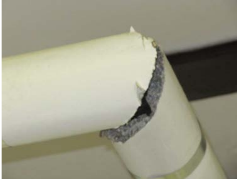
Typical ACM Pipe Insulation
