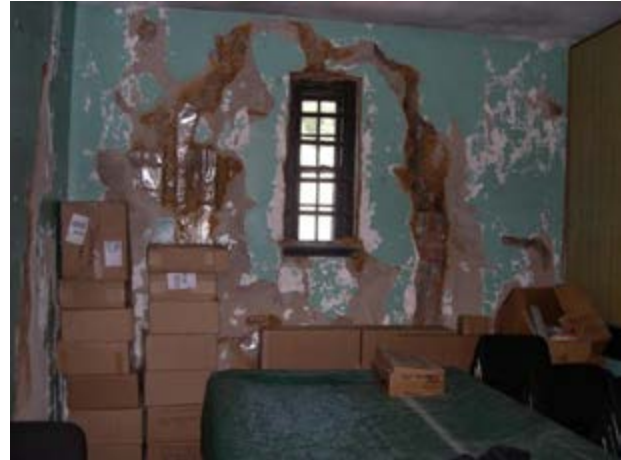
Flaking Paint and Damaged Plaster
