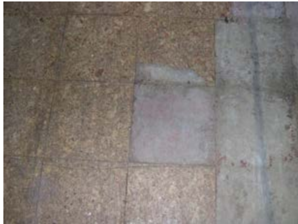
Damaged Floor Tile
