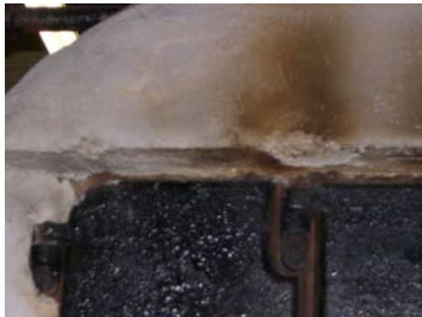
Damaged Boiler Breeching
