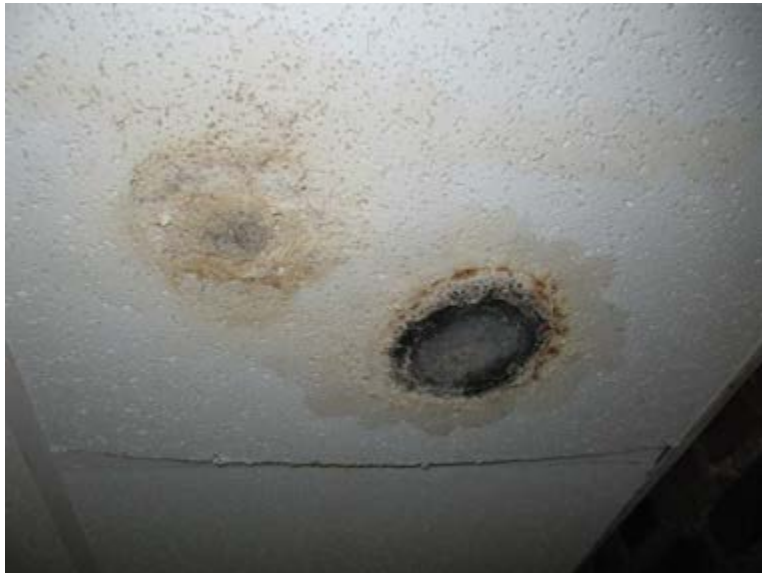
Water Stained Ceiling Tile and Visible Mold Growth in Mess Hall
