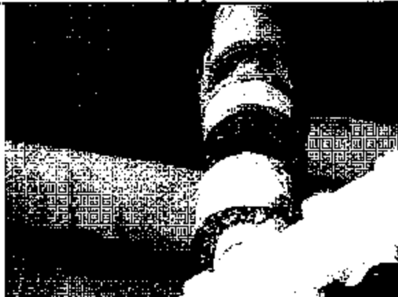
Photo 3578: Supply Room #3 - Damaged asbestos-containing pipe insulation
