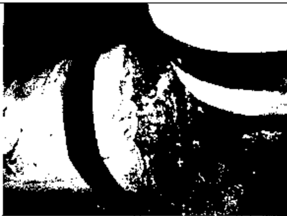
Photo 3407: Open Area #11 - Damaged asbestos-containing pipe insulation
