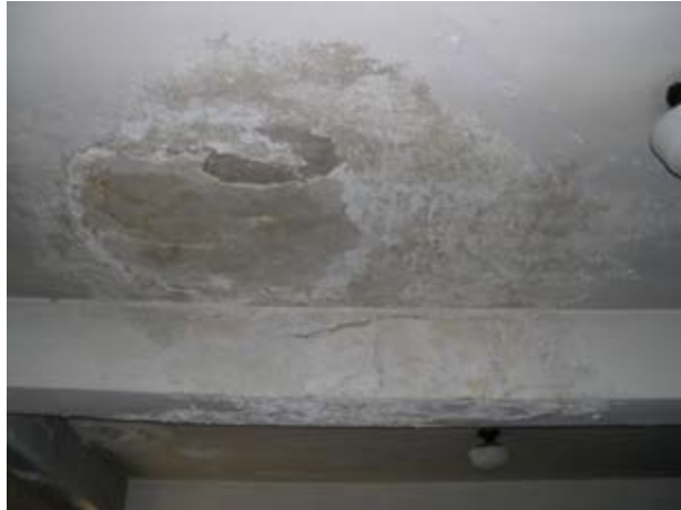
Damaged Plaster and Peeling Paint on Ceiling
