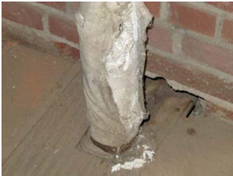
Damaged ACM Pipe Insulation in Basement
