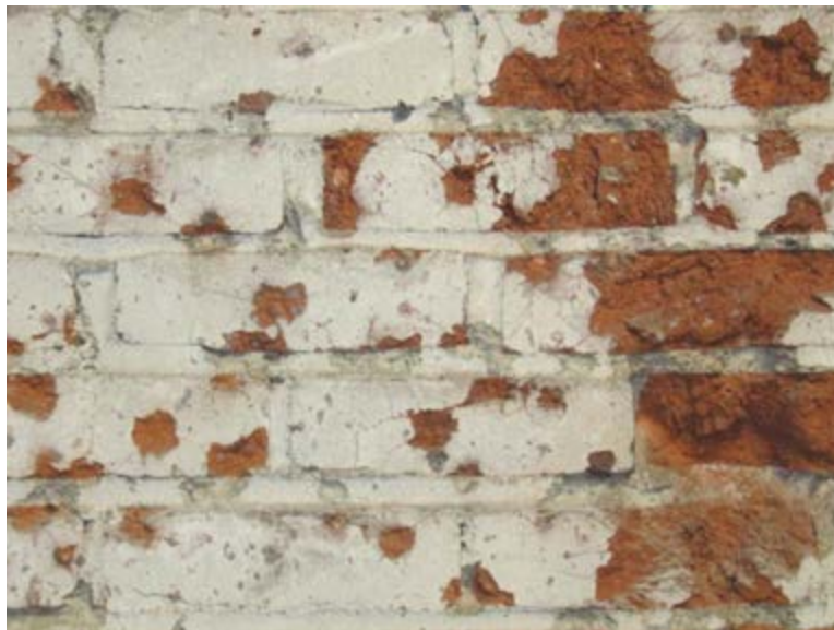
Range Wall with Visible Lead
