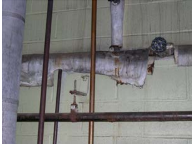
Boiler Room, Damaged TSI
