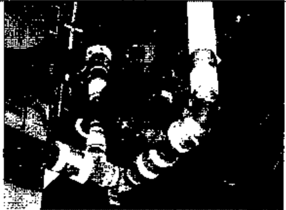
Photo 3673: Drill Shed #21 - Damaged asbestos-containing pipe insulation
