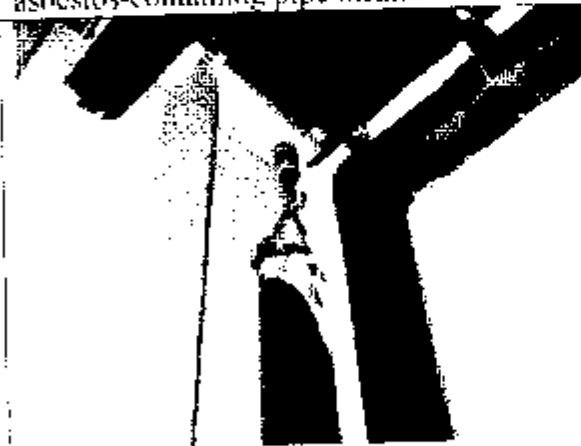
Photo 3719: Room 12A - Damaged asbestos-containing pipe insulation
