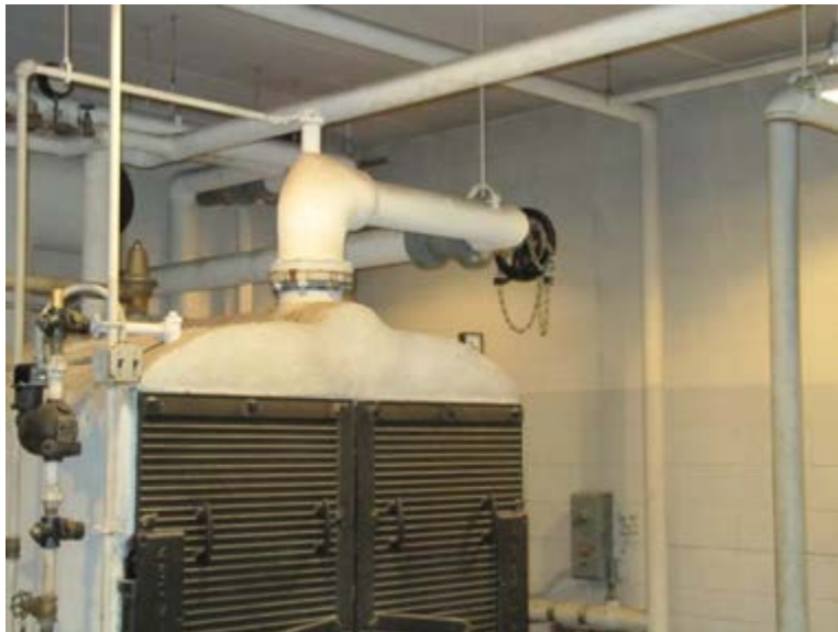
Boiler Room and ACM Insulation
