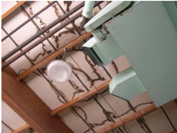
Water Intrusion on Ceiling
