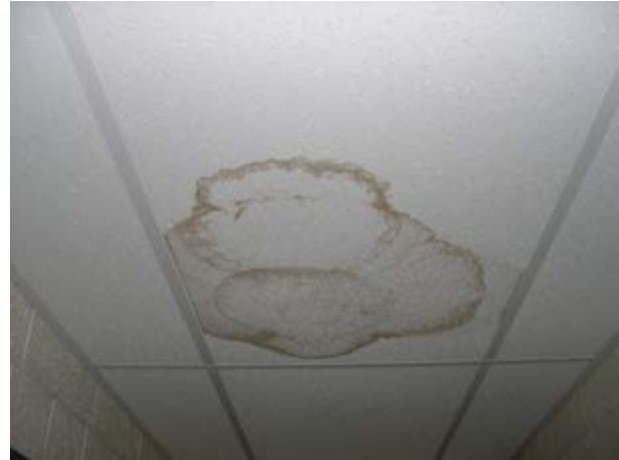
Water Intrusion on Drop Ceiling
