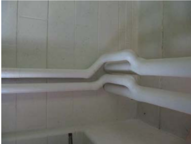
Typical Pipe Insulation
