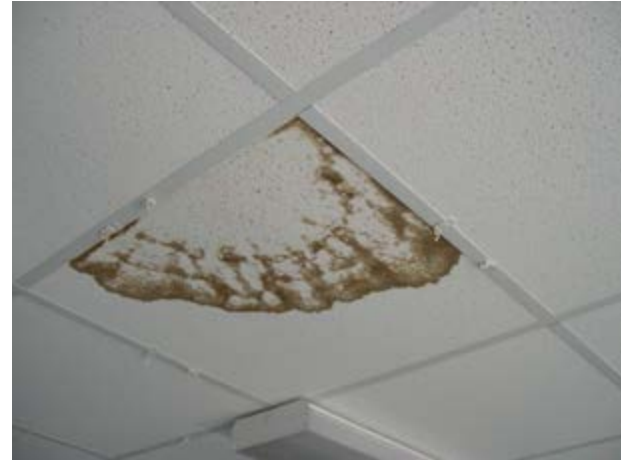
Water Intrusion on Drop Ceiling
