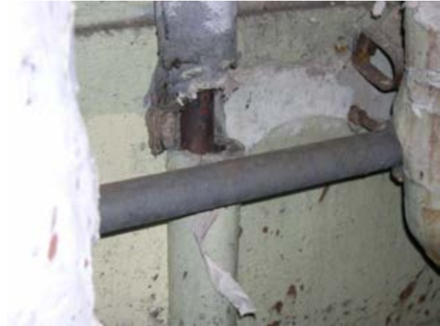
Boiler Room, Damaged TSI
