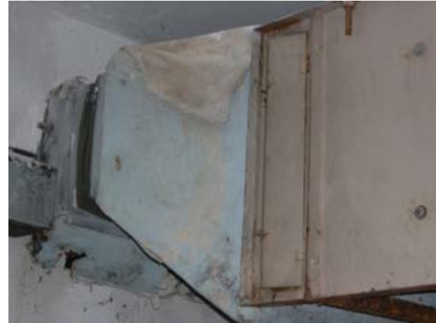
Damaged Air Handler
