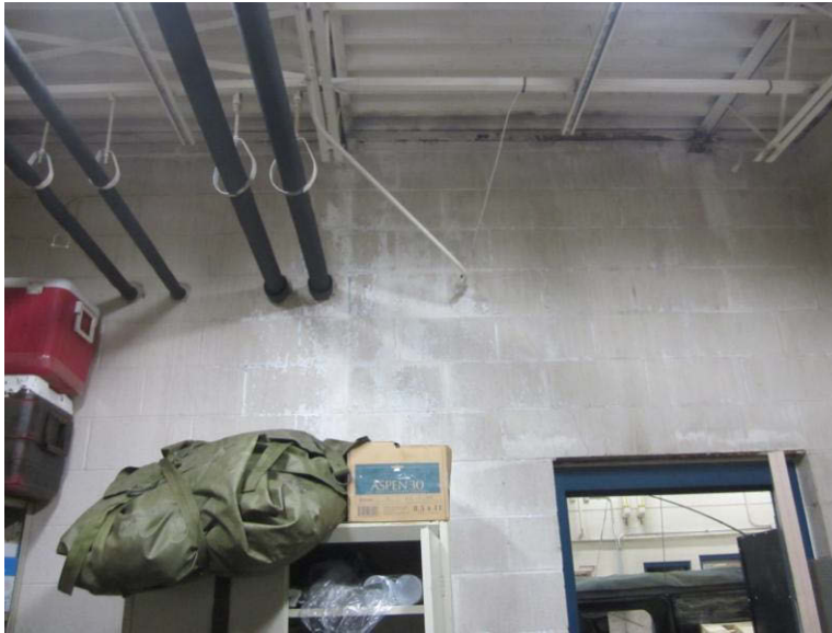
Figure C-2 – Water Damage and Efflorescence on Cement Block Wall in RSP Storage Room
