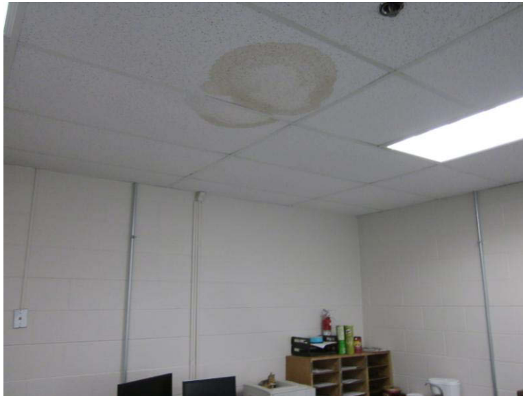
Figure C-1 – Water Damage and Mold on Ceiling Tile in 1-161 Orderly Room
