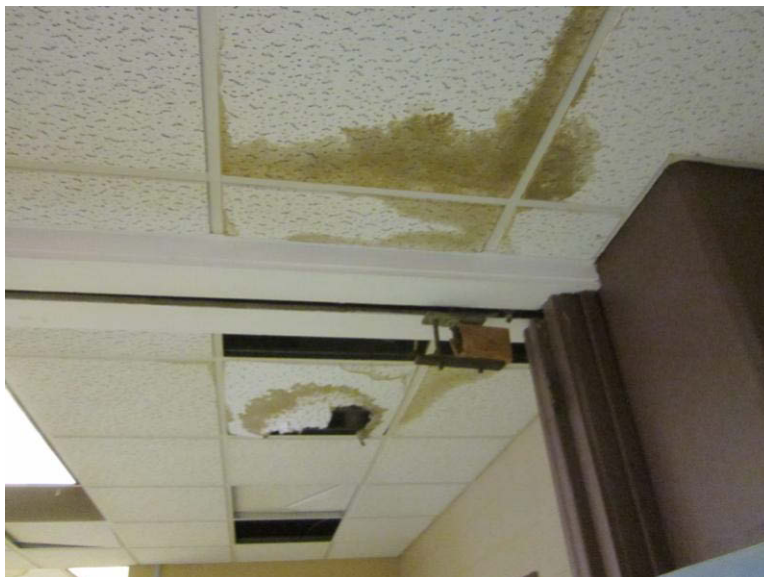
Figure C-4 Water Damage and Mold on Ceiling Tiles in Basement Kitchen and Dining Area
