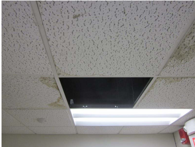
Figure C-1 Water Damage and Mold on Ceiling Tiles in the West End of the John W. Briedenthal Hall
