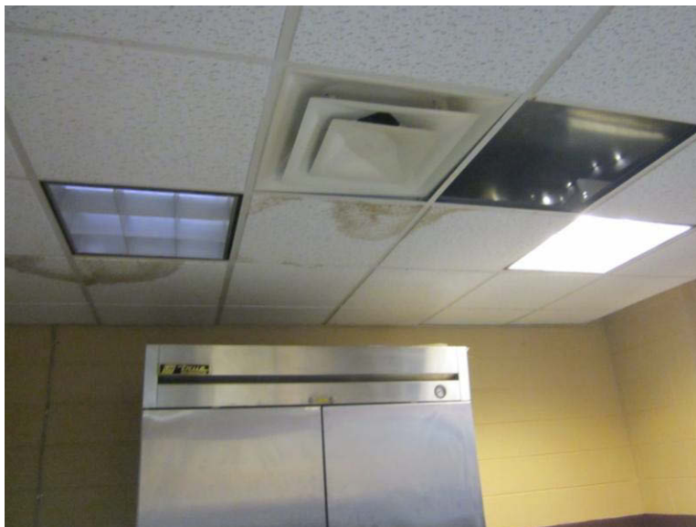
Figure C-2 Water Damage and Mold on Ceiling Tiles in First Floor Kitchen Area
