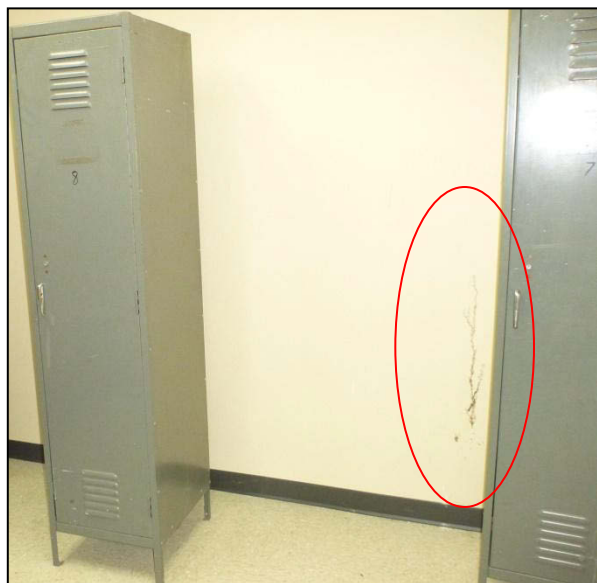
Figure 4 - Possible Termite Damage in the Platoon Office Area.
