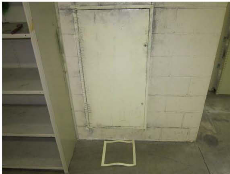
Figure 2 – Access door to bullet trap with visible silver/gray deposits that originate from the edge of the sealing area of the access door.
