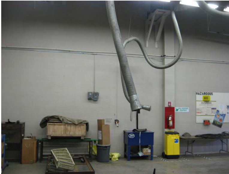
Figure 3 Tailpipe LEV
