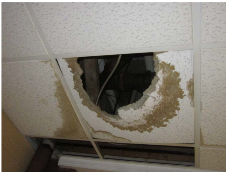
Figure C-3 Water Damage and Mold on Ceiling Tiles in Basement Kitchen and Dining Area - Beneath Leaking Cast Iron Waste Pipe
