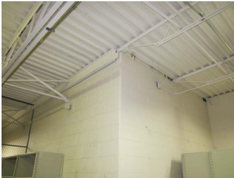
Figure 4 -Unsealed areas above partition wall between firing range and FA storage room
