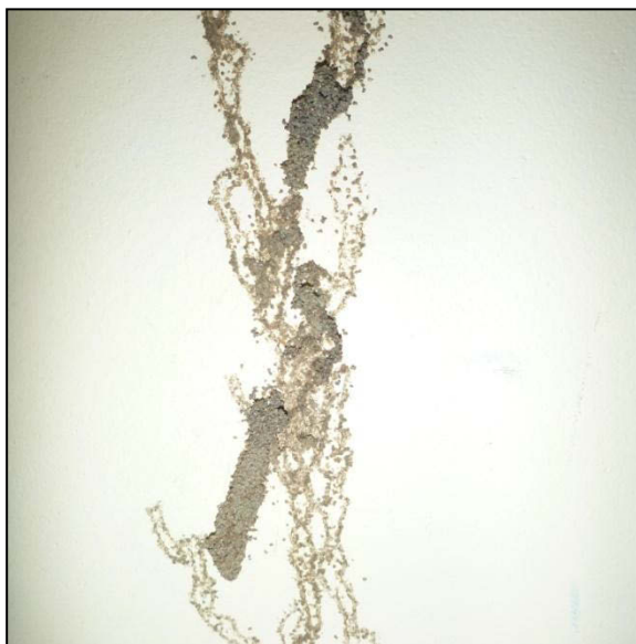
Figure 4 - Possible Termite Damage in the Platoon Office Area.
