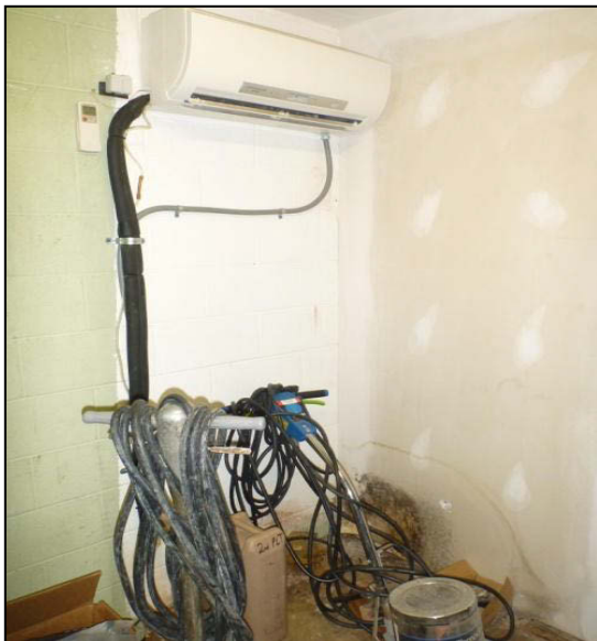
Figure 3 - Mold in the Server Room.
