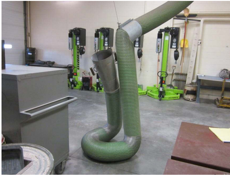
Figure C-1. Tailpipe Exhaust System.
