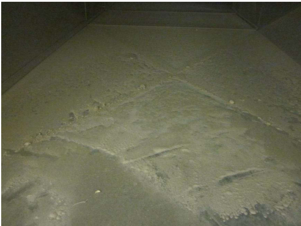
Figure A-1 Dust Accumulation Inside of Return Air Duct, Near the Area Where Sample IAOSIFW9 Was Collected
