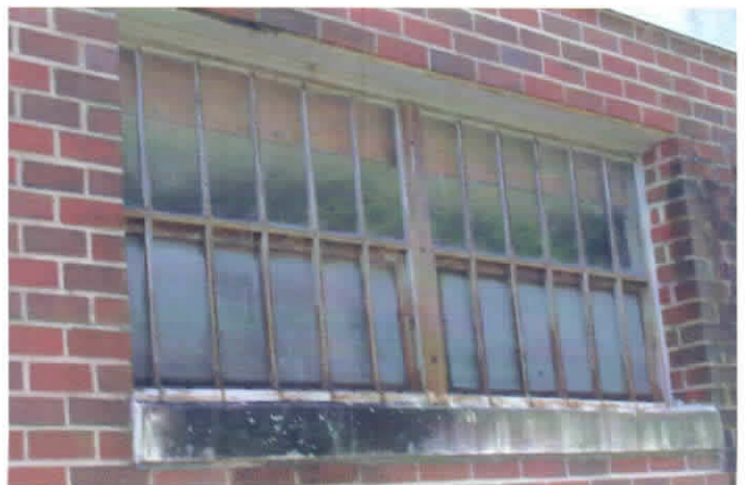
View of dirt and mold growth window
