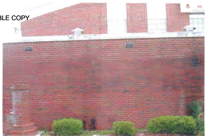
Excessive moisture on bricks of the building
