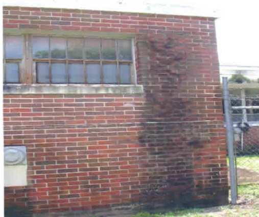
View of water staining and mold growth on brick of the building
