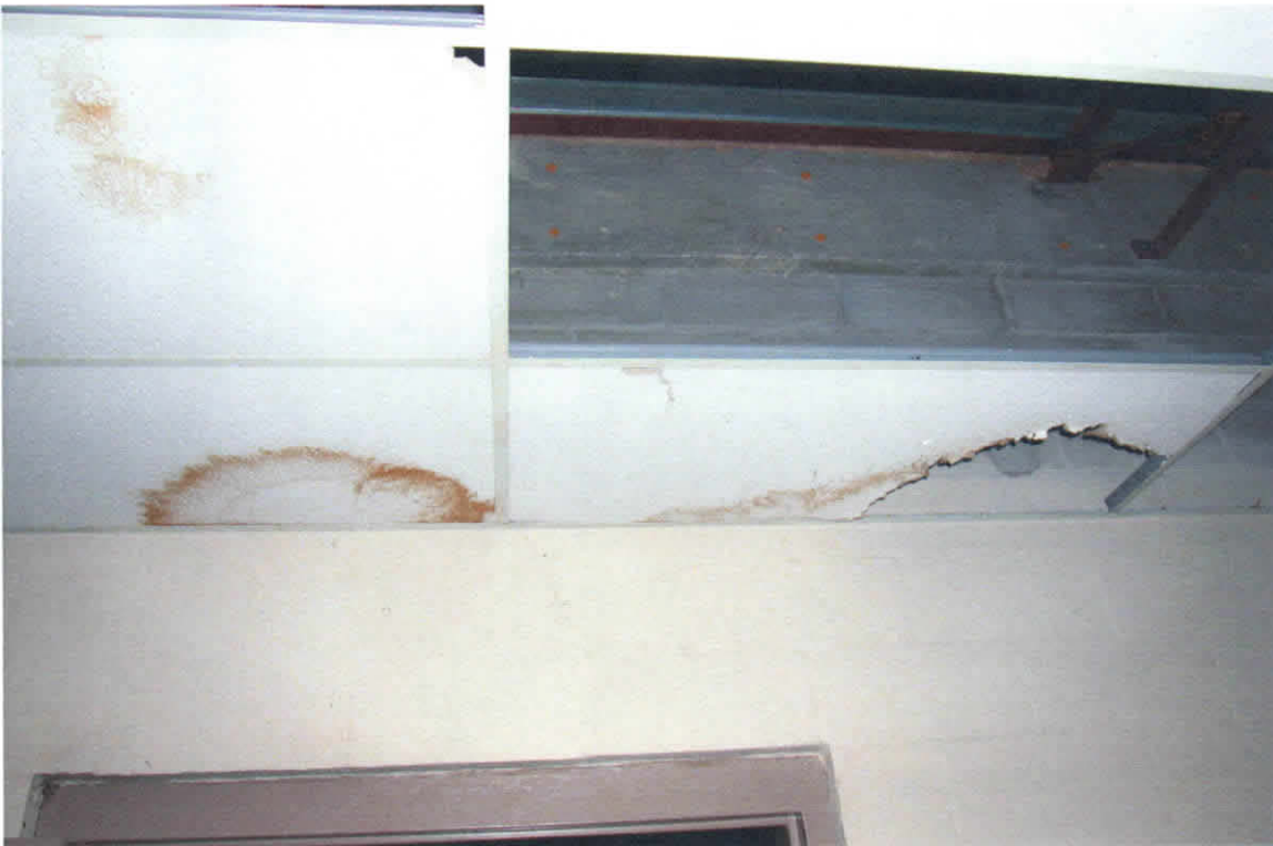
Photo 6: Water damaged ceiling tiles in armory.
