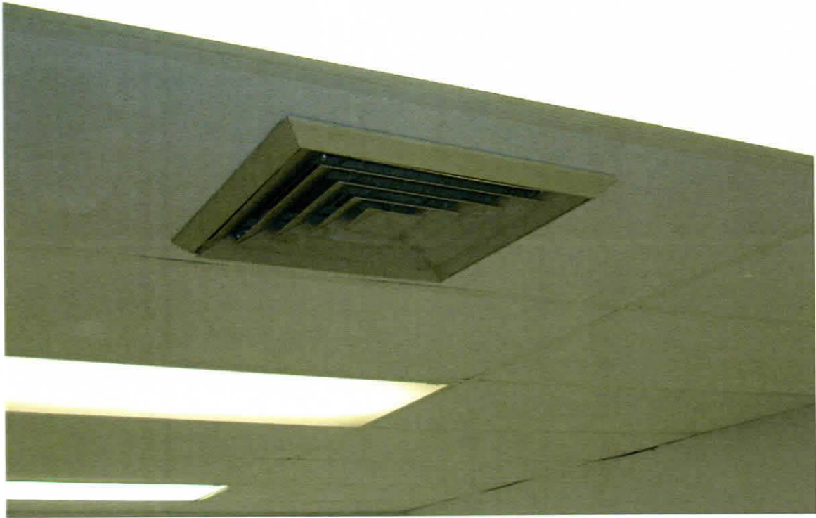
Photo 13: Another type of supply air diffuser for the office area.
