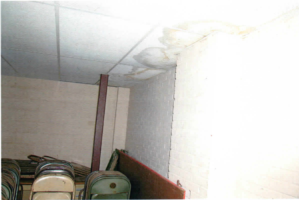
Photo 13: Stained ceiling tile in storage area
