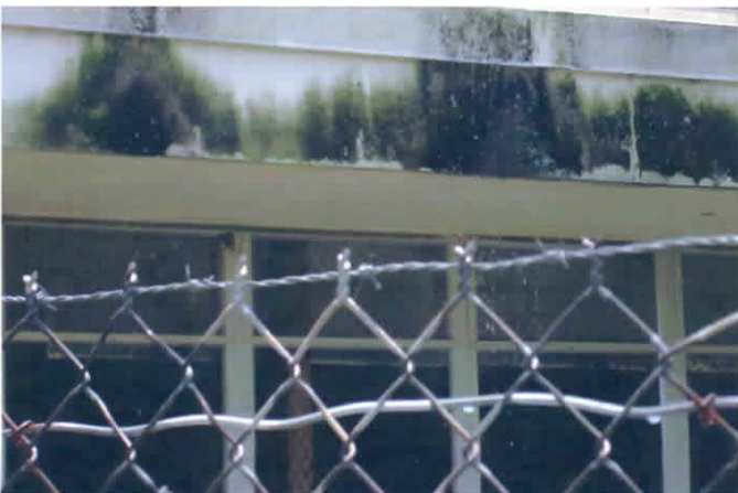
View of dirt and mold growth along fascia of the building
