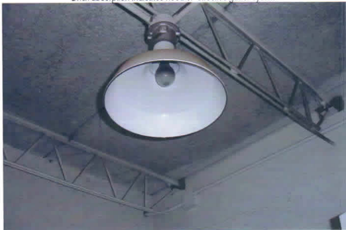
View of kitchen lighting with bulbs that are not shatter proof
