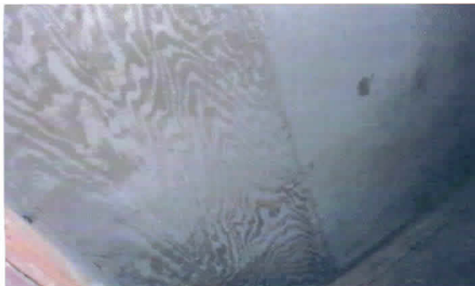
View of concrete ceiling. The wood pattern may be from the wood that was removed when associated range items were removed.
