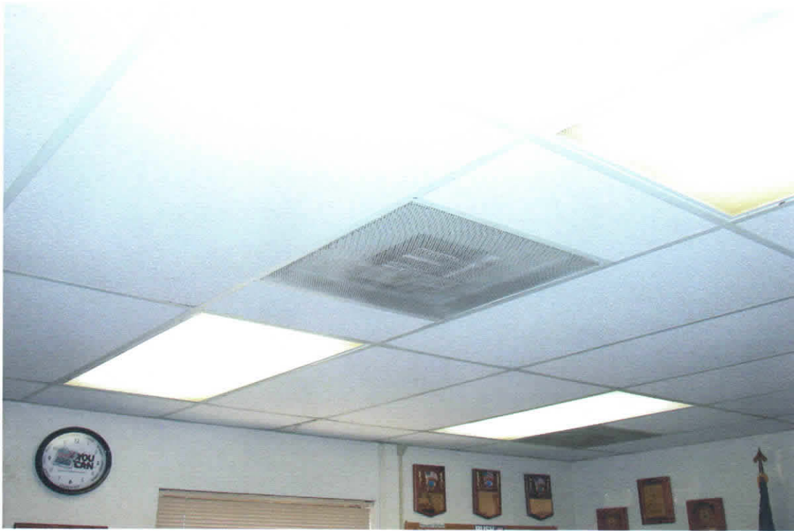
Photo 7: Air supply diffuser in administrative office.
