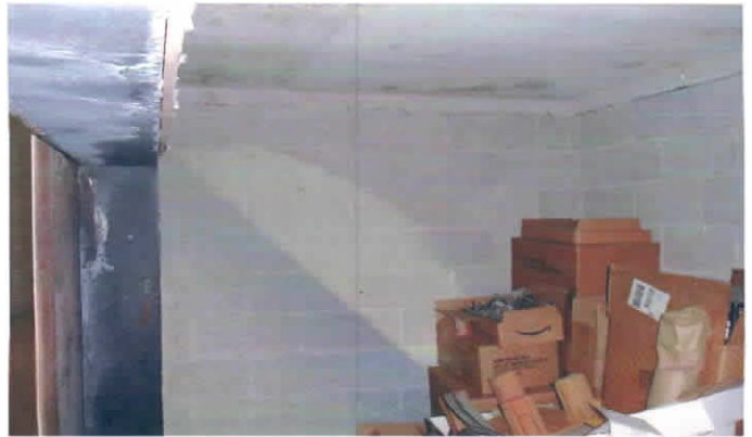
View of left wall inside space that held former backstop. The white color on blocks indicate where the backstop was mounted to the wall
