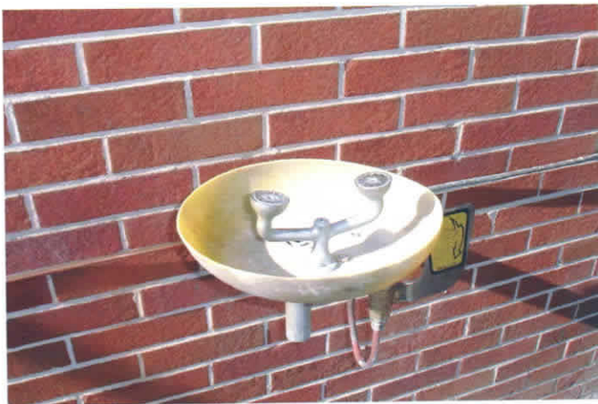
View of eyewash located outside the maintenance shop. The eyewash has no eye covers
