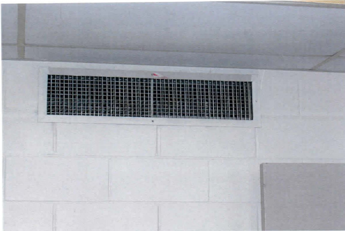
Photo 13: Air supply grill to office area.
