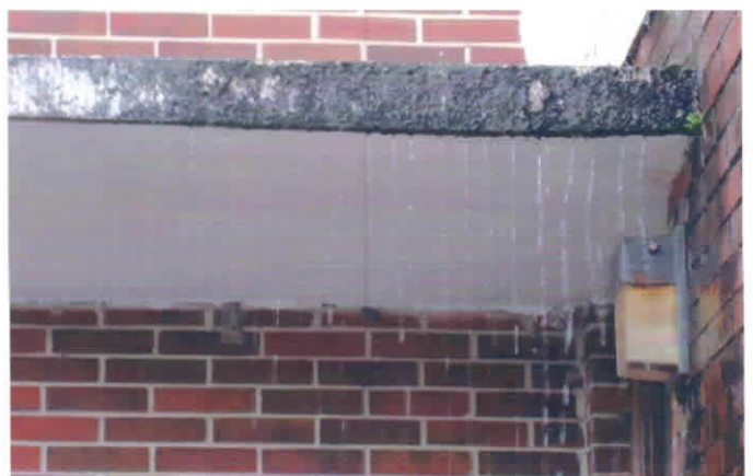
View of dirt and mold growth along fascia porch overhang. The need for an effective gutter.
