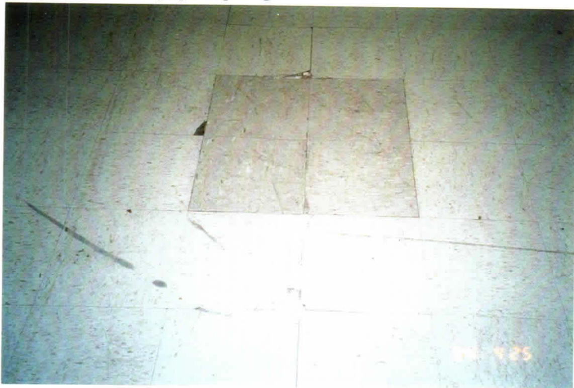
Photograph, Depicting Broken/Friable Asbestos Tiles
