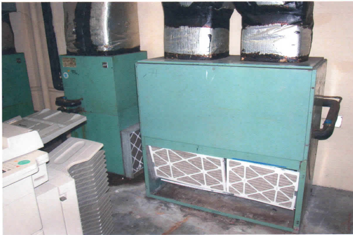
Photo 12: Air handling units to the office areas.
