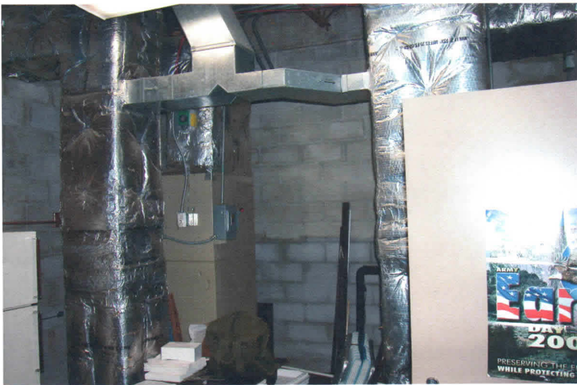
Photo 12: Air handling units showing the outside air connections.
