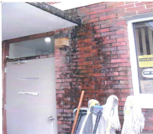
View of water coming from porch overhang during heavy rain shower. Brick absorption indicates need of effective gutter system.
