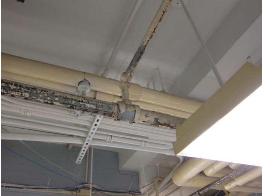
Peeling paint on pipes in kitchen
