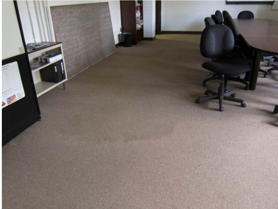
Conference room water stain on carpet from above ceiling mounted UV that leaked condensate water
