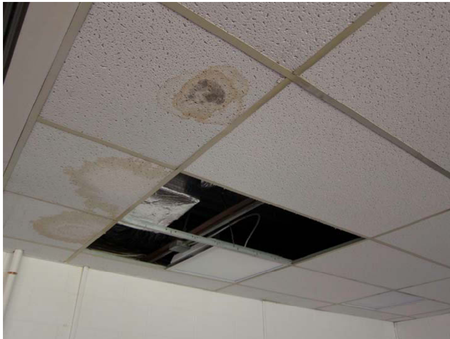
Conference room visible fungal growth, missing, and water stained ceiling tiles from above ceiling mounted UV that leaked condensate water
