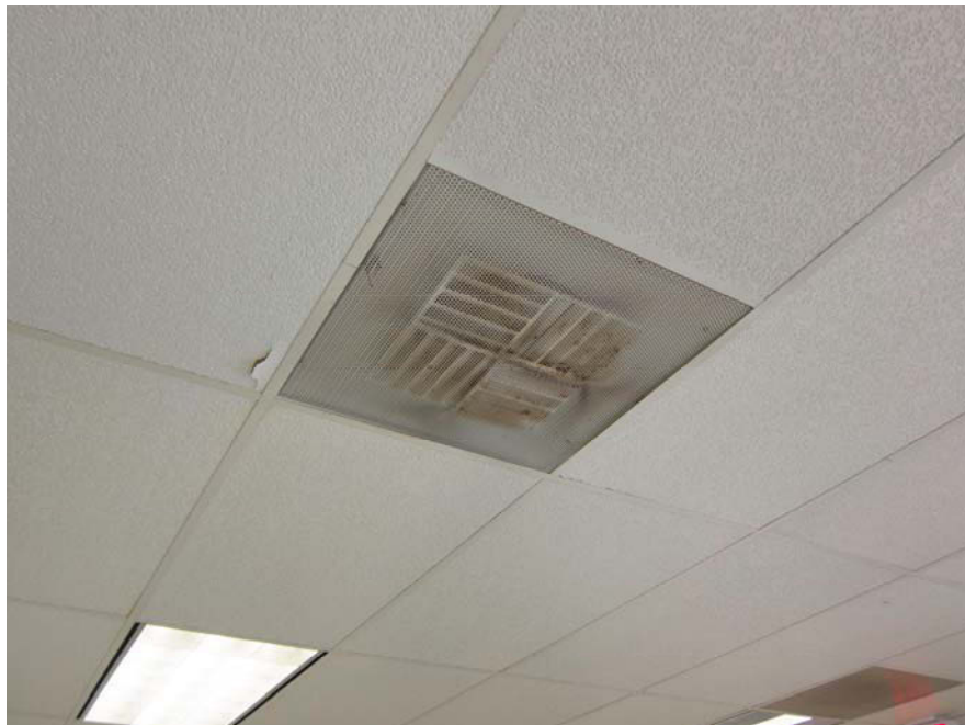
Drill hall dirty supply diffuser
