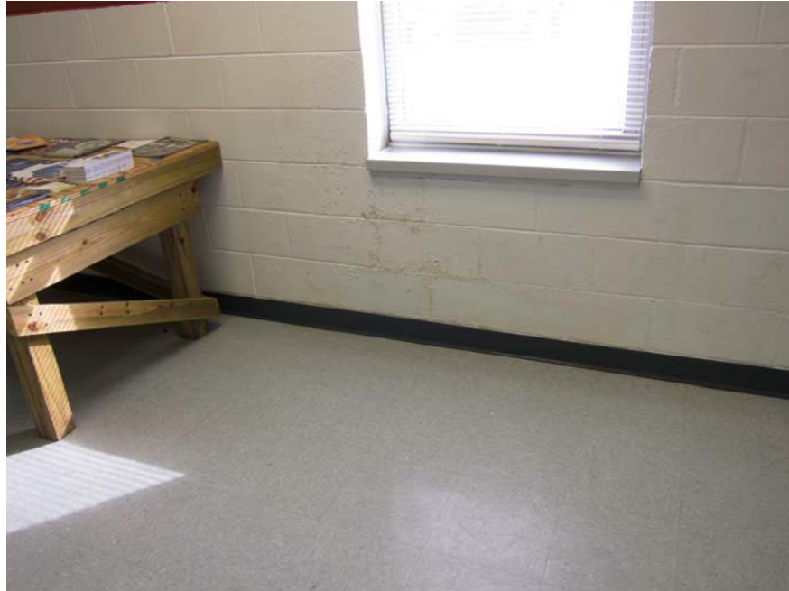
Drill hall efflorescence below window
