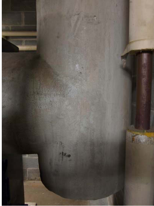
Mechanical room breeching possible ACM in good condition
