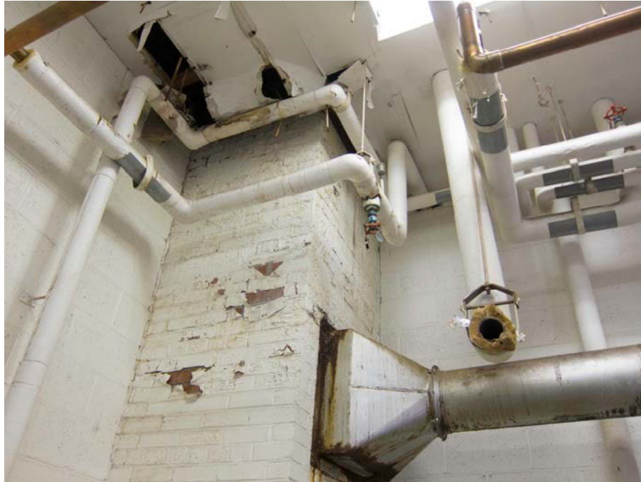
Boiler room peeling paint and water damage ceiling
