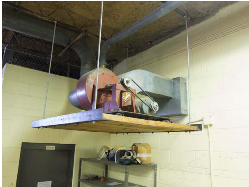
Inside the two bay detached garage overhead vehicle exhaust blower motor
