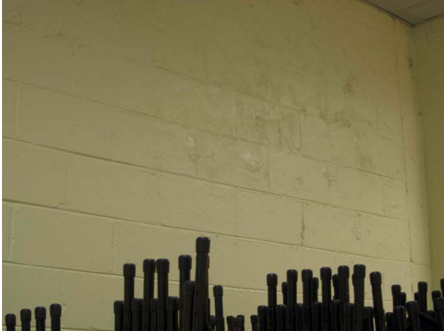
Dining hall efflorescence on exterior concrete block wall
