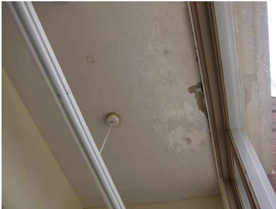
Front entrance water damage on ceiling plaster
