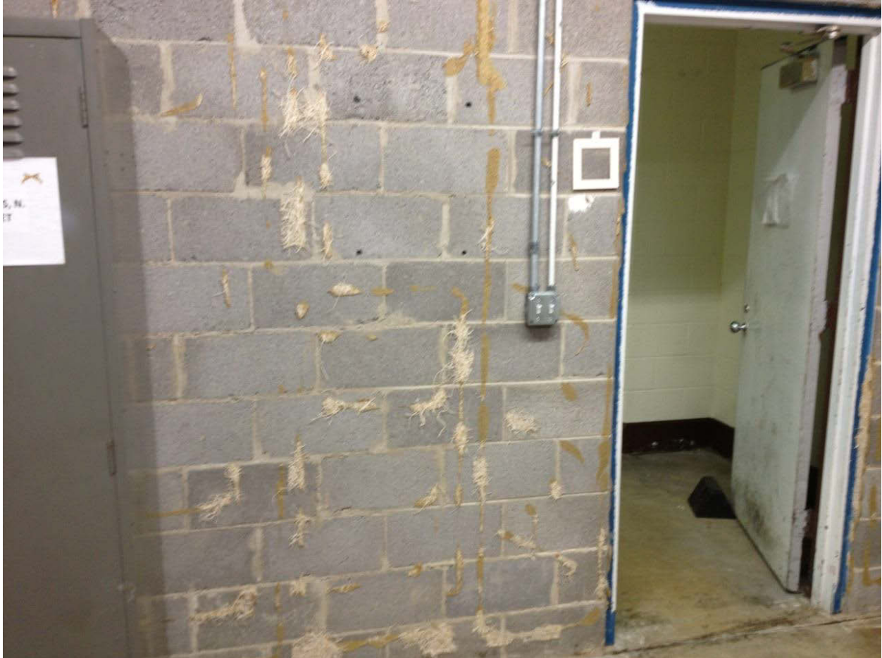
View of remaining soundproofing on wall.
