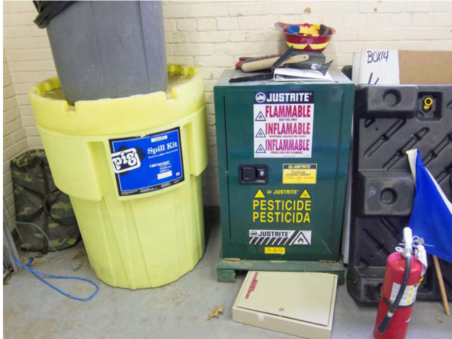
Garage flammable storage, fire extinguisher and spill kit
