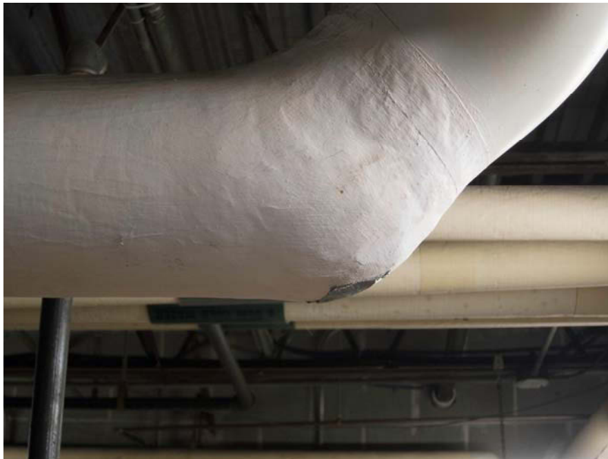
Mechanical room muddied pipe fitting possible ACM in good condition
