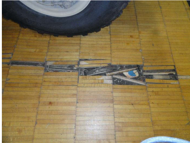
Damaged Parquet Floor
