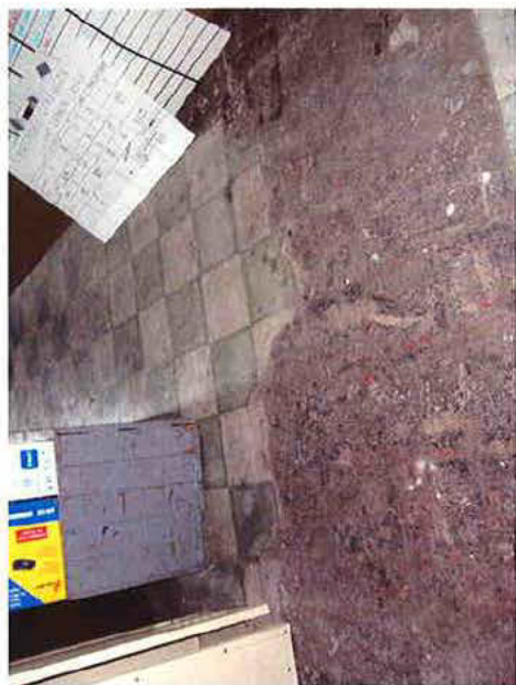
Photo 5: 3rd Floor Room 309B-Damaged ACM Floor Tile
