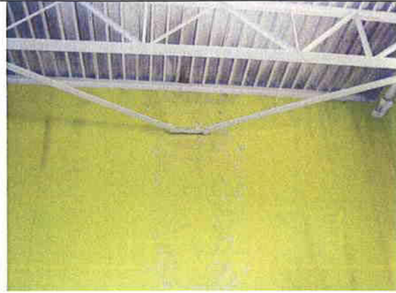
Photo 7049: Drill Hall – Water marks on wall
