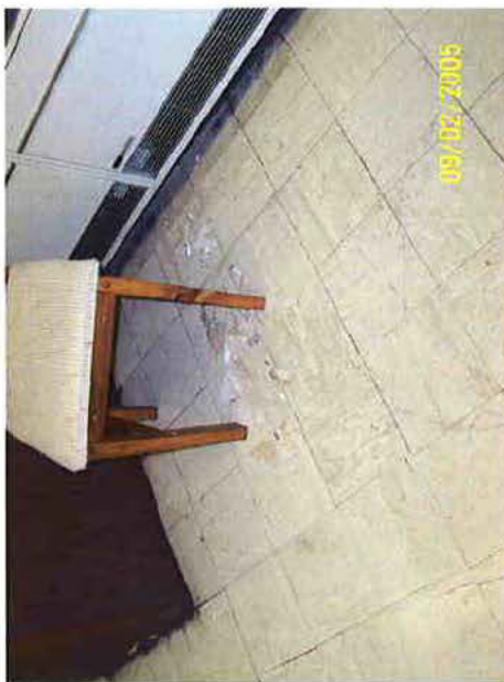
Photo 4: Day Room-Damaged ACM Floor Tile
