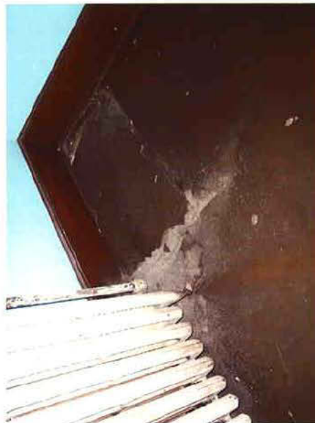
Photo 2: 3rd Floor Restroom-Damaged Plaster Ceiling
