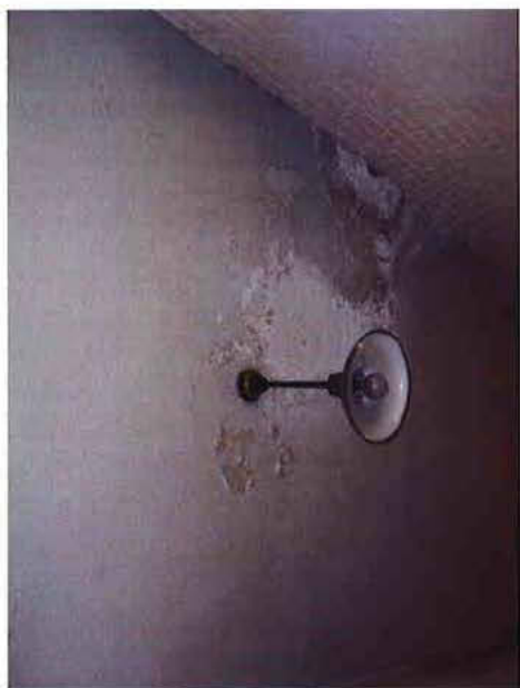
Photo 6: 3rd Floor Room 309B-Peeling Paint
