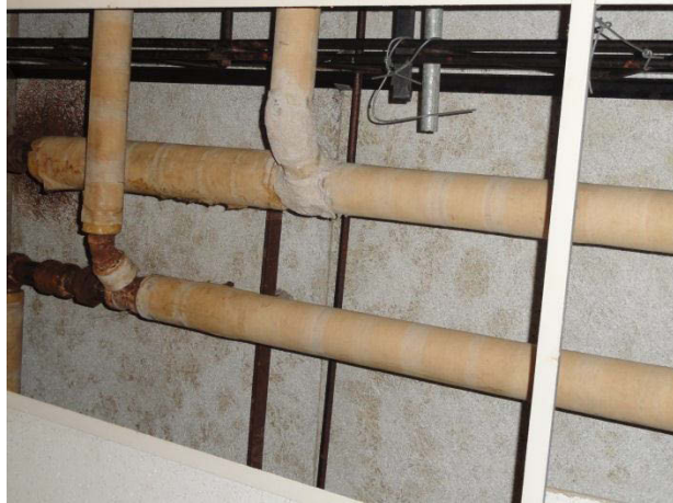
Hard Elbow Pipe Insulation
