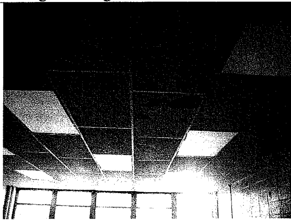
Photo 2: Conference Room – Water damaged ceiling tile
