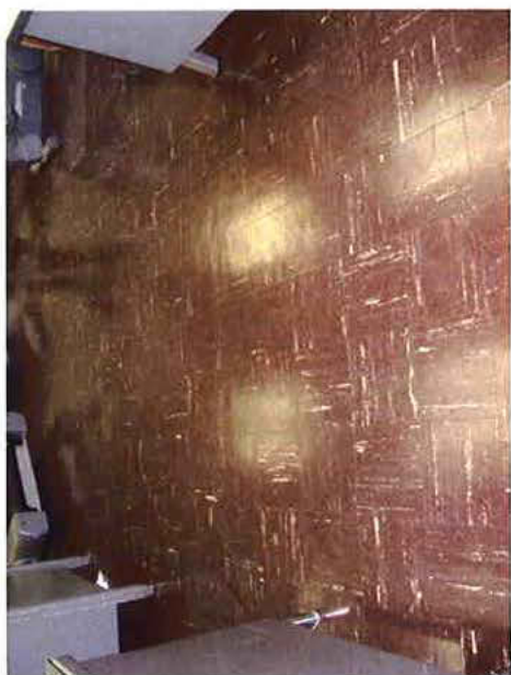
Photo 6: Platoon Room-ACM 9" x 9" Tiles in Good Condition
