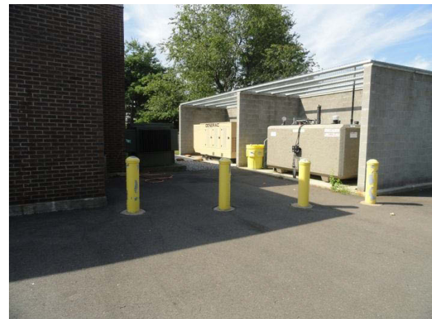
Generator and Fuel Tank
