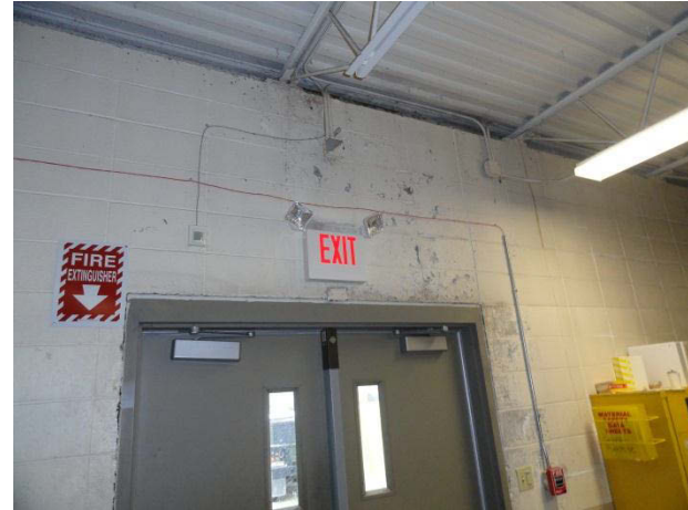
Supply Area Wall with Water Intrusion and Peeling Paint
