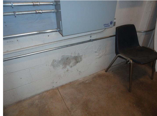
Peeling Paint in Boiler Room
