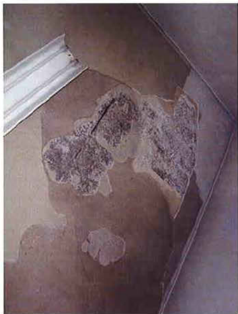
Photo 2: 3rd Floor Restroom-Damaged Plaster Ceiling
