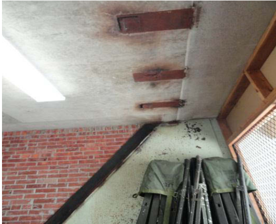
Remains of Bullet Trap on Ceiling
