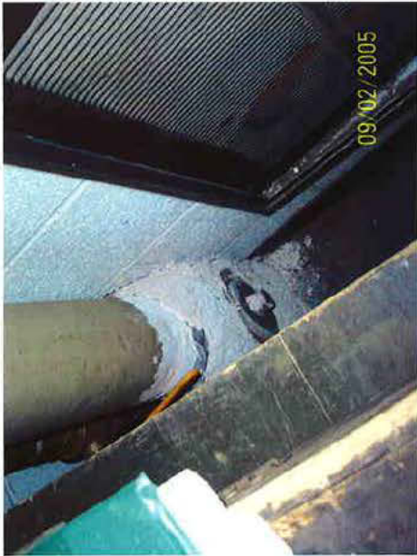
Photo 6: Former Firing Range-Damaged ACM Pipe Fitting
