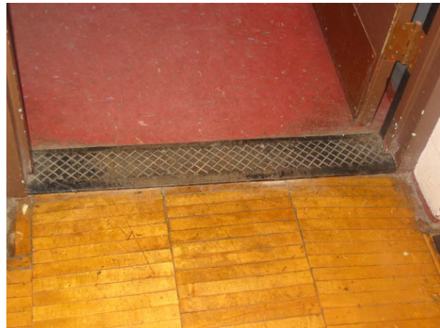
Photo 8: Day Room-Loose Threshold
