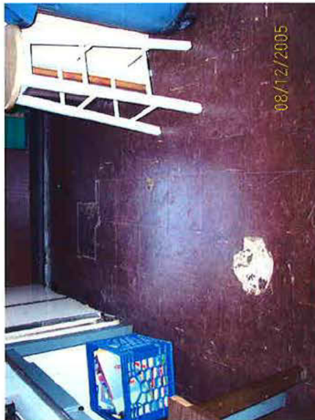
Photo 4: Day Room-Damaged 9"x9" Floor Tiles
