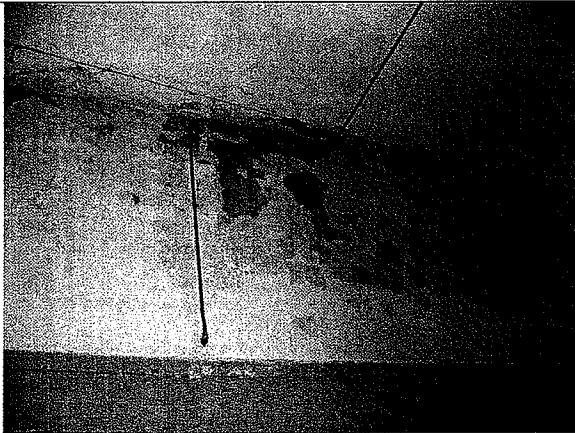
Photo 6883: Drill Hall – Stage with water damaged plaster and peeling paint (0825-25).
