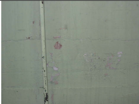
Photo 6858: Room 116 – Peeling lead-based paint
