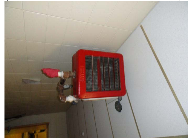
Stained Ceiling Tile and Rusty Pipes
