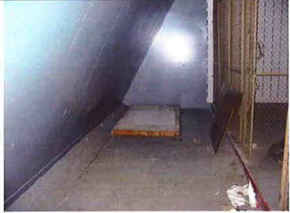
Photo 6983: Former Indoor Firing Range – Bullet Trap
