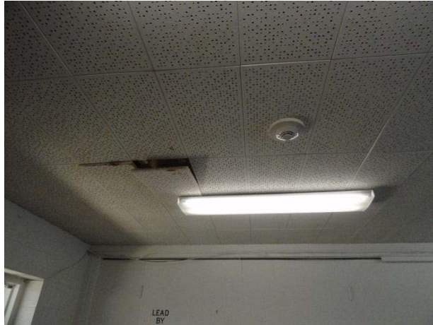
Spline ceiling tile coming unglued
