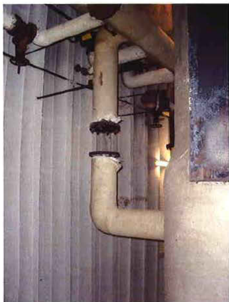
Photo 10: Boiler Room-Damaged Pipe Insulation
