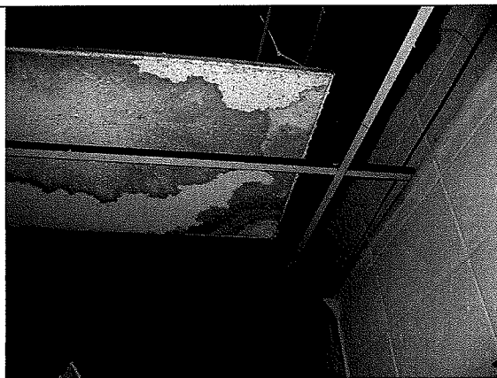
Photo 7106: Administrative Area – Water Damaged Ceiling Tiles
