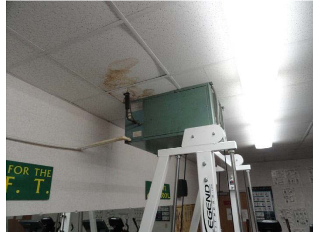
Stained Ceiling Tiles near Heater
