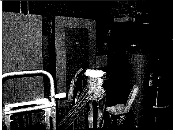
Photo 7098: Boiler Room – Obstructed Electrical Box
