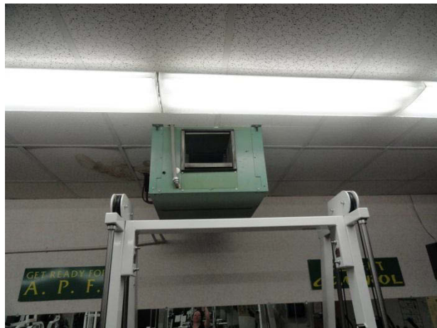
Stained Ceiling Tiles near Heater
