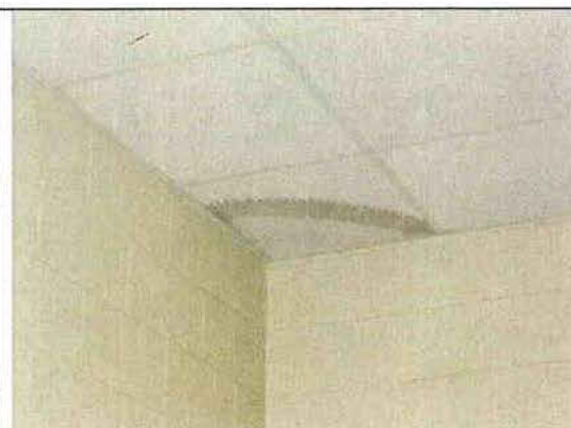
Photo 7034: Stairwell – Water damaged ceiling tile
