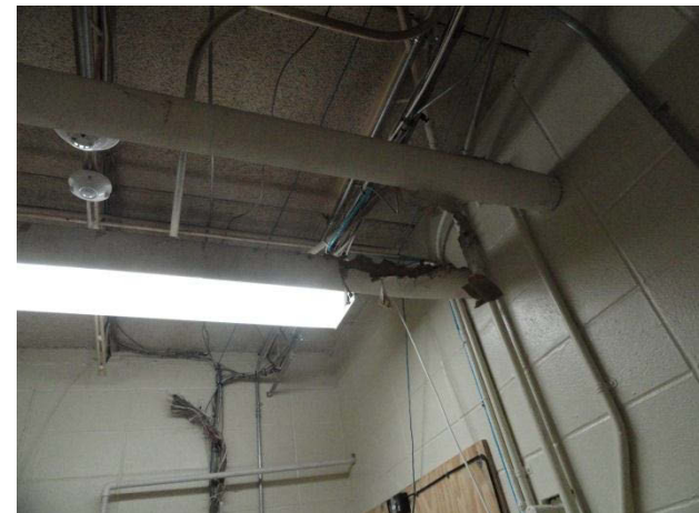
Damaged Pipe Wrap
