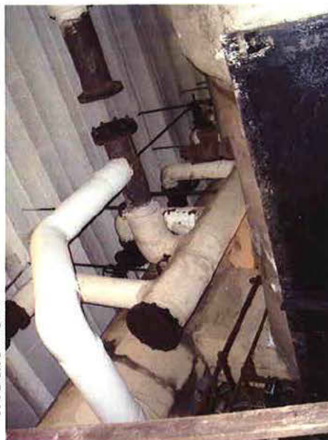
Photo 10: Boiler Room-Damaged Pipe Insulation
