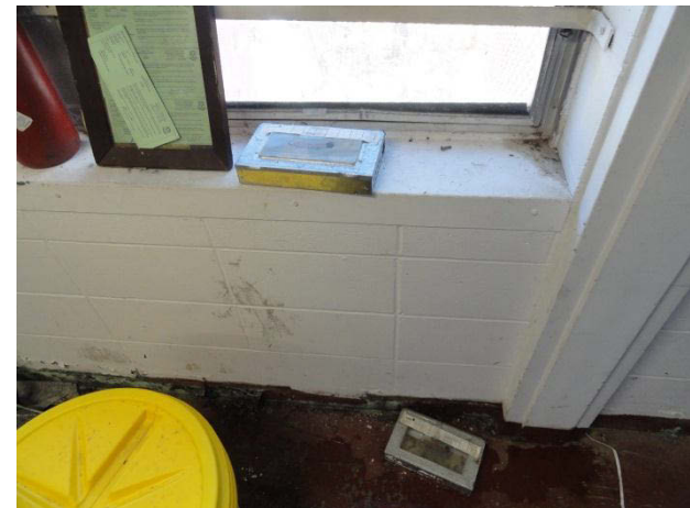
Water Intrusion on Floor
