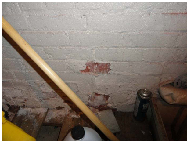
Peeling Paint and Moisture Problem in Custodian Closet #129
