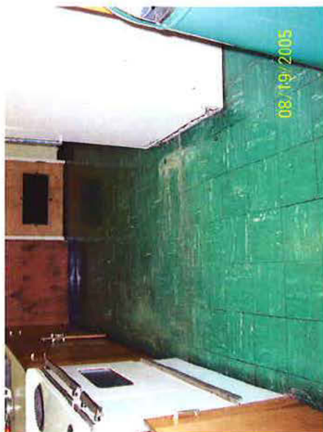
Photo 5: Kitchen-Suspect ACM Floor Tiles in Good Condition
