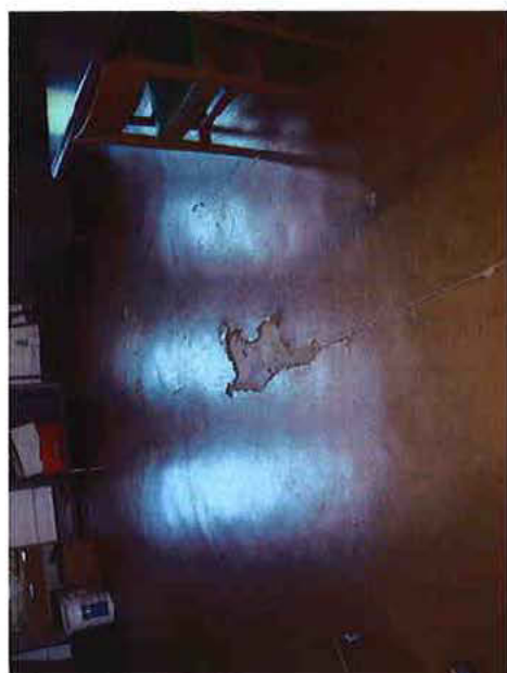
Photo 9: 2nd Floor Room 213-Damaged Suspect ACM Flooring
