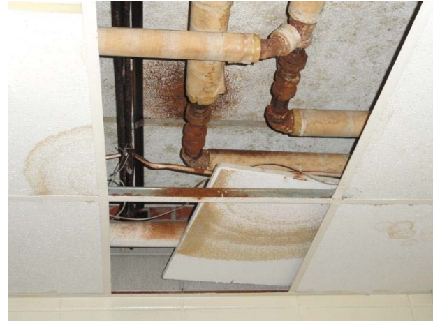
Stained Ceiling Tile and Rusty Pipes
