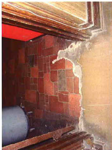
Photo 6: 3rd Floor Room 309B-Peeling Paint
