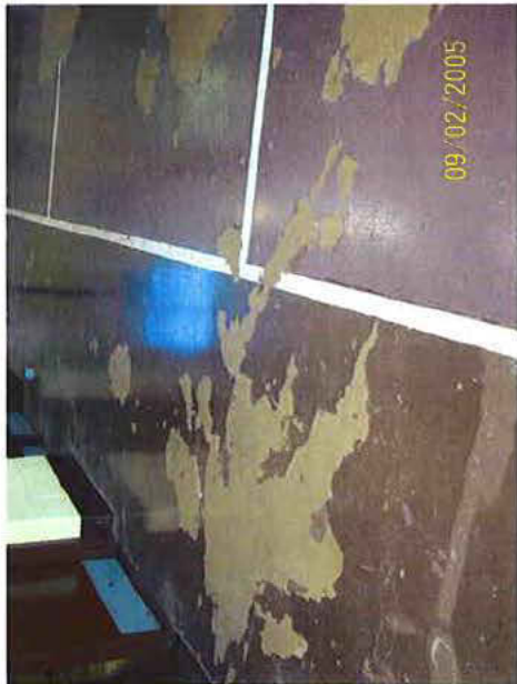
Photo 5: Drill Hall-Peeling Paint
