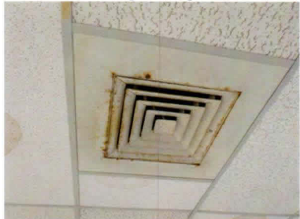
Damaged ceiling tiles
