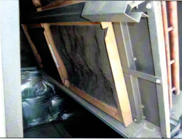
A/C =Heating Filter
