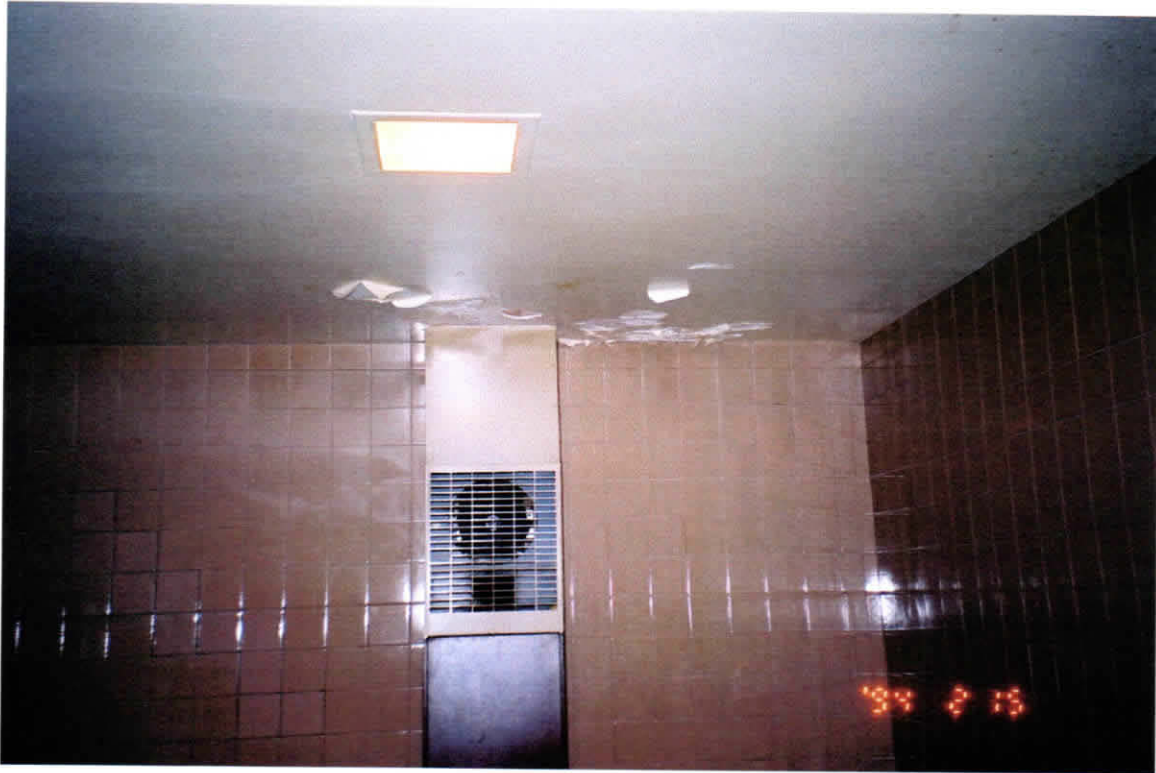
Views of paint blistering on the ceiling in the Men's latrine
