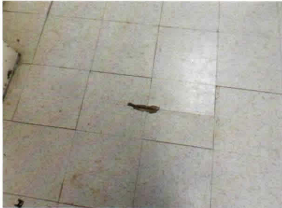
Damaged floor tiles/samples taken
