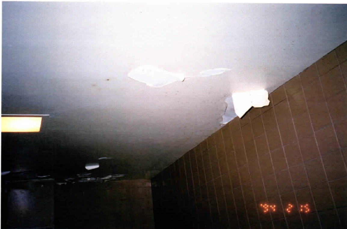
Views of paint blistering on the ceiling in the Men's latrine
