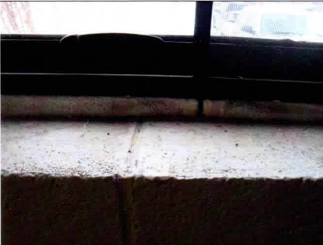
Towel Covering Air Leak At Bottom Of Window, OPS NCO Office (100B)
