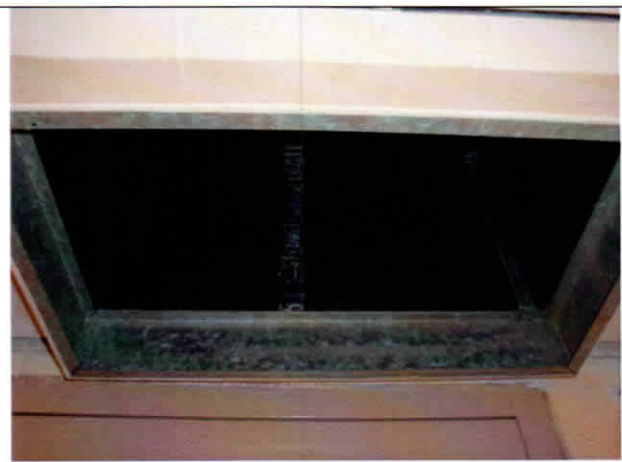
Missing A/C Filter, Next to SFC Combs/SSG Jones Office
