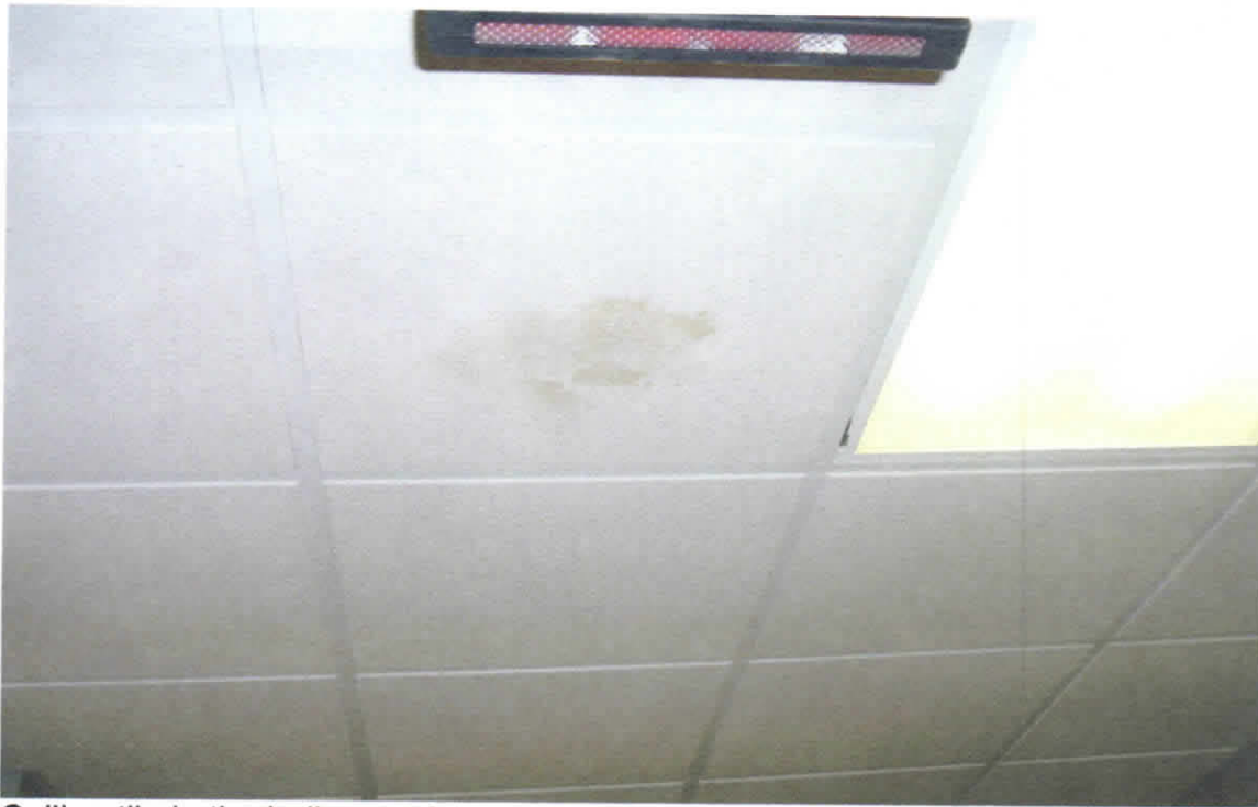
Ceiling tile in the hall way of the armory stained with water circles from leaks.
