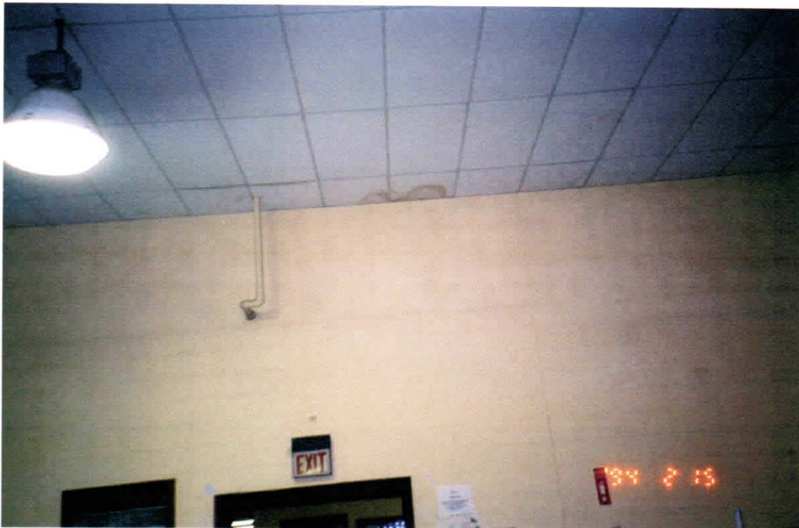
Views of water leakage from the roof in the Rodgers, Arkansas Drill Hall
