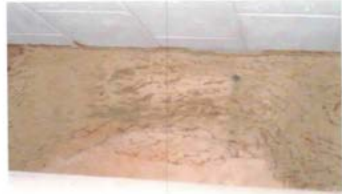
View of termite damage on the shelving in the supply room.
