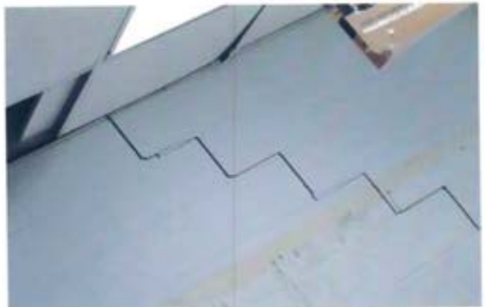
View of extensive structural damage of the interior wall of the Armory
