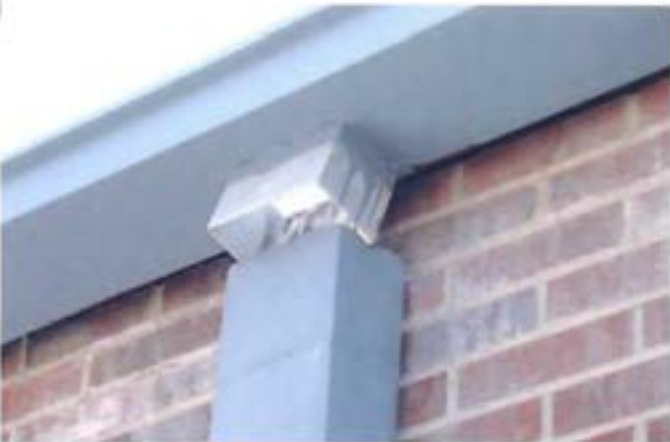
View of the gutter outlet that is dislodge from the downspout
