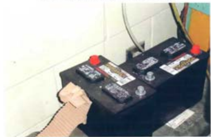
View of batteries improperly stored near an electrical outlet in the converted range
