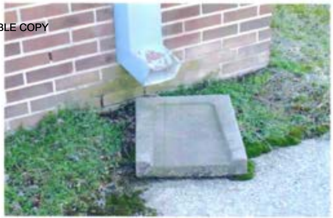
View of a dislodged splash block and water intrusion at the foundation
