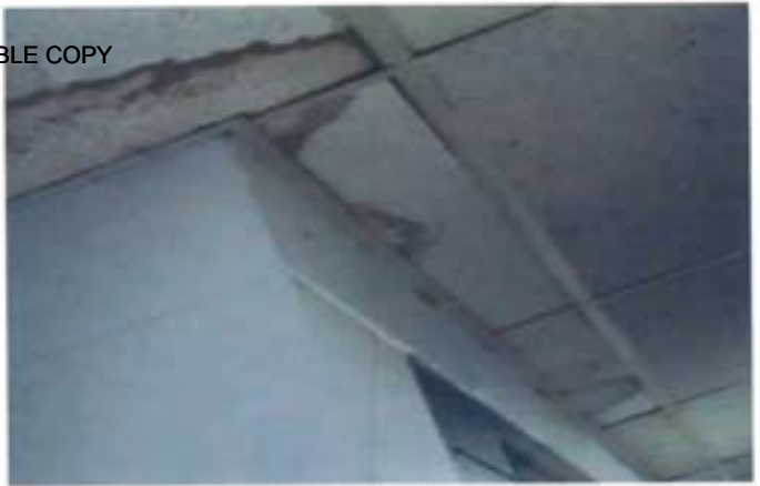
View of stained ceiling tiles in the hallway
