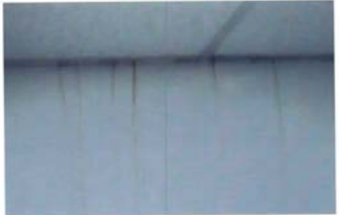
View of water stained walls that are present in several areas of the facility
