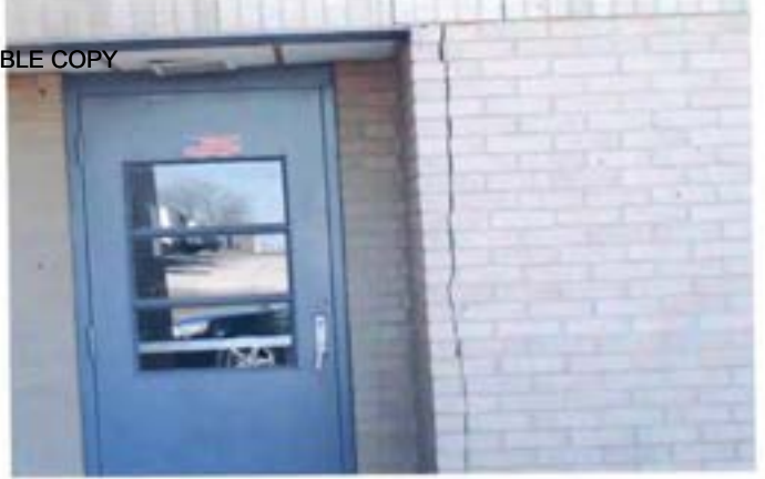
View of exterior damage on the brick of the Armory
