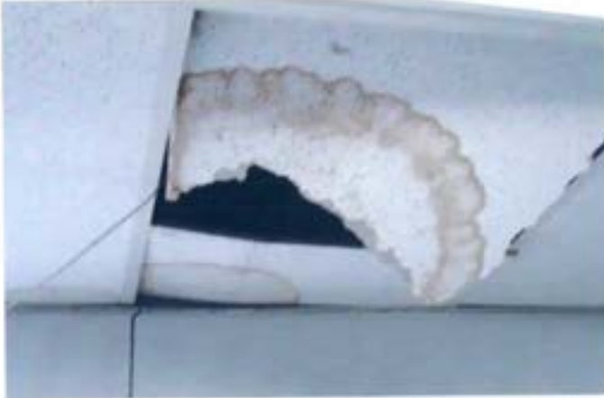
Example of stained water tiles that are present throughout the facility
