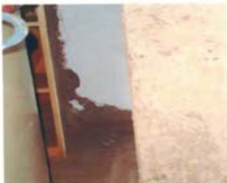
View of water and termite damage behind the shelving in the supply room
