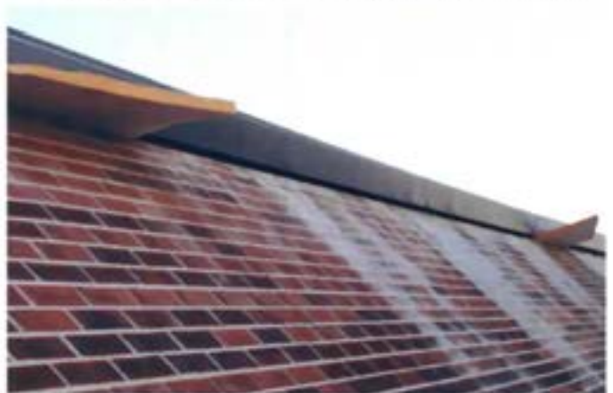
View of roof insulation that has dislodged from the roof
