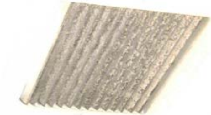
Example of soiled air grills that are typical in this facility
