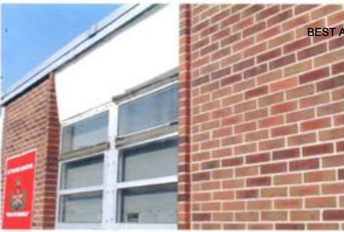
View of water damage around windows. (Wood header is swelling)
