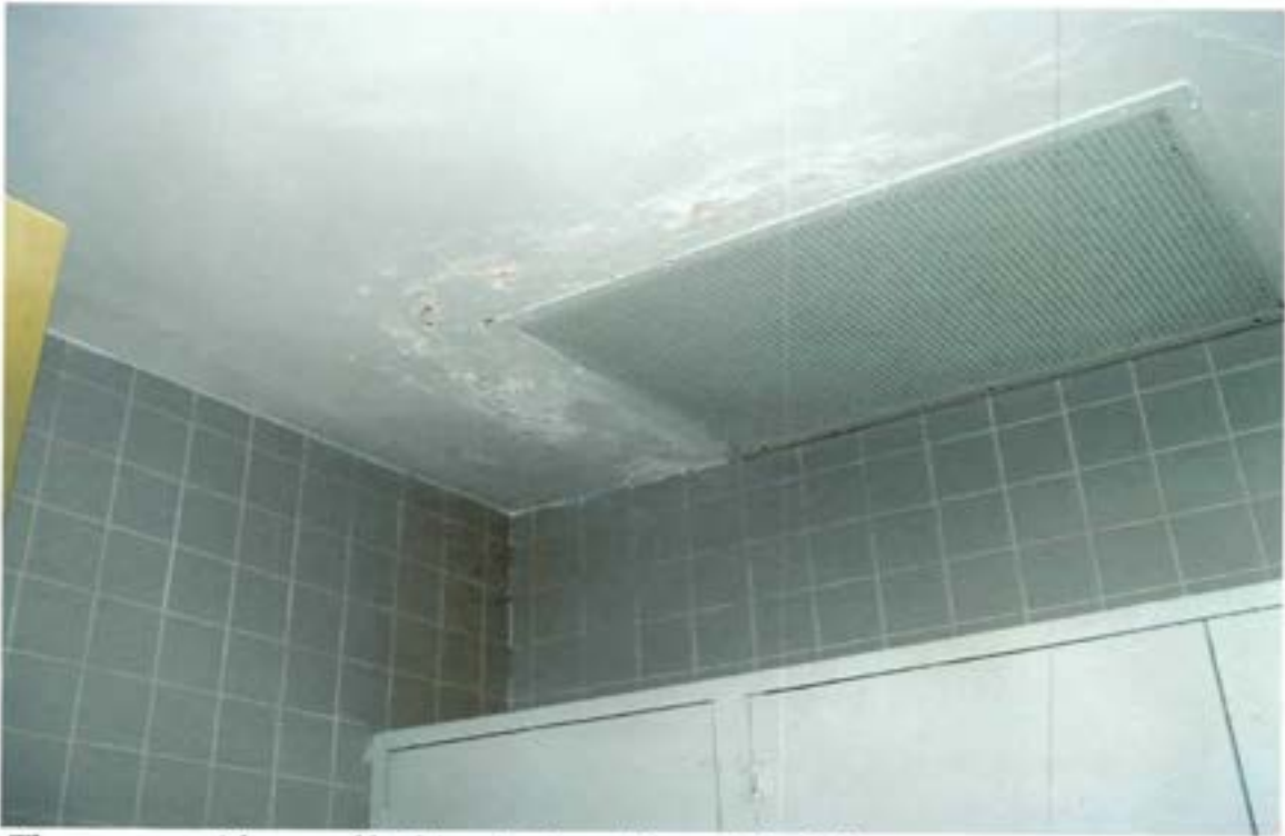
There was evidence of leaking in the ceiling of the kitchen
