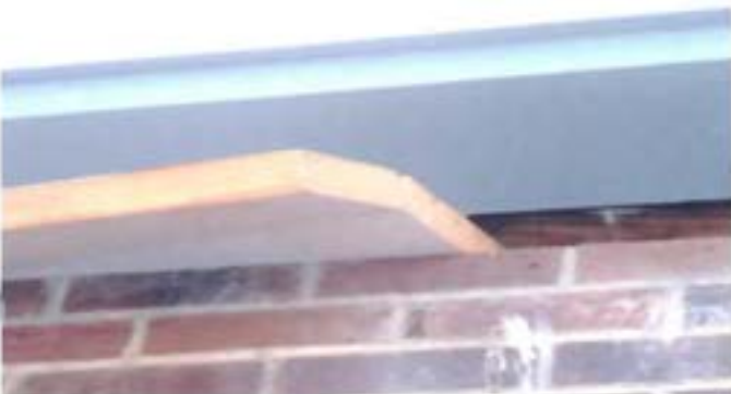
View of roof insulation that has dislodged from the roof
