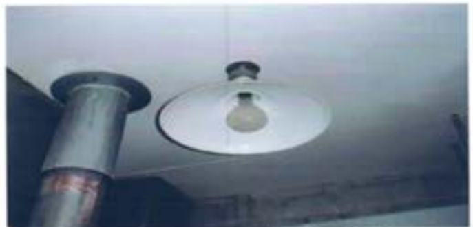
View of the non-explosion proof lighting in the AHU room
