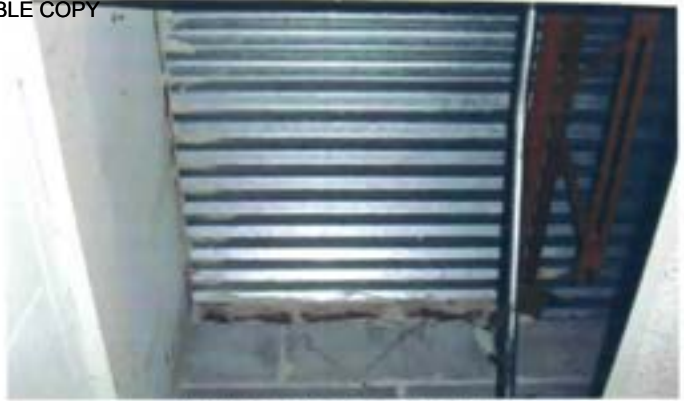
View rusting on the metal roofing material above the drop ceiling in the office of the commander
