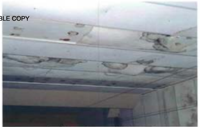
View of the water damage and mold growth on the ceilings within the deactivated indoor firing range
