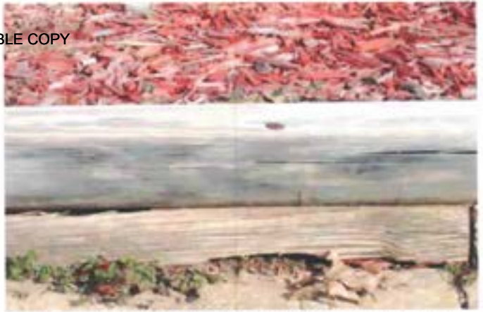
View of possible termite damage on landscape timbers located in the front of the Armory
