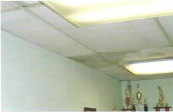
View of the stained ceiling tiles in the commander's office
