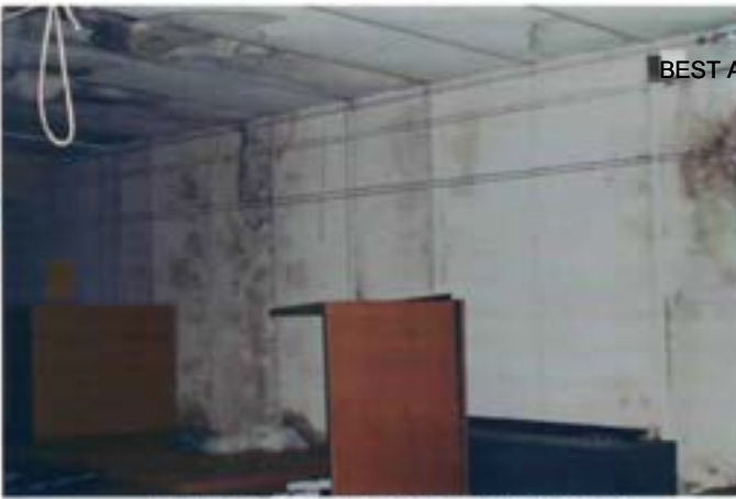
View of the water damage and mold growth on the walls and ceilings within the deactivated indoor firing range
