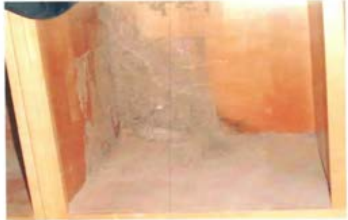
View of termite damage on the shelving in the supply room.
