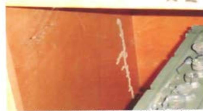
View of termite mud tunnels, located within the wooden shelving in the supply room
