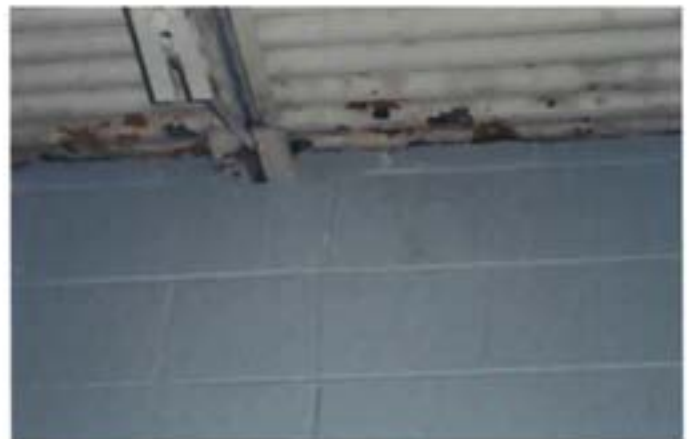
View of the rusting roof structure in room 116
