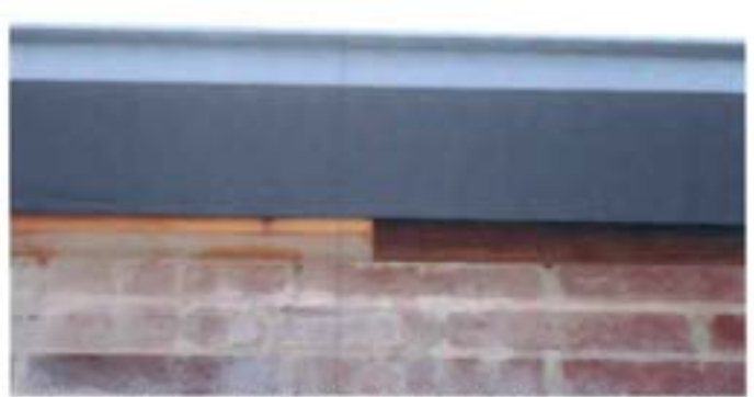
View of missing metal sheathing at the roof header, exposing wood
