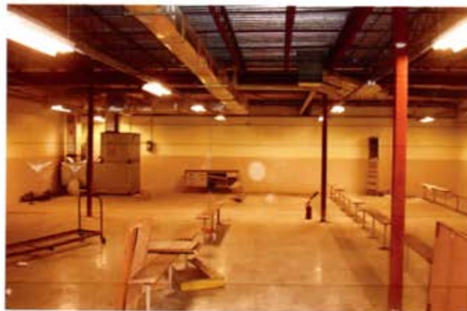
View of former locker room within the Armory
