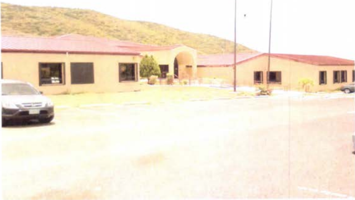
Photo #1: Front entrance of the VIARNG Armory Building.
