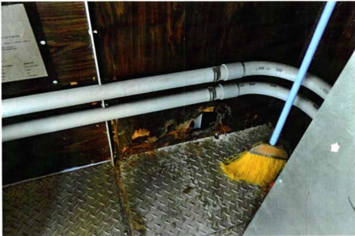
#16 – GUARD SHACK INTERIOR
