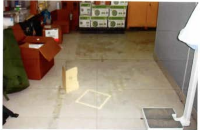
View of Lead wipe sample 4, located on the floor in the Medical Det supply room
