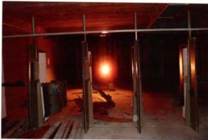
View of the Indoor Firing range (downrange view)
