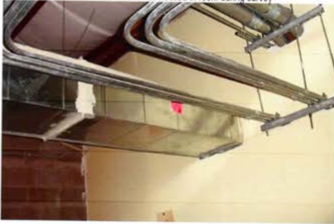
View of duct leading into the indoor firing range
