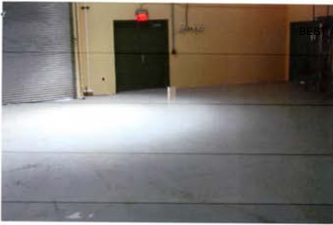
View of Lead wipe sample 5, located on the Drill Hall Floor
