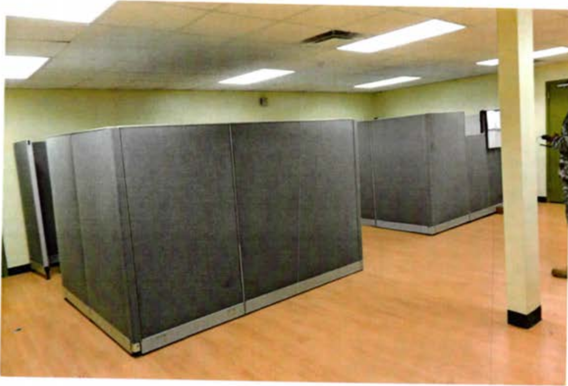
#7 – TYPICAL REMODELED OFFICE AREA
