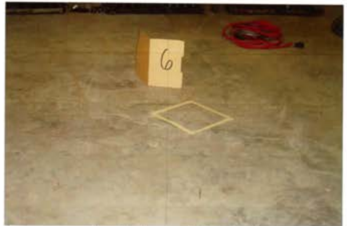
View of Lead wipe sample 6, located on the floor in the Medical Det between cubicle and shelf
