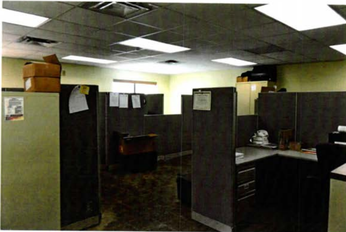
#8 – OFFICE AREA AWAITING FLOORING
