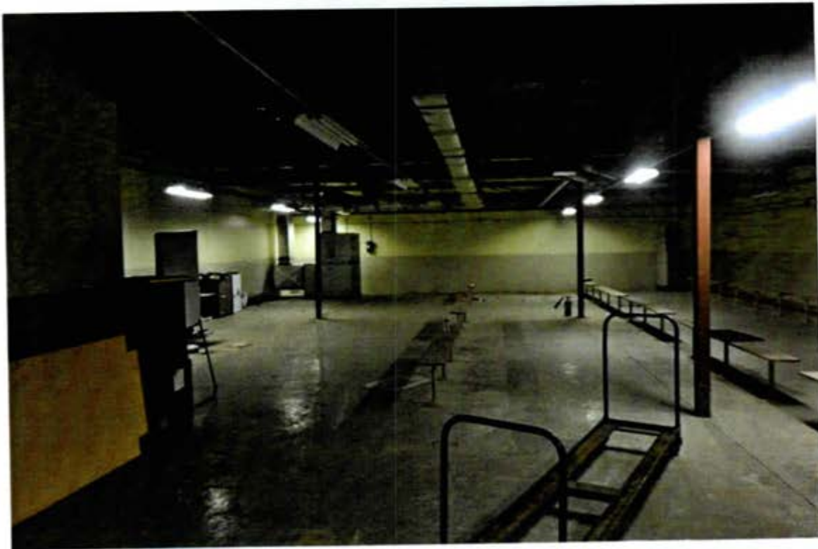
#14 – MEN'S LOCKER ROOM
