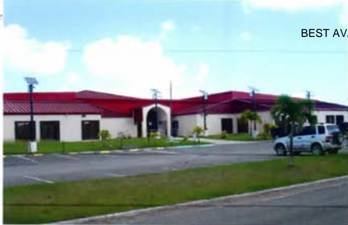
View of the ST Croix USVI Armory
