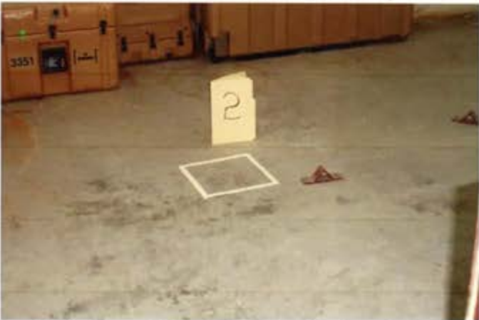
View of Lead wipe sample 2, located on the floor of vault of Troop Command supply room
