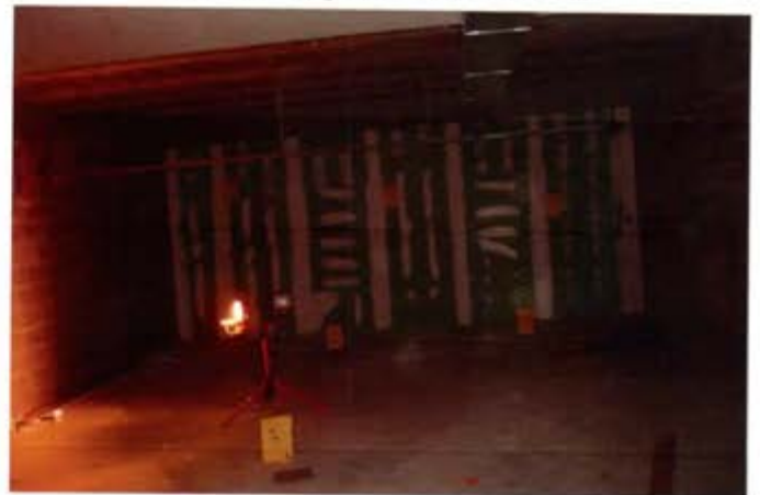
View of encapsulated wall (drywall), former area of backstop
