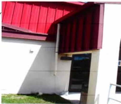
View of downspout from the gutter
