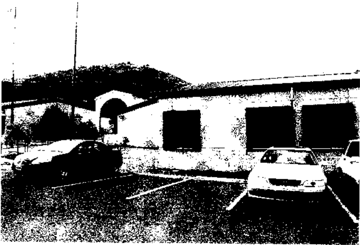
Photo #1: Front entrance of the VIARNG Armory Building.
