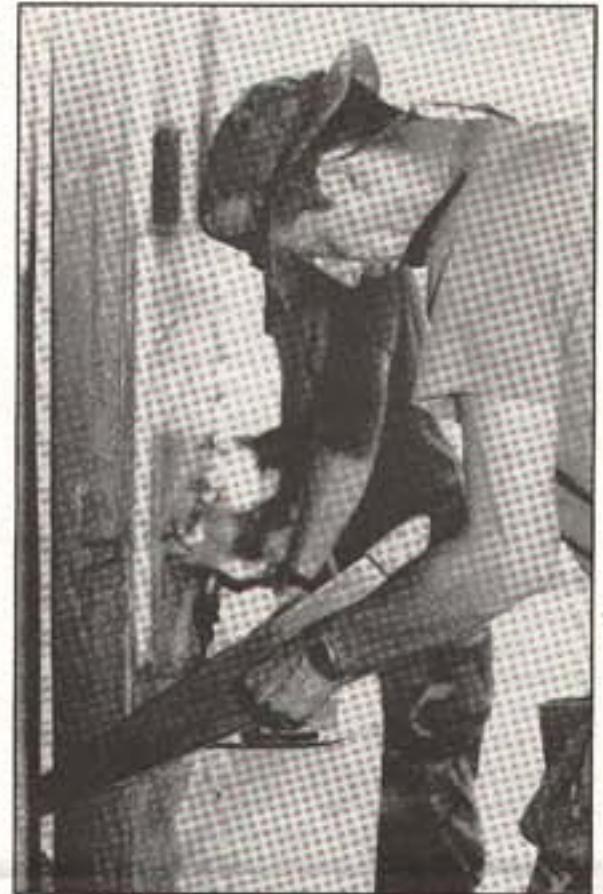
NEW CUT - Sgt. Charles Goza, a carpenter with the 875th Combat Engineers, Arkansas Army National Guard, removes a damaged door jamb at the school in Pese, Panama. (Photo by Staff Sgt. Mike Dorcey, Kansas Army National Guard).
