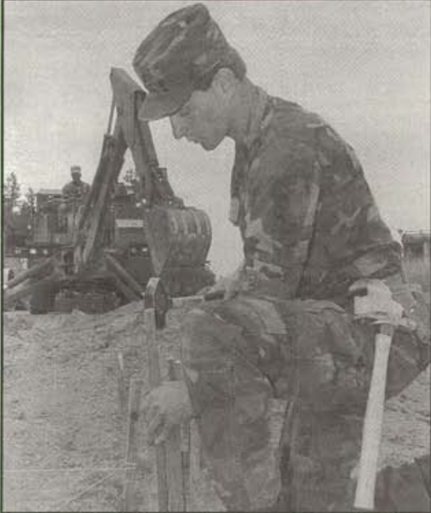
Even though the batterboard that Oregon National Guard Spc. David Dowell is constructing is designed for precise layout of concrete forms, in reality he is several hundred miles off target. In fact, he's out of Oregon entirely. He and other members of the 442nd Engineer Detachment traded annual training sites with the Wyoming Army Guard's 1041st Engineer Detachment. In the background, Spc. Peter Davis digs a trench for the same Camp Guernsey project in eastern Wyoming.
