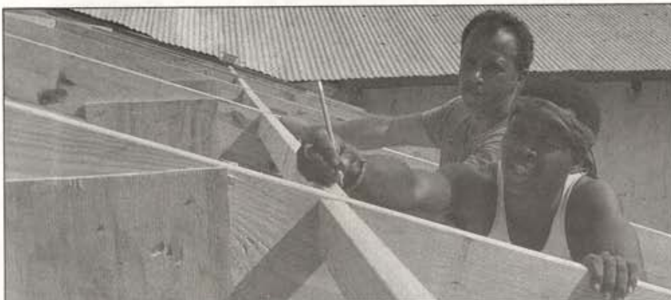
PENCILING - Staff Sgt. Pat Hayek, a power production technician, 133rd Civil Engineering Squadron, Minnesota Air National Guard, lends a hand as 22-year-old Carmelo Rodriguez marks roof rafters on a school. The Air Guard squadron spent their two week annual training restoring the schoolhouse, with volunteer help from many of the villagers. (Photo by SPC. Bill Kelley, 110th Public Affairs Detachment).
