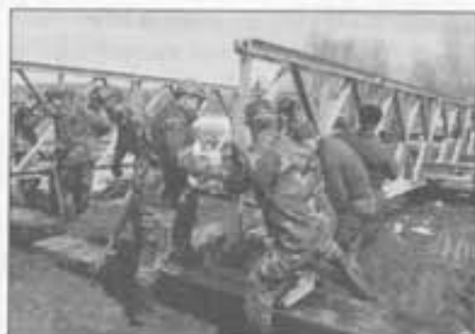
SPANNING THE GAP - Engineers constructed a Bailey Bridge to carry traffic while an earthen dam is being rebuilt for environmental purposes.
