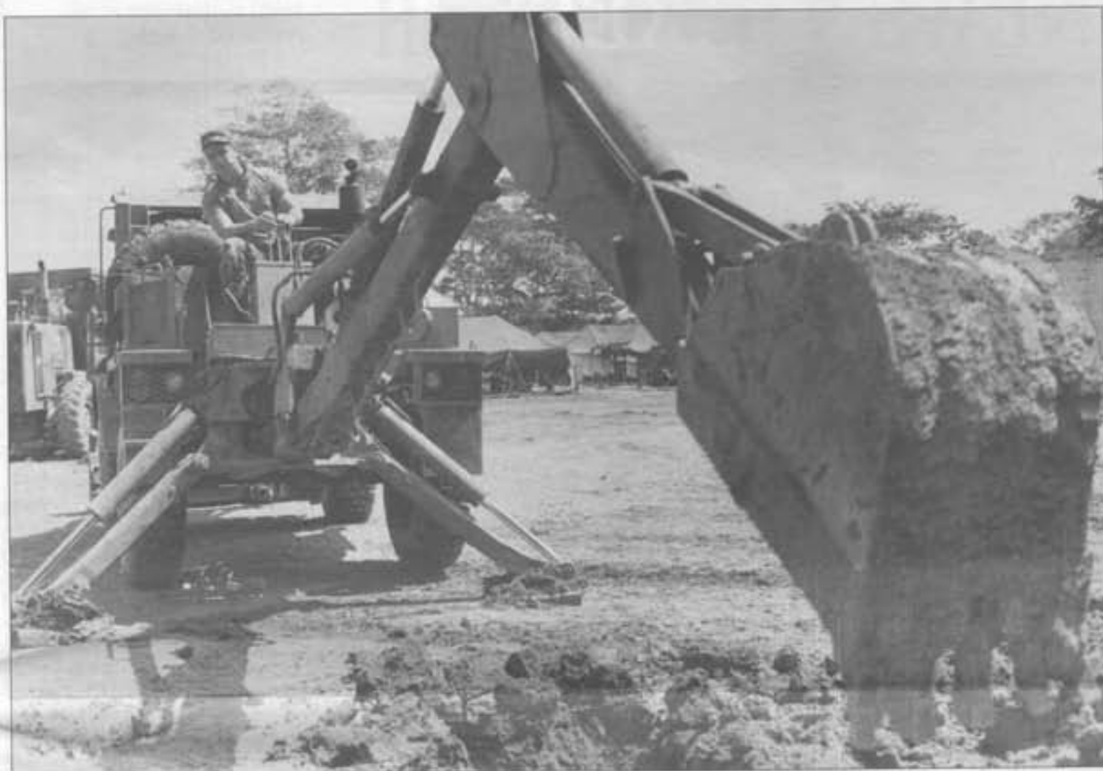
DITCH DIGGING- Spc. Scott D. Yonker, with the Missouri Army Guard's 204rd Engineer Battalion, operates a Small Emplacement Excavator to dig a drainage ditch in Puerto Jimenez, Costa Rica. Yonker is a student at Missouri Southern State College.
