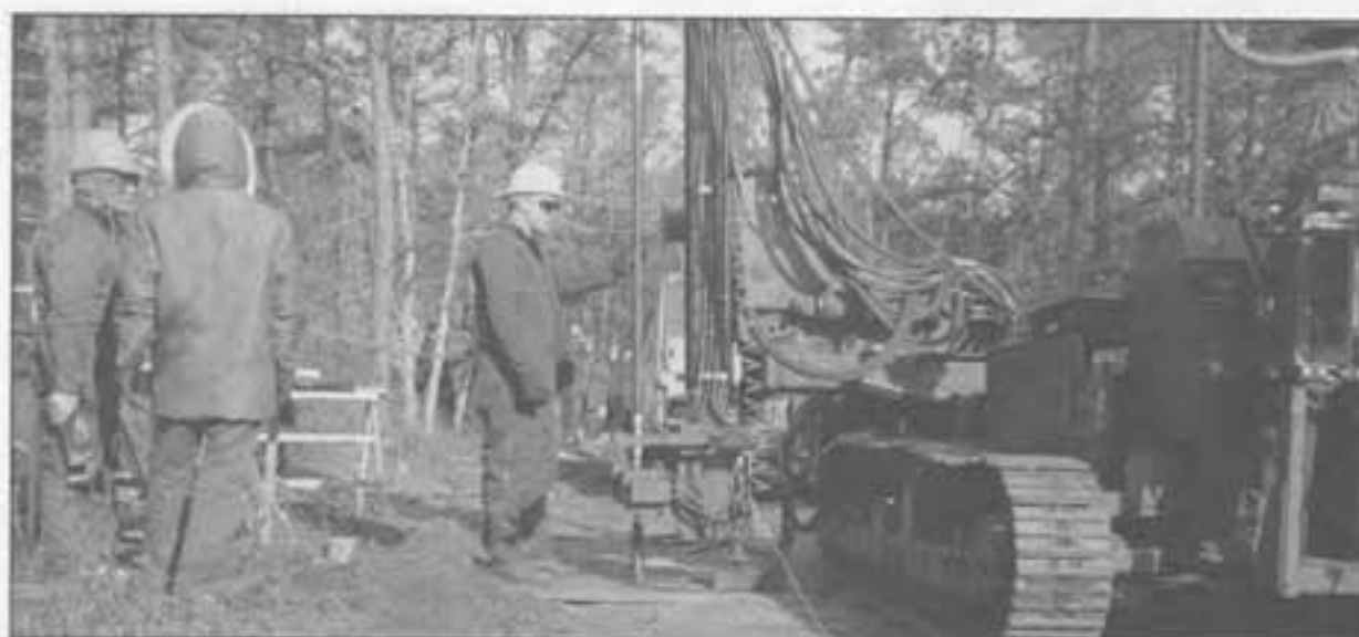
WELL MONITOR - A drill rig is used to install a ground water monitoring well at the Massachusetts Military Reservation.
