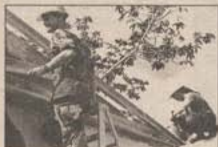
ON TOP OF THINGS - Michigan Army Guard engineers align a roof beam on a schoolhouse.
