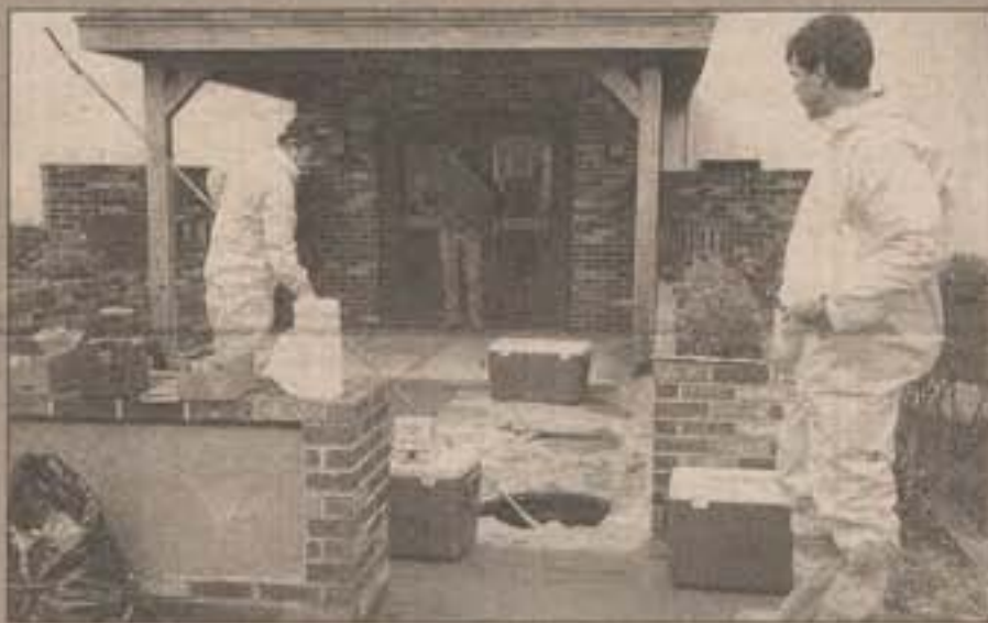
DIGGING FOR CLUES - Field technicians (left) obtain a sample from a drainage structure. Those identified as contaminated will be pumped out. One environmental compliance expert looks at how units store hazardous materials (above). This, they say, is a safe way to prevent potentially harmful chemicals from interacting and causing unnecessary damage.
